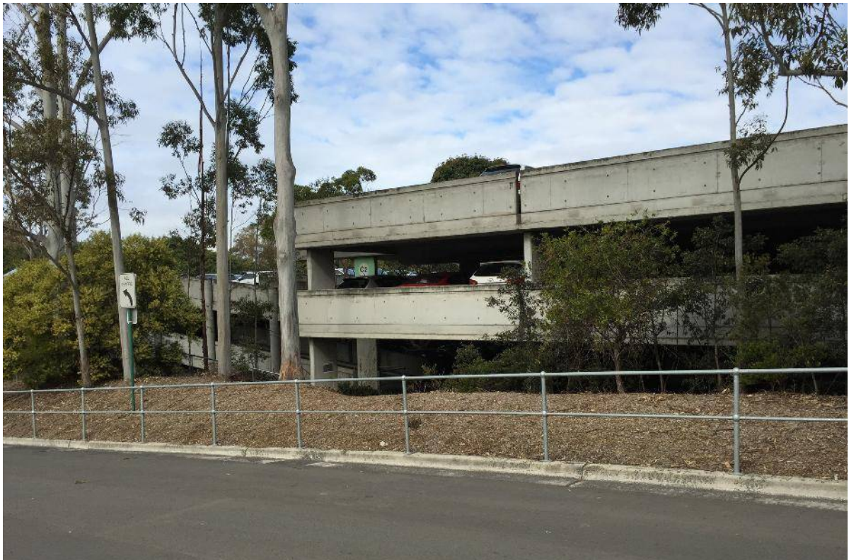
Figure 3.10, Existing multi-deck carpark on lot E3.
