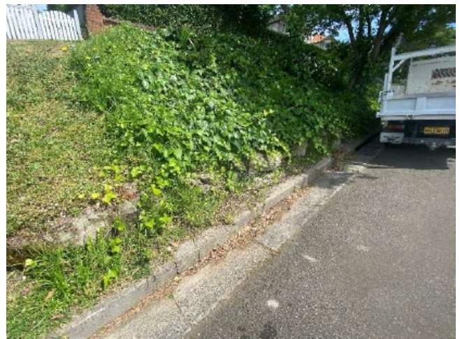
Picture 8 Vegetated retaining wall on Redan Street
