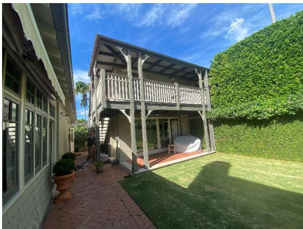
Figure 34 Ancillary structure located to the rear of the house.
