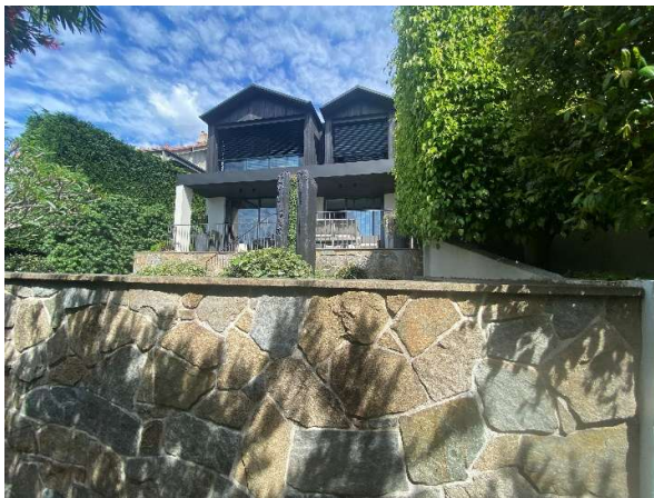
Figure 38 Primary façade of 46 Redan Street.
