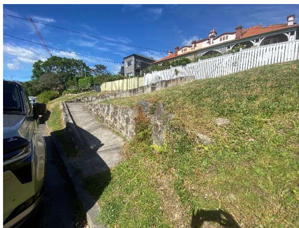
Figure 9 Retaining wall, concrete path cut through it.
