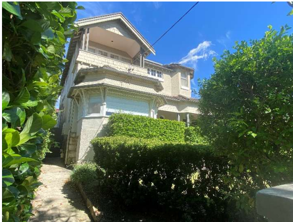
Figure 24 Southern corner of the primary elevation.
