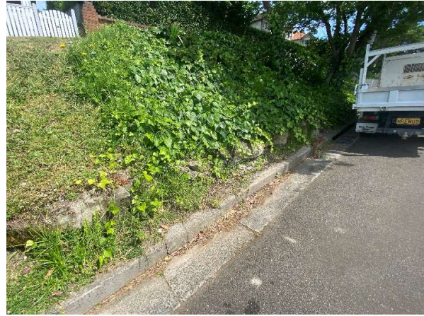
Figure 4 Section of the vegetated retaining wall on Redan Street.
