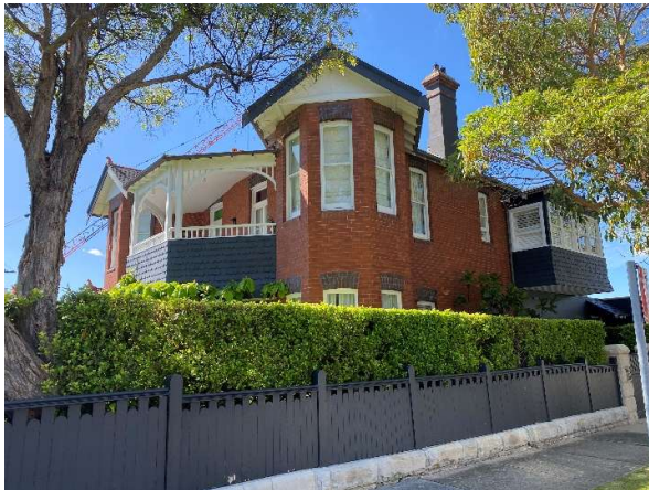
Figure 13 Heritage item at 29 Redan Street (Redan Street elevation).
