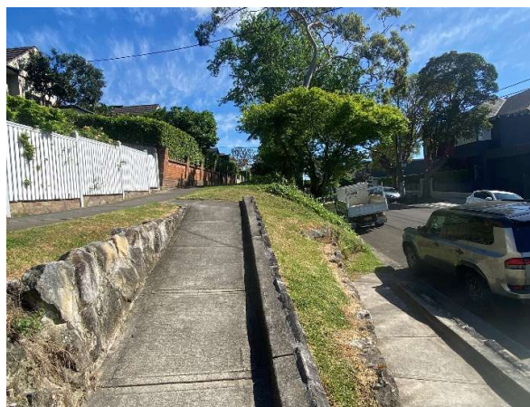
Figure 10 Retaining wall, with the Divided Road to the right.
