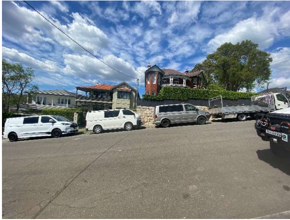
Figure 15 29 Redan Street as viewed from the north side of Balmoral Avenue.
