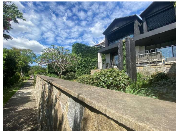
Figure 39 Primary façade showing stonework detail of the podium.
