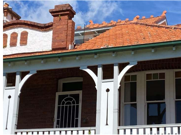
Figure 12 Detail of the roof of 38 Redan Street.
