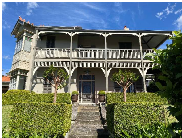
Figure 28 Primary façade of 44 Redan Street.
