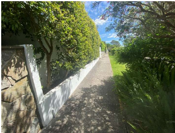
Figure 40 Concrete fence with built in garden bed of 48 Redan Street.
