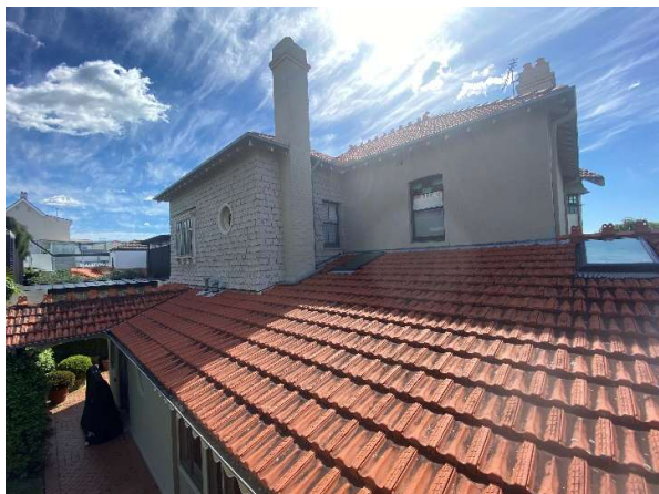
Figure 35 View across the roof, showing orange terracotta tiles.
