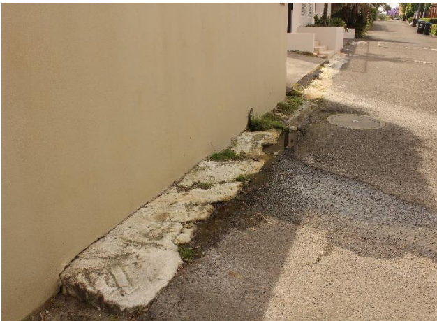
Figure 23 – View northwest of remnant sandstone along Redan Lane.
