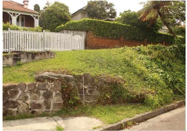
Figure 27 – View northwest of continuing slope along Redan Street along the southeast corner of the subject area.
