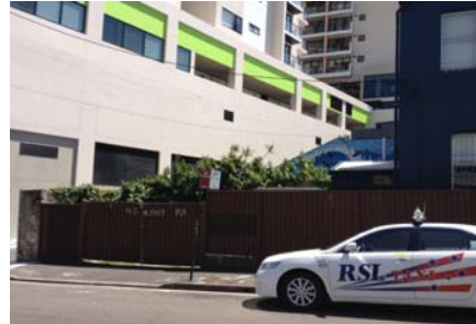
View of metal gate on southern boundary of site Looking north Inspected on 20.11.2015
