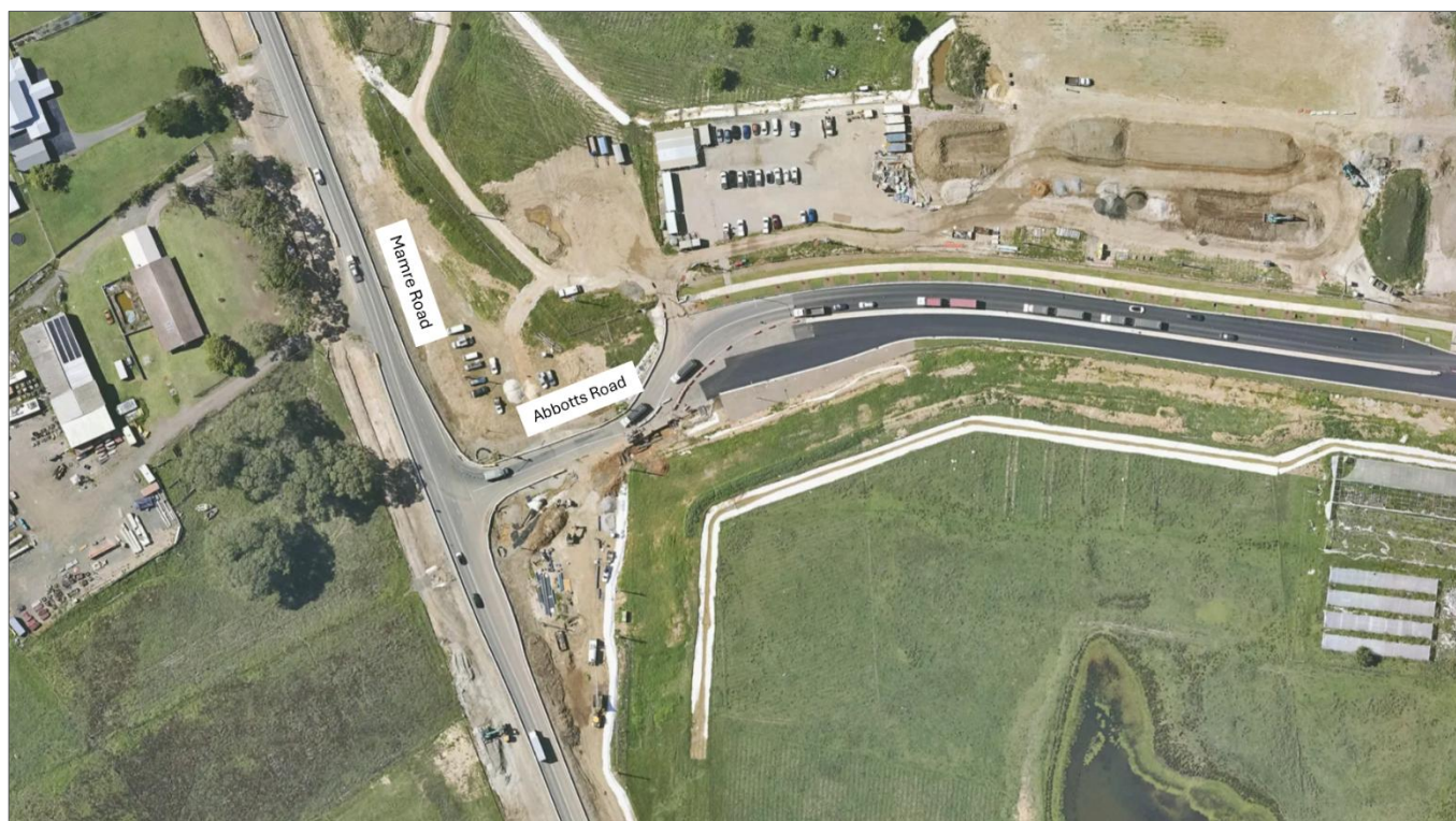
Figure 21: Existing Mamre Road / Abbotts Road Intersection
