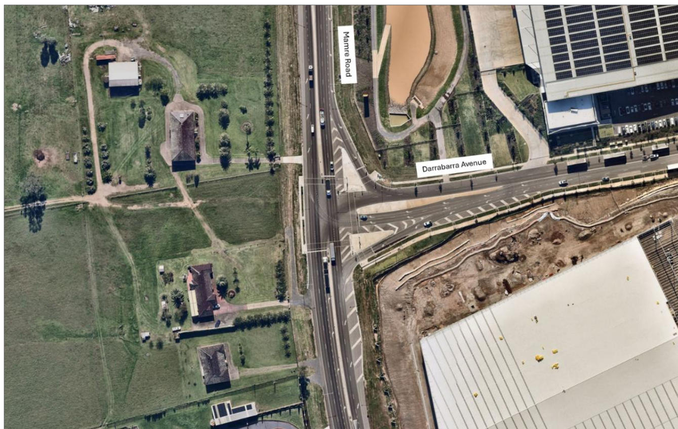
Figure 20: Existing Mamre Road / Darrabarra Avenue Intersection
