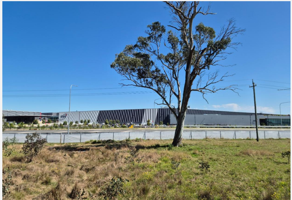
Photo 3 PCT 3320 in low condition within the subject land
