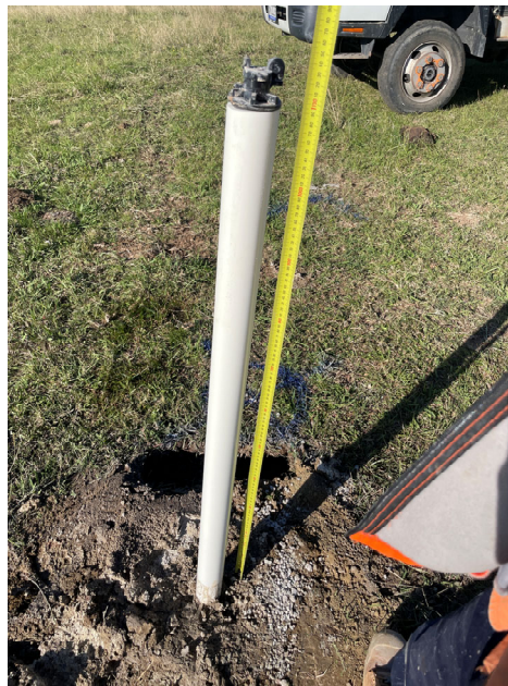
Photo 6 - Ground monitoring well stick-up
