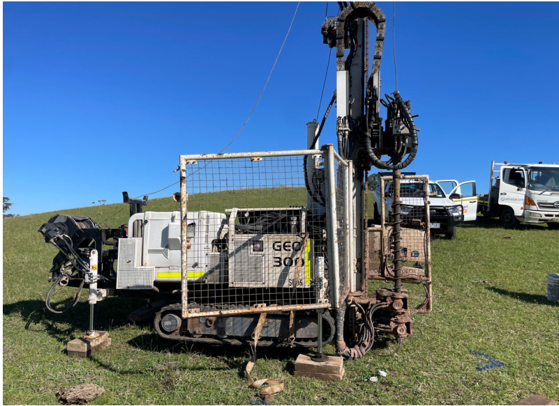
Photo 3 - Track mount drill rig (Comacchio Geo 300)
