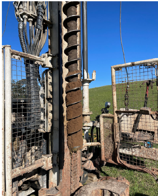
Photo 4 - Soil material from auger drilling
