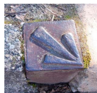
Alignment Pin references road alignment
