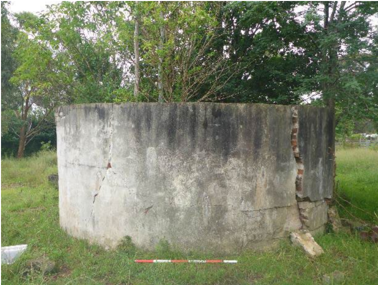
Photo 22 Brick water tank, facing north-east
