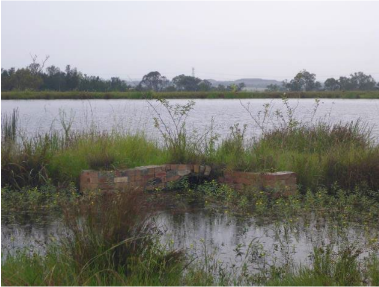
Photo 12 Brick culvert and dam [14], facing south-west
