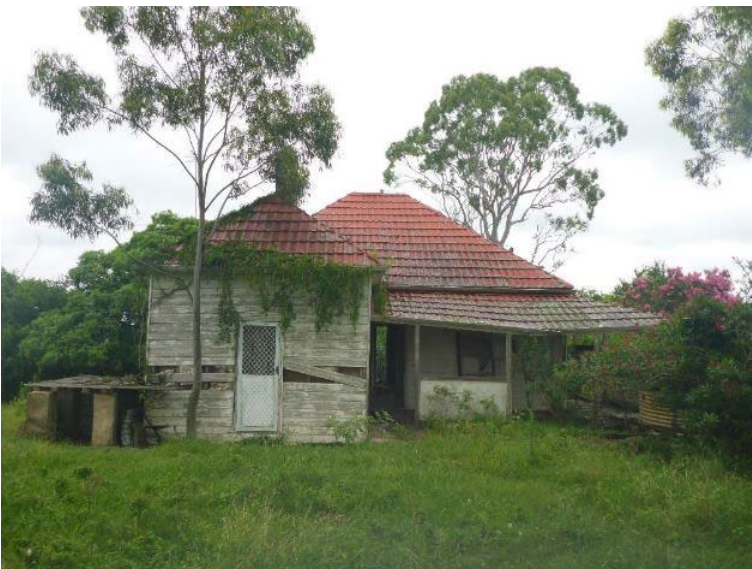
Photo 13 Residential building [2], facing west
