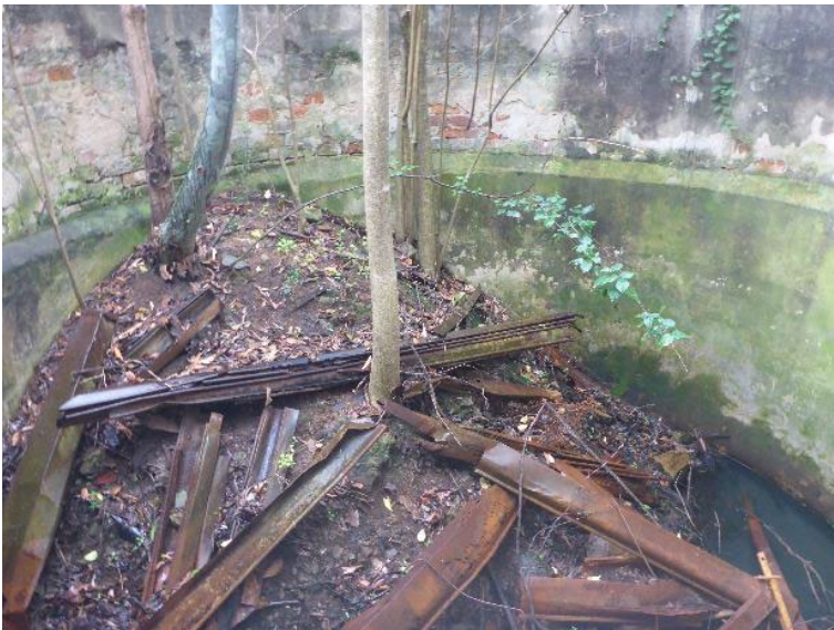
Photo 23 Internal view of brick water tank
