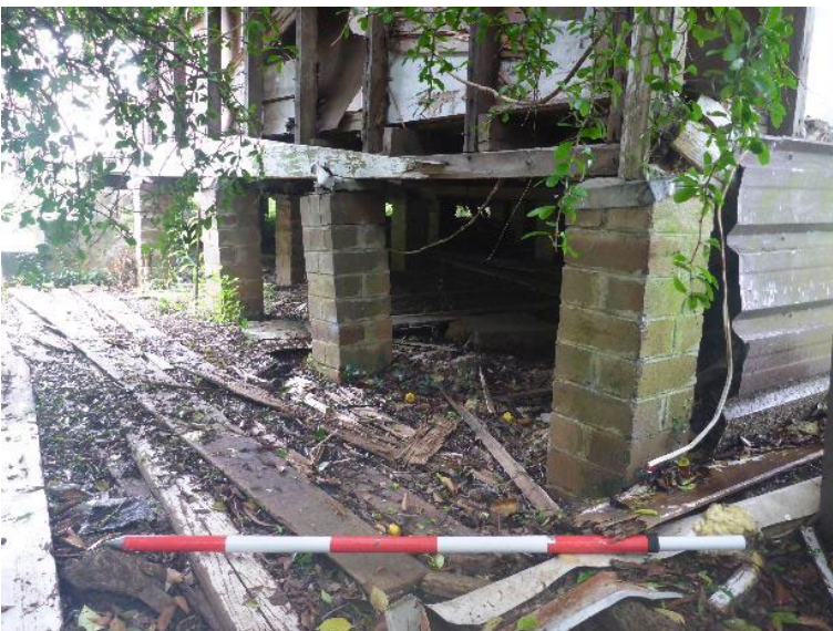
Photo 16 Brick piers under residential building [2], facing north-east
