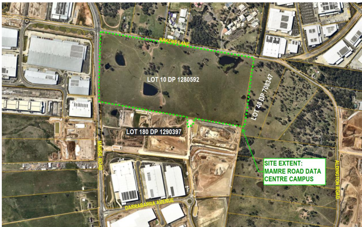
Figure 1: Site Area (imagery source: nearmap, 10 October 2025)
