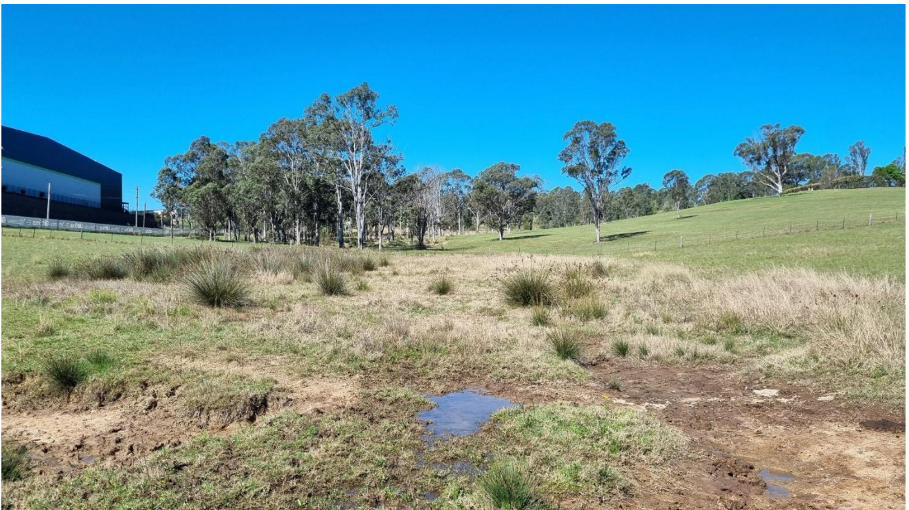
Photo 12 Pooling near Dam 8 along Overland flow 4
