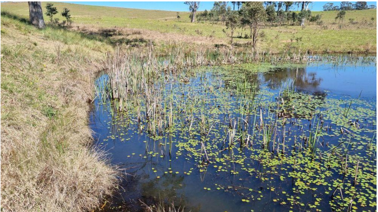
Photo 6 Water flowing from Dam 8 into Dam 7 with an eroded back edge of Dam 8 creating a bank
