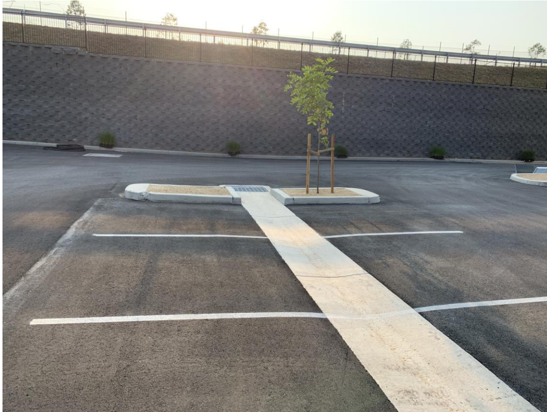
Figure 8: Example of retaining wall in location of cut
