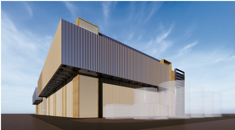
CORNER NORTH- EAST FACADE
