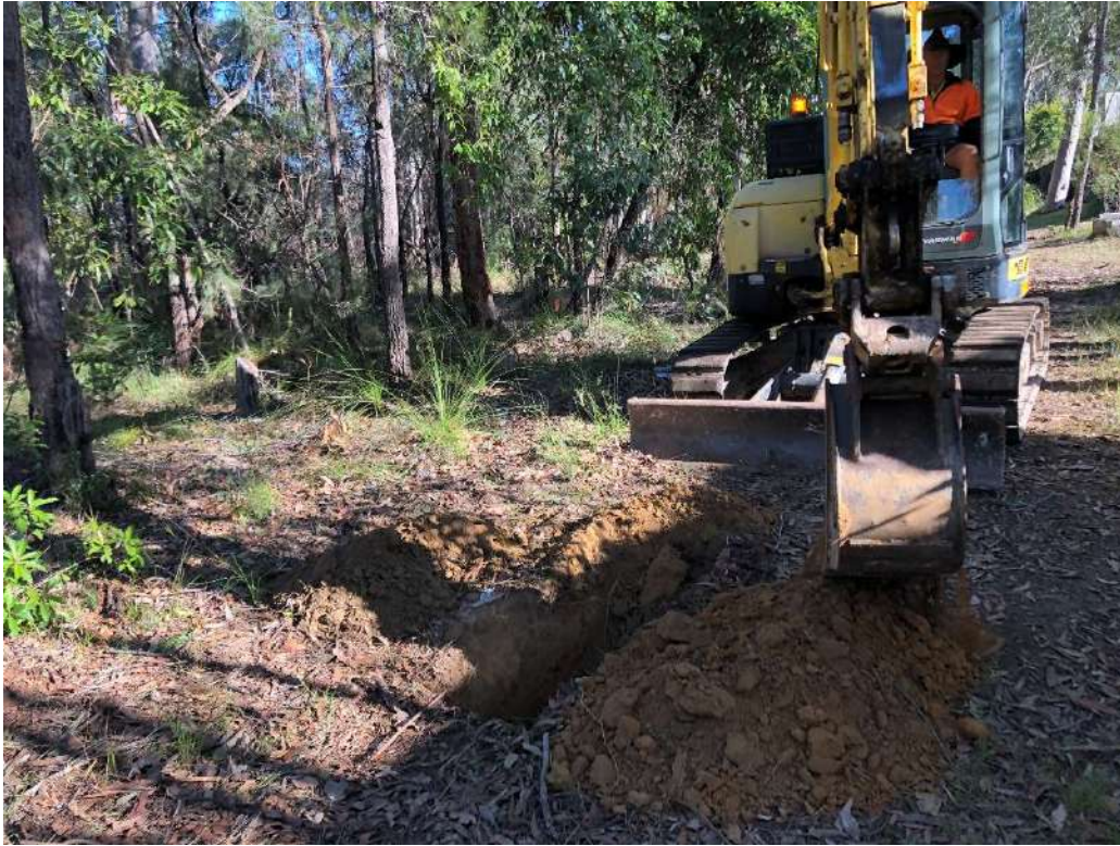
Photo 1. Test pitting at the southern vegetated portion of the site
