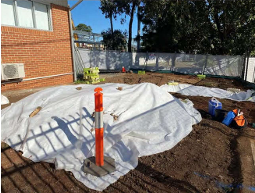
Photo 1. Example of stockpile covered with geofabric layer (STP06)
