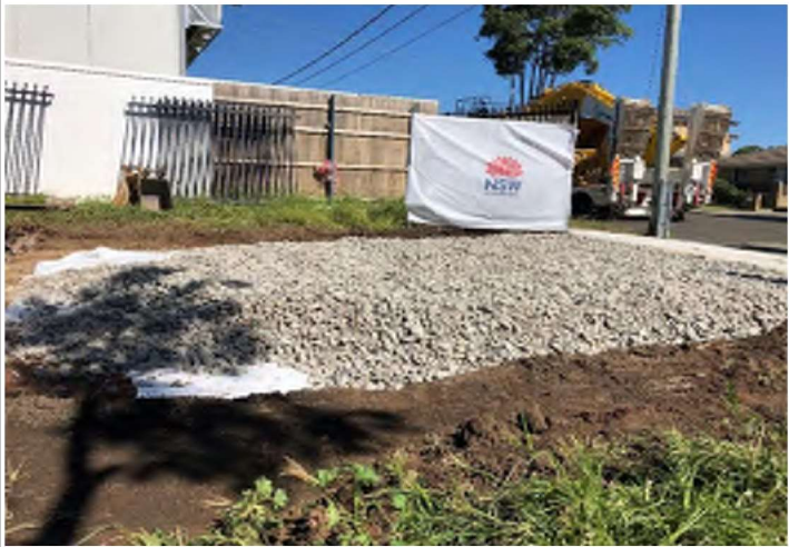
Photo 11: Entrance and exit gate covered with geofabric layer and imported certified material
