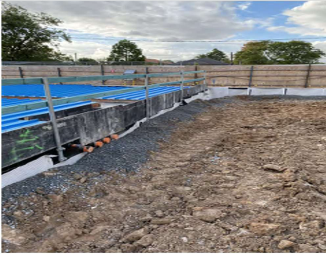
Photo 21: WSP inspection dated on 15/05/2020 - placement and pinning of geotextile material around OSD wall
