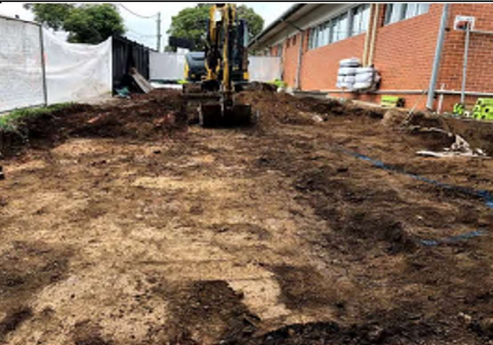
Photo 29: Removal of ACM containing fill material
