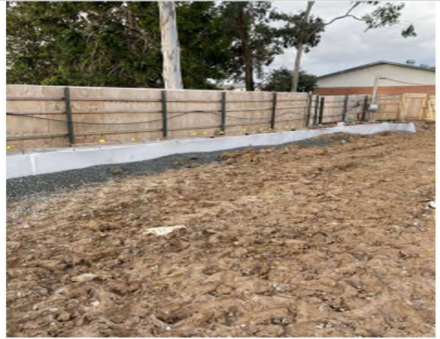
Photo 22: WSP inspection dated on 15/05/2020 - placement and pinning of geotextile material around the exposed walls through site
