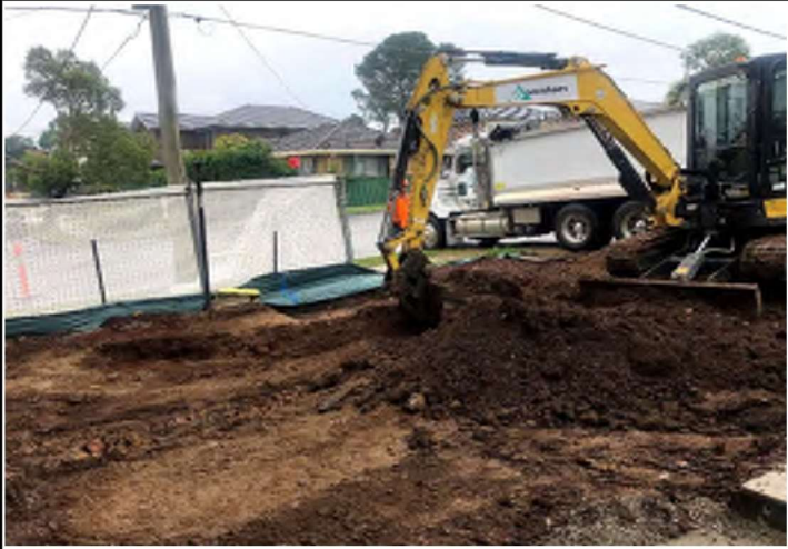
Photo 27: ACM contaminated fill material being transferred directly to the dump truck
