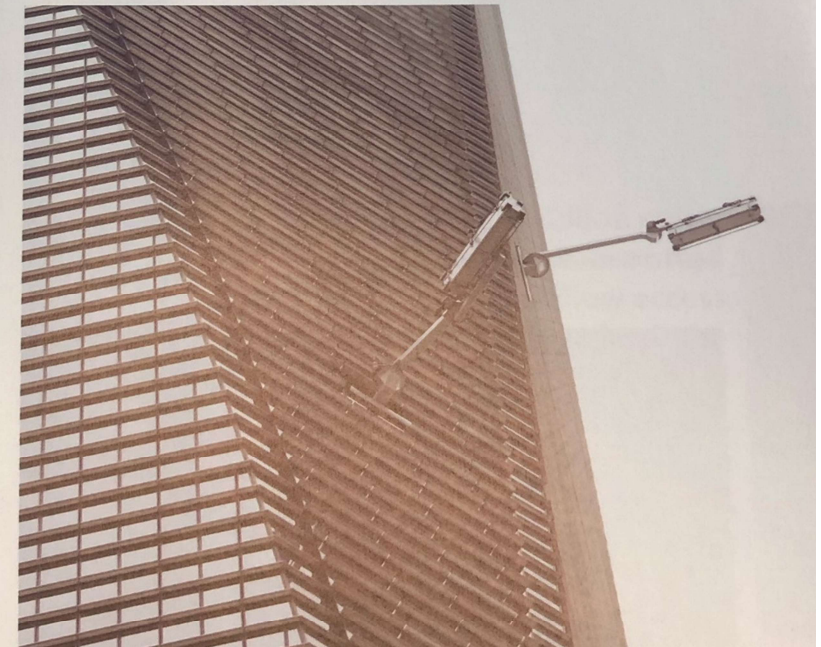
▲ Figure 2.3.5: Side elevation of the level 42 BMU. © CoxGorriyl
