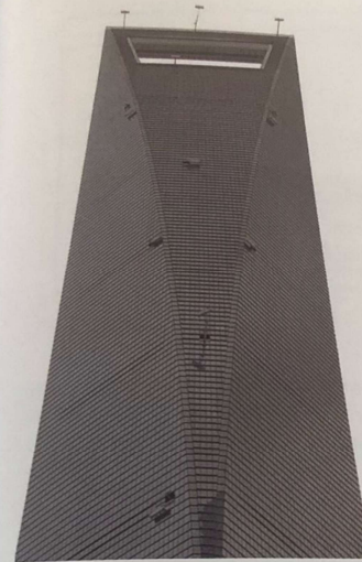
▲ Figure 2.3.4: This image shows Shanghai World Financial Center's BMUs, which are able to retract into the building to park. © Mori Building
