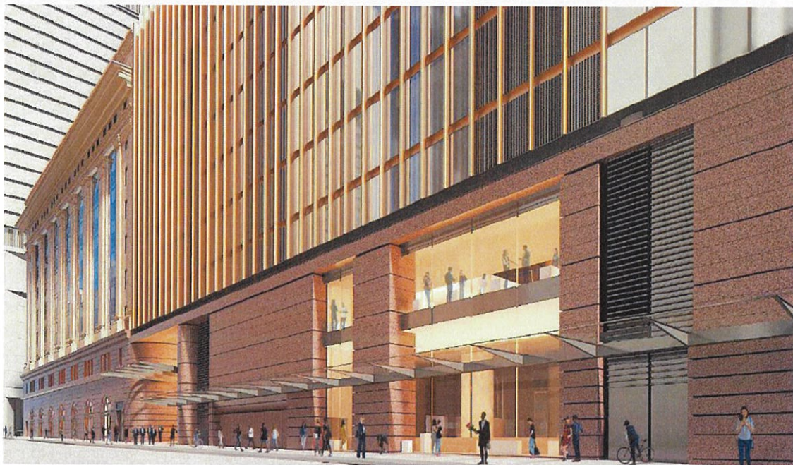
Figure 28 | Photomontage of proposal and 50 Martin Place looking south along Elizabeth Street (Source: Applicant's RtS)
