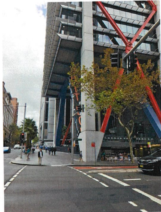
Figure 17 | Looking east along Hunter Street from corner Elizabeth Street. The “reverse podium” atria spaces and “tower to ground” format of 8 Chifley Square and Deutsche Bank building are shown (Source: DPE)
