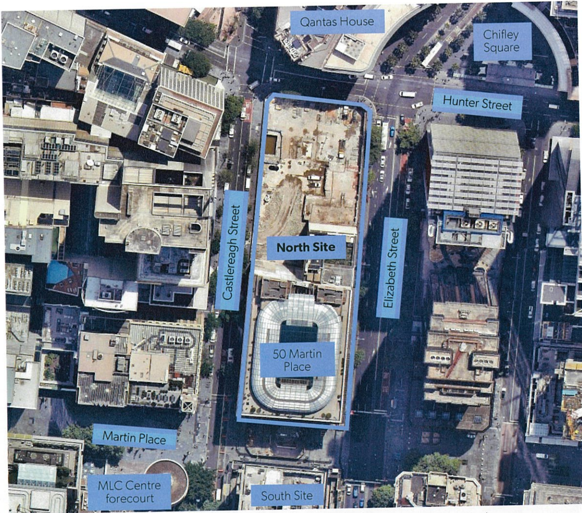
Figure 2 | North Site location and surrounds (Source: Nearmap with annotations)
