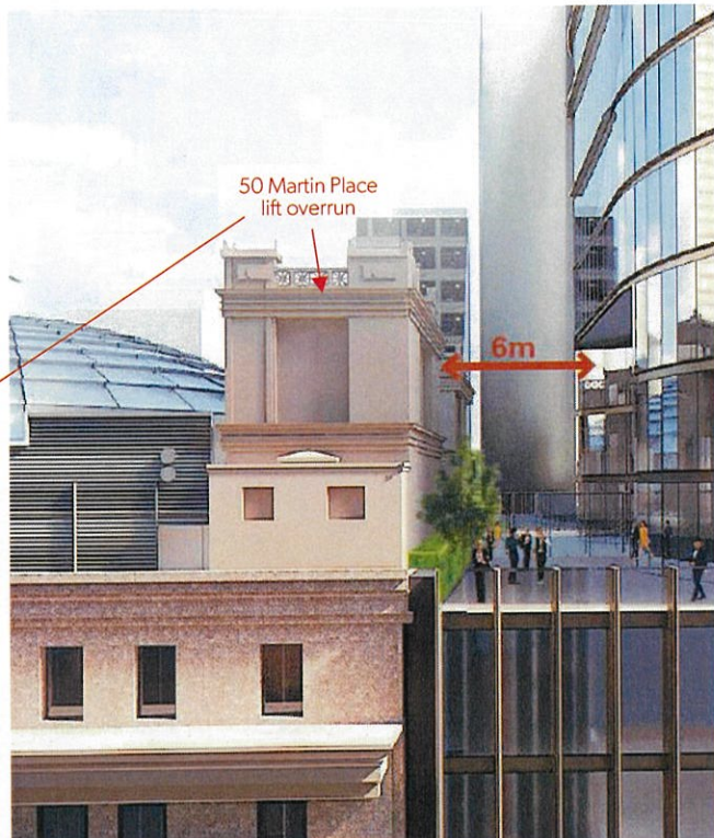
Figure 30 | Perspective showing proposed 6m setback to 50 Martin Place lift overrun (Source: Applicant's RtS)
