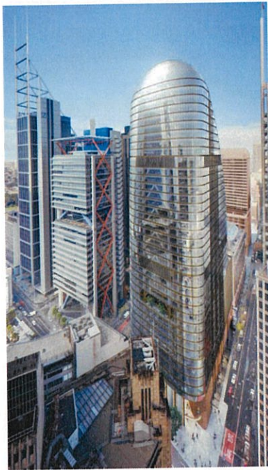
Figure 16 | Photomontage from corner Castlereagh Street and Hunter Street. The proposal has a consistent void height and proportions with 8 Chifley Square and Deutsche Bank, creating a strong visual connection along Hunter Street (Source: Applicant’s RTS)
