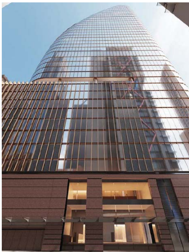
Figure 50 Eastern façade of the North Tower
