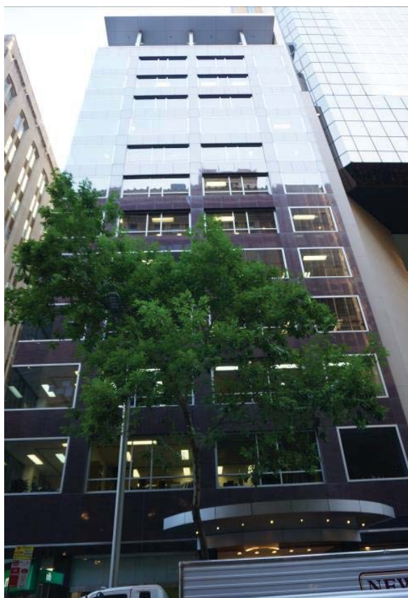
Figure 28 17 Castlereagh Street, as viewed from Castlereagh Street
