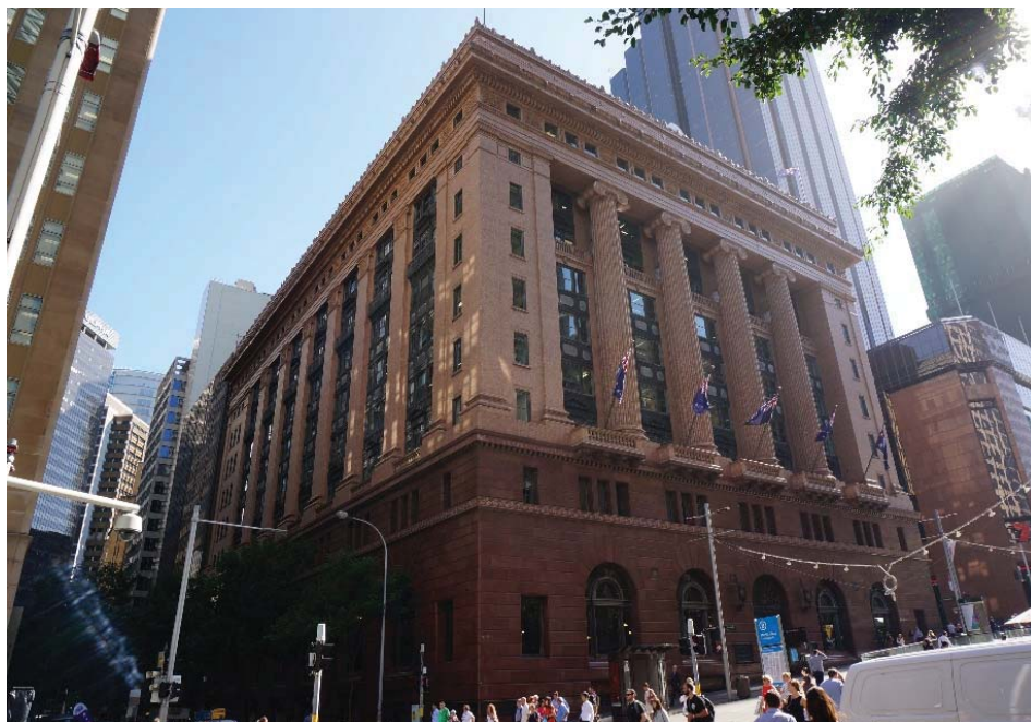
Figure 12 50 Martin Place as viewed from Martin Place and Castlereagh Street
