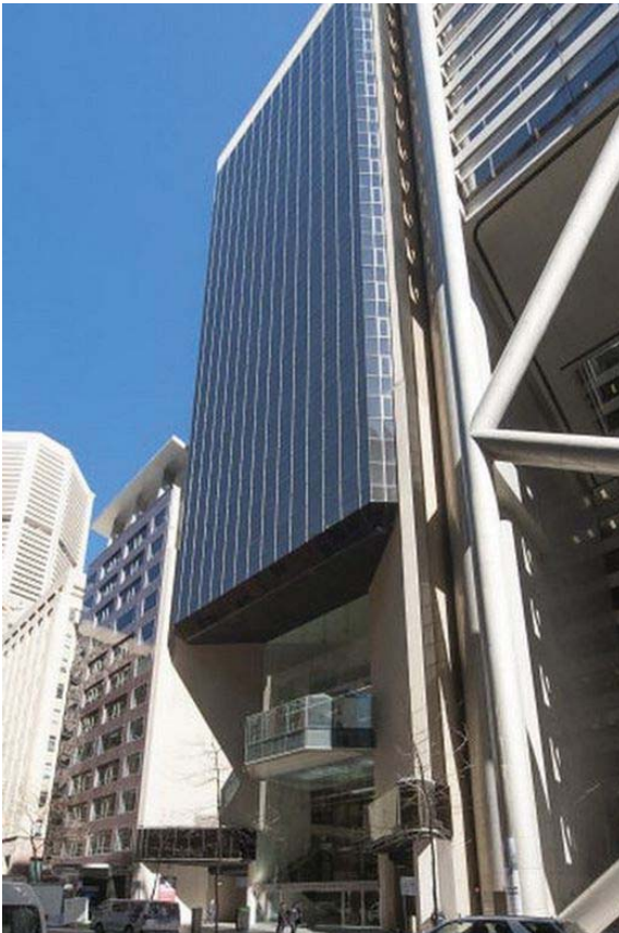
Figure 29 15 Castlereagh Street, as viewed from Castlereagh Street
