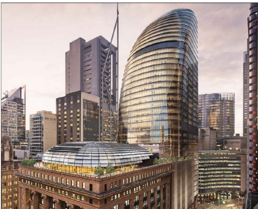
Figure 49 'Lense' on the southern façade
