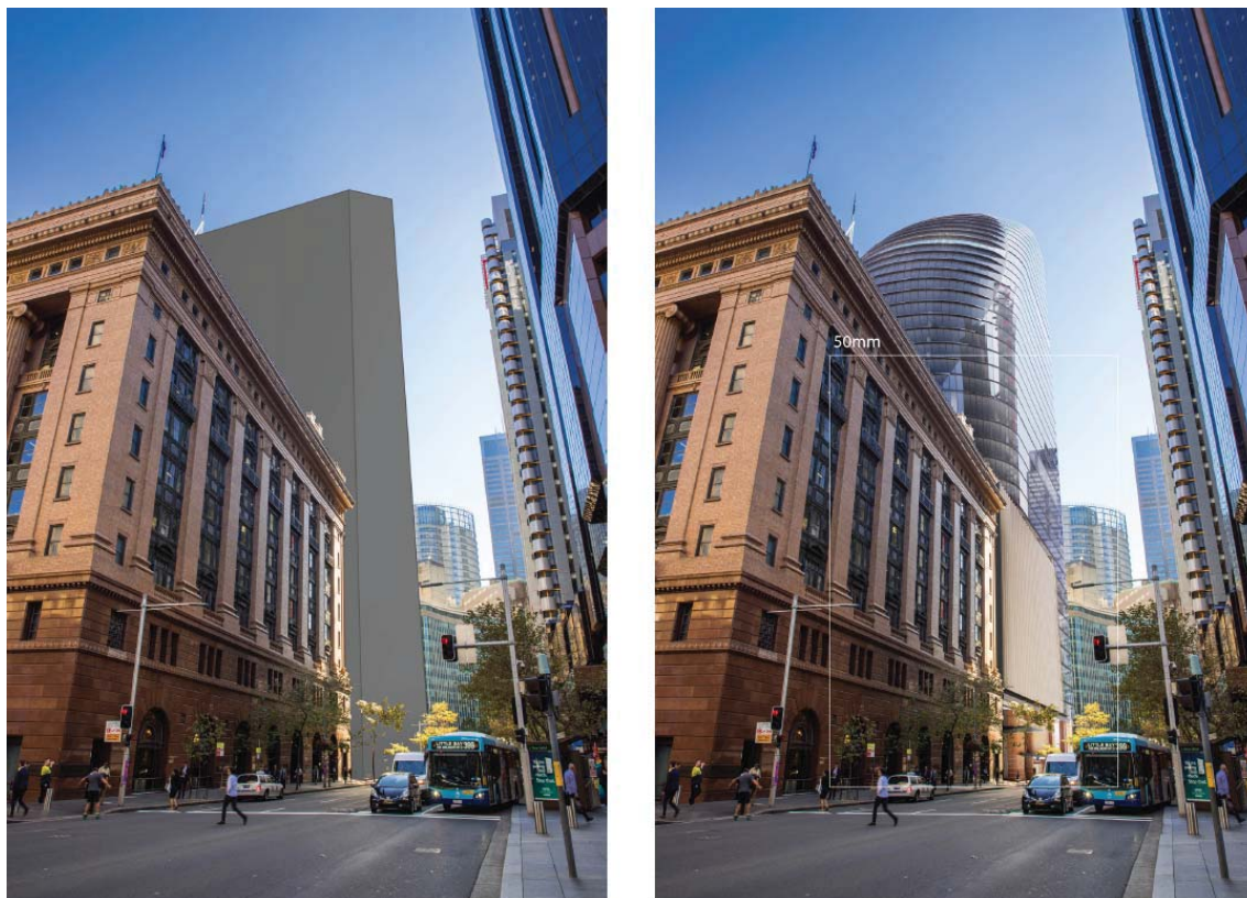
Figure 83 Building envelope (left) and detailed North Tower (right) as viewed from Elizabeth Street looking north
