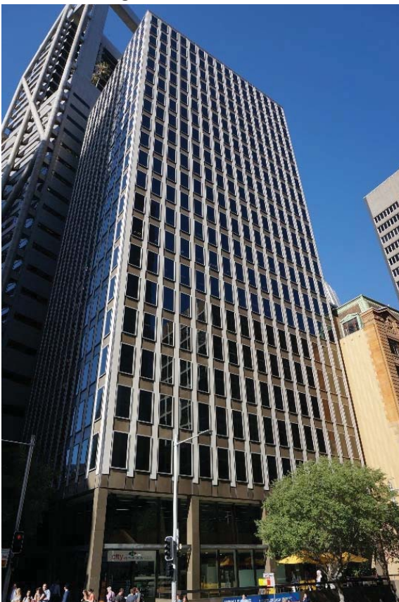
Figure 31 1-7 Castlereagh Street, as viewed from Hunter Street
