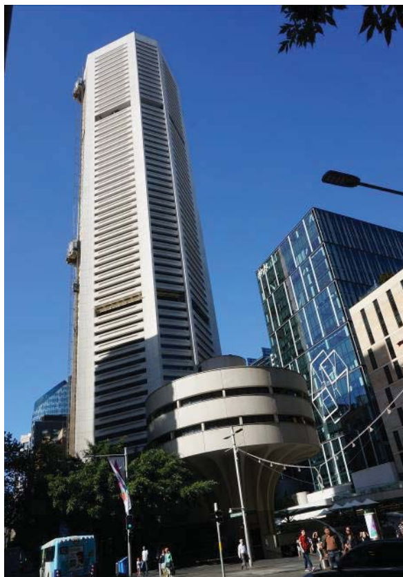
Figure 25 MLC Centre building as viewed from Martin Place
