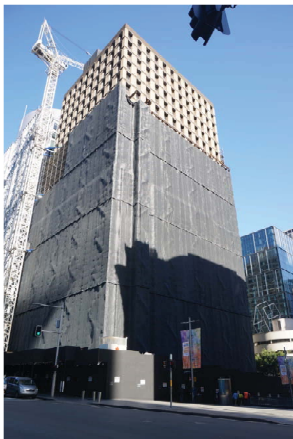
Figure 26 Demolition of 39-49 Martin Place underway on the South Site, as viewed from Elizabeth Street (July 2018)
