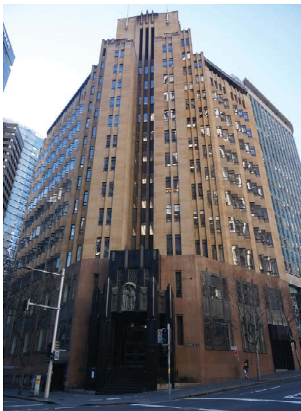
Figure 20 60-66 Hunter Street, as viewed from Bligh Street
