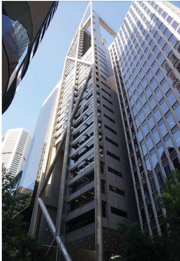
Figure 30 9 Castlereagh Street, as viewed from Castlereagh Street
