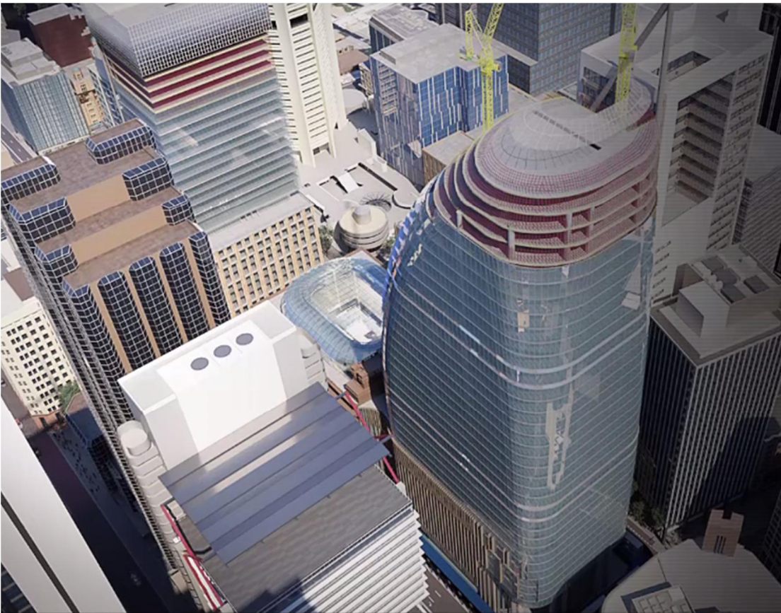
Figure 284 – North Tower Façade - Curtain Wall & Rooftop Dome
