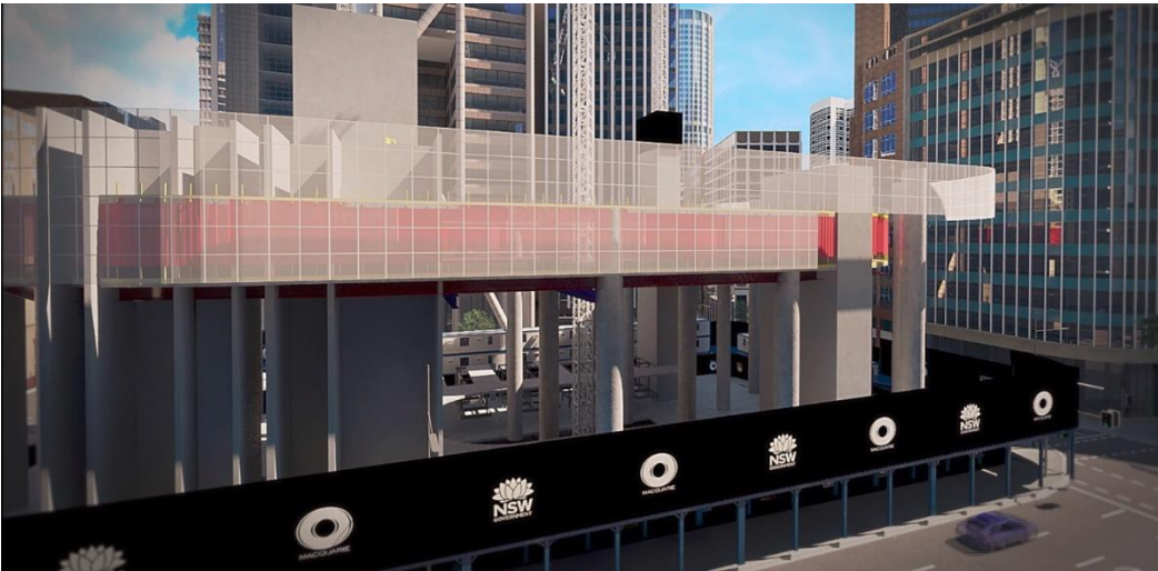
Figure 22 – L3 Jump Structure Jumped, facilitating early commencement typical floors above
