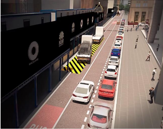
Figure 3 –B Class Hoarding North & South Buildings along Castlereagh St
