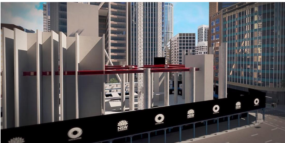
Figure 20 – L3 Jump Steel Structure
