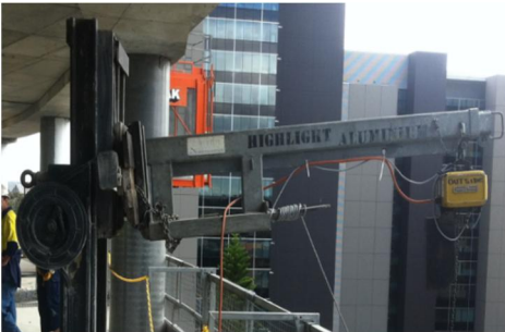
Figure 317 – Façade panels lifted with WR with jib.
