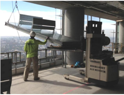
Figure 306 – Façade panels launched with WR.
