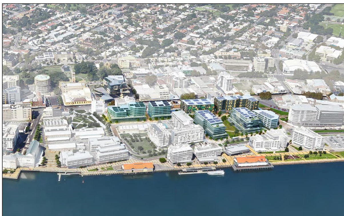
Figure 10 | Aerial perspective looking south towards Honeysuckle Precinct and the site (Source: Applicant's SRtS)
