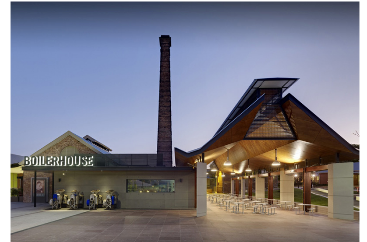
Boilerhouse heritage adaptation, WSU Rydalmere
