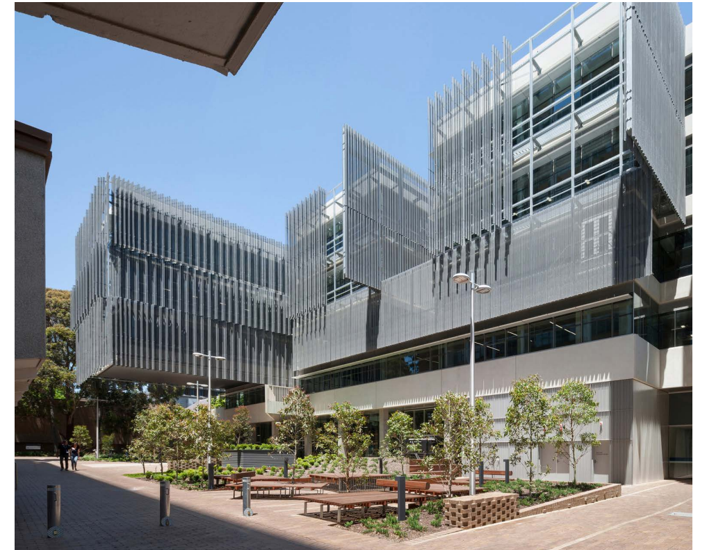
Building screening creates comfortable internal spaces, while ground level planting enhances biodiversity and regulates the microclimate. Melbourne School of Design, University of Melbourne
