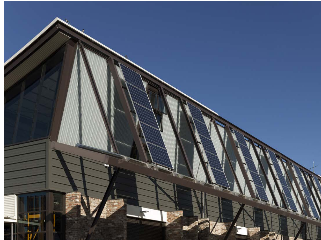
Photovoltaic cells are integrated with the roof form to enable energy collection Sustainable Buildings Research Centre, University of Wollongong, photographer: Richard Glover
