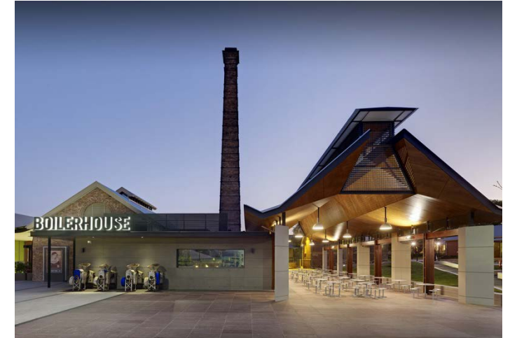
Boilerhouse heritage adaptation, WSU Rydalmere
