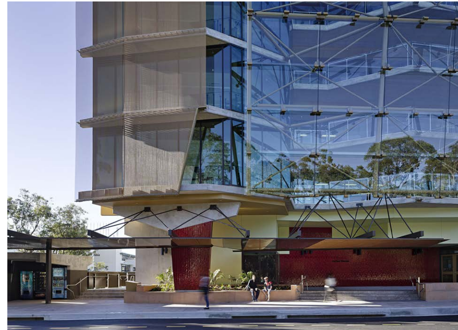
Glazing with sun shading screening provided to exposed facades Sir Samuel Griffith Centre
