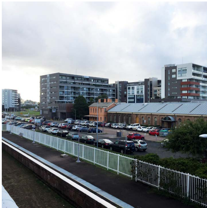
Heritage locomotive buildings
