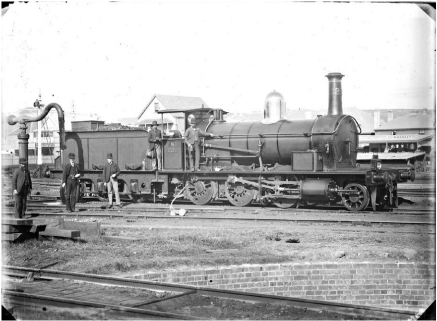
Locomotive and Turntable at Honeysuckle, installed 1857
