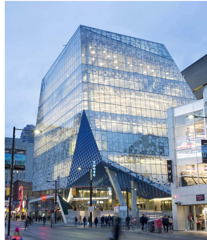
Figure 2.3.5: Ryerson Student Learning Centre, Toronto
