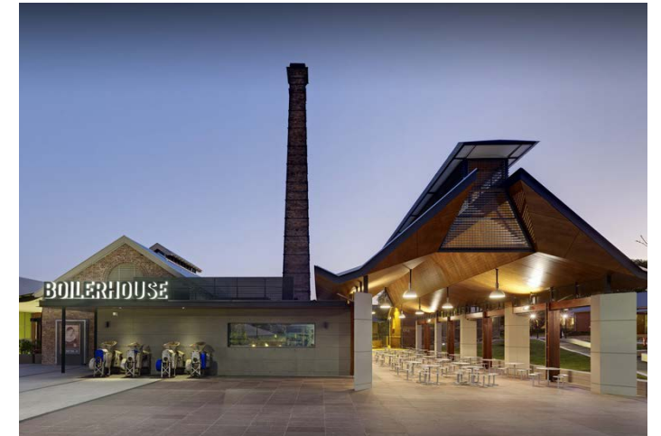
Boilerhouse heritage adaptation, WSU Rydalmere
