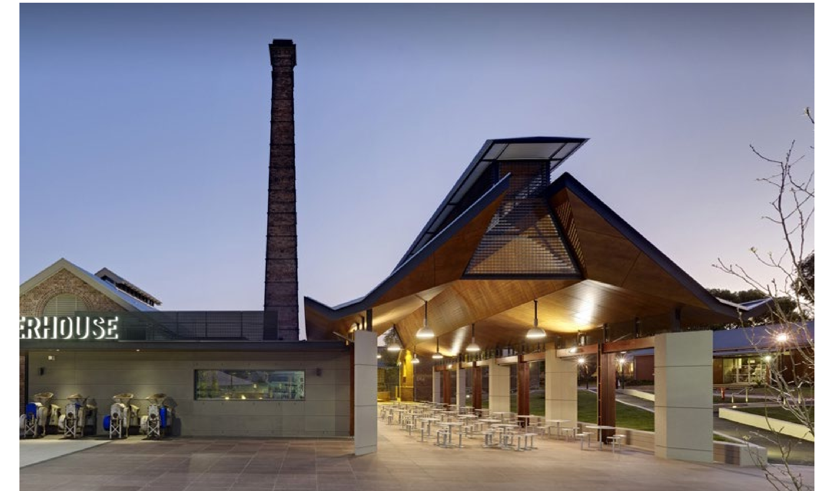
Boilerhouse heritage adaptation, WSU Rydalmere
