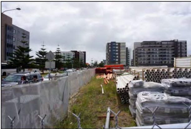
FIGURE 21: INTERIOR OF SITE 1, NORTH. VIEW EAST (SOURCE: CURIO 2018)
