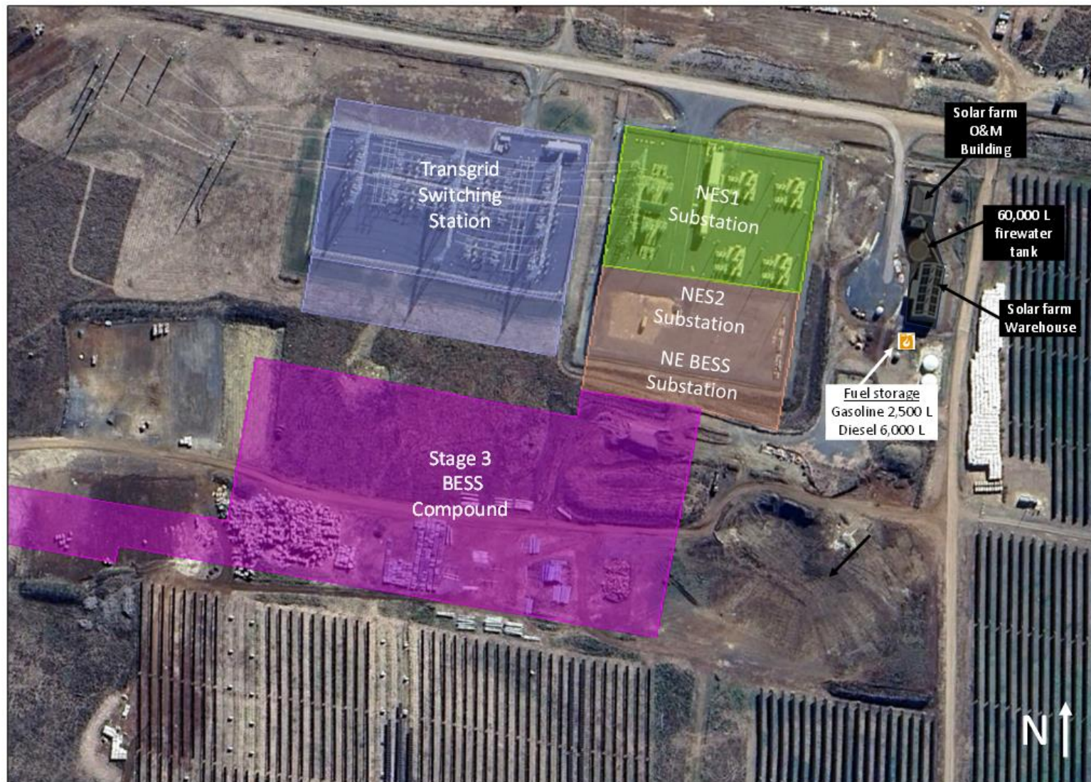
Figure 2-3 Substations and Stage 3 BESS compound area
