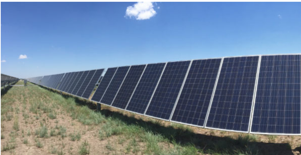
Photograph 4.1 PV module row with single axis tracking technology (Source: NexTracker 2018)
