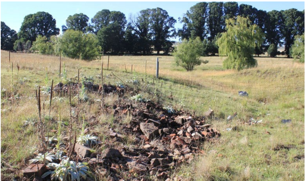
Plate 5.23 View of the demolition site - View east
