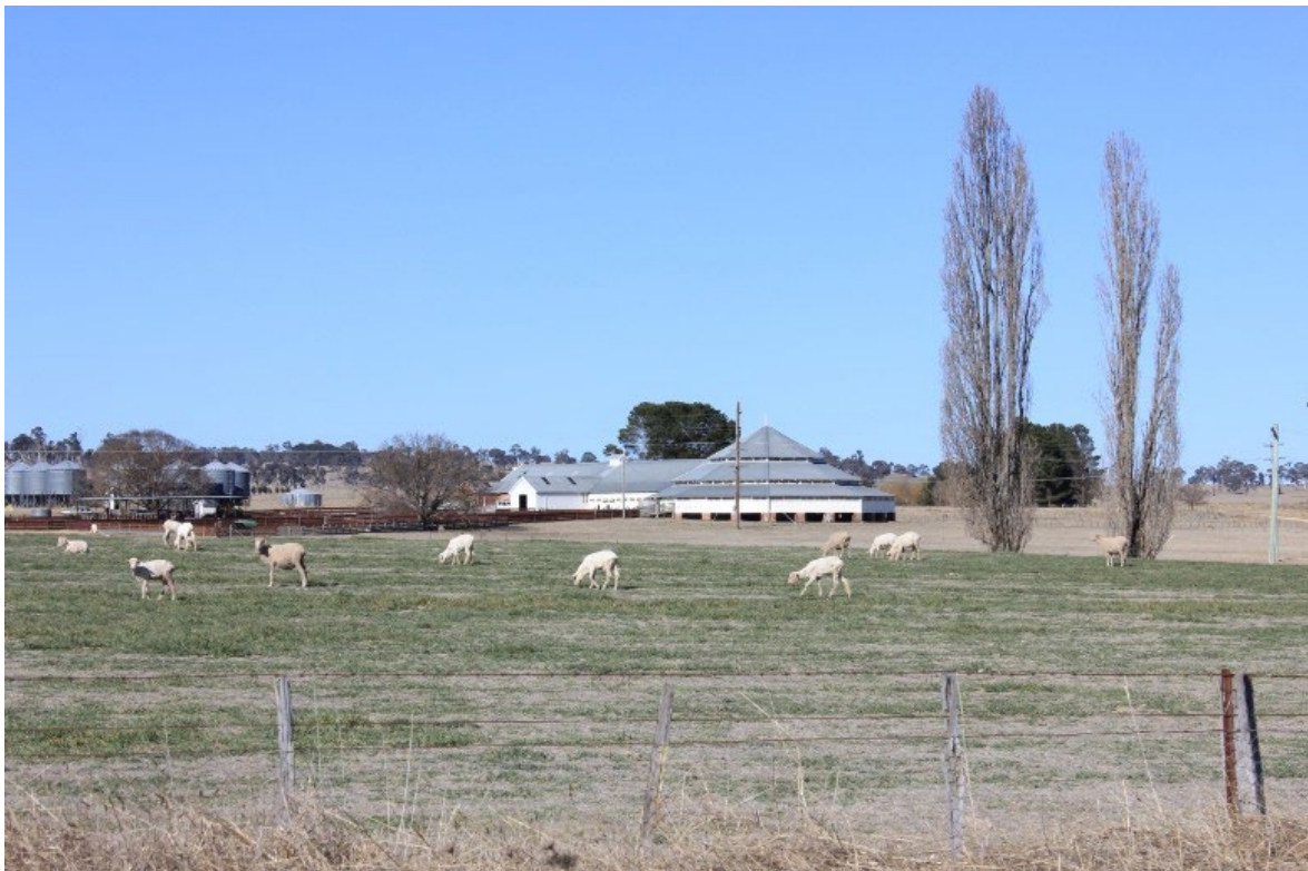
Plate 5.26 The earliest section of the Deeargee Woolshed - View south
