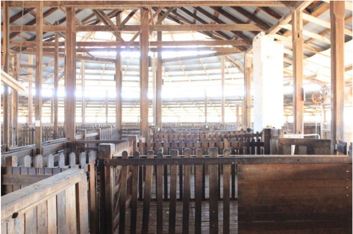
Plate 5.27 Centre catching-pens inside the Deeargee Woolshed
