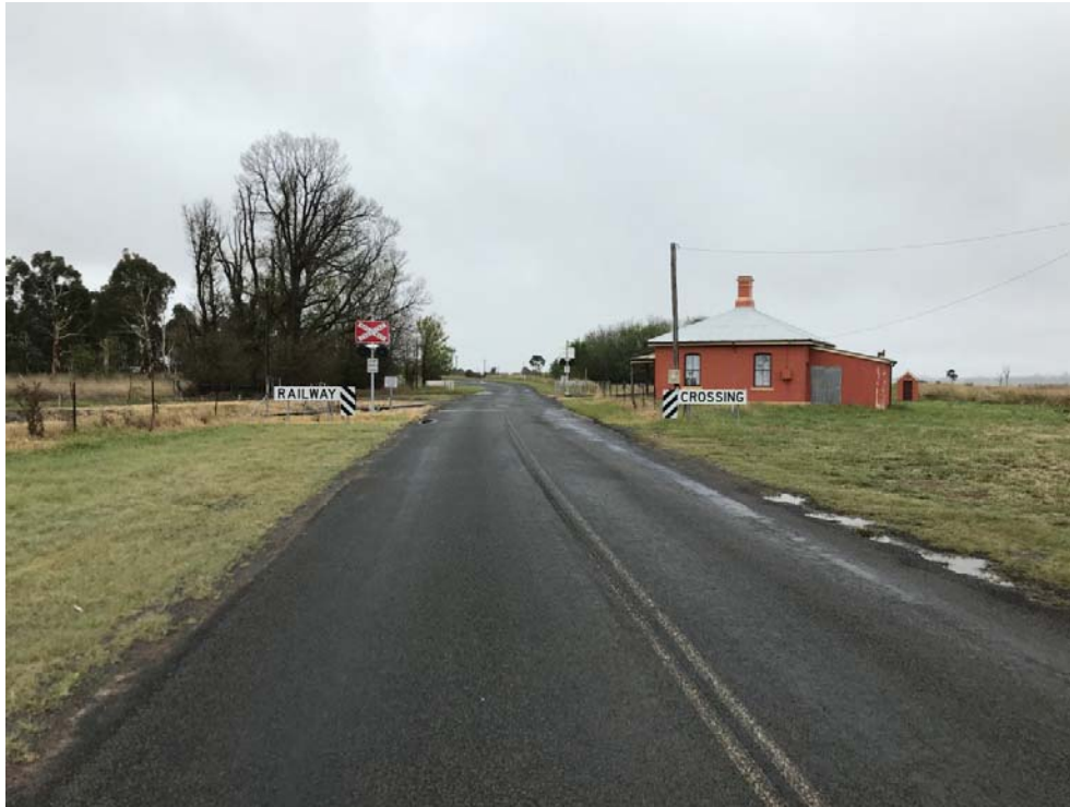
Photograph B.19 Rail crossing – Barleyfields Road
