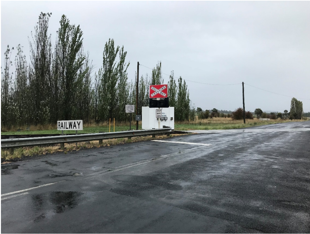
Photograph B.21 Rail crossing – Thunderbolts Way
