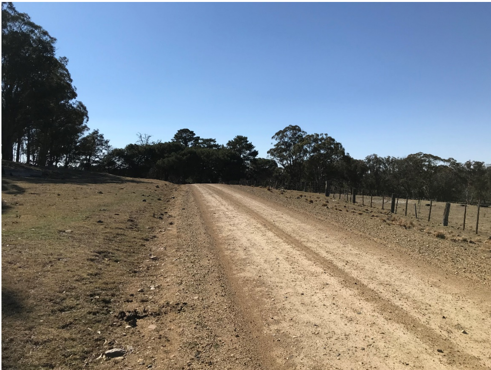
Photograph C.8 Munsies Road access point looking east – central array
