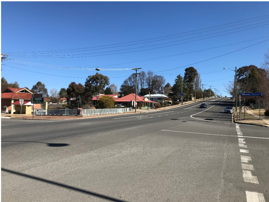
Photograph B.10 New England Highway / Thunderbolts Way intersection (looking south-west)
