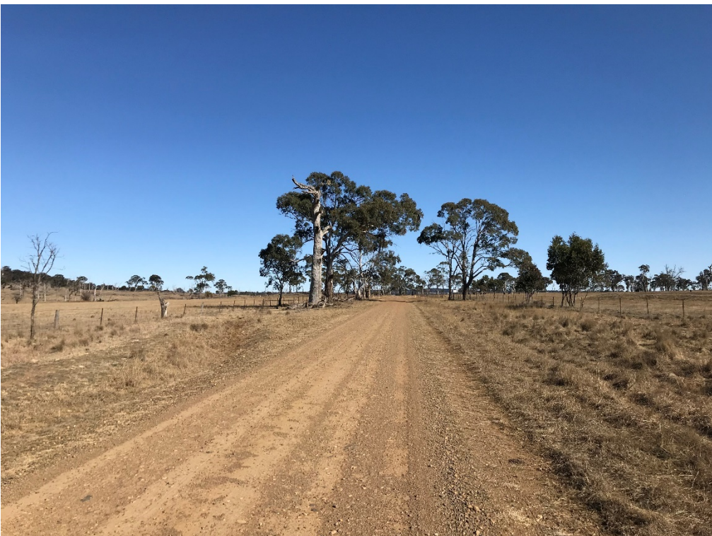
Photograph B.2 Big Ridge Road looking west (6 km from Barleyfields Road)
