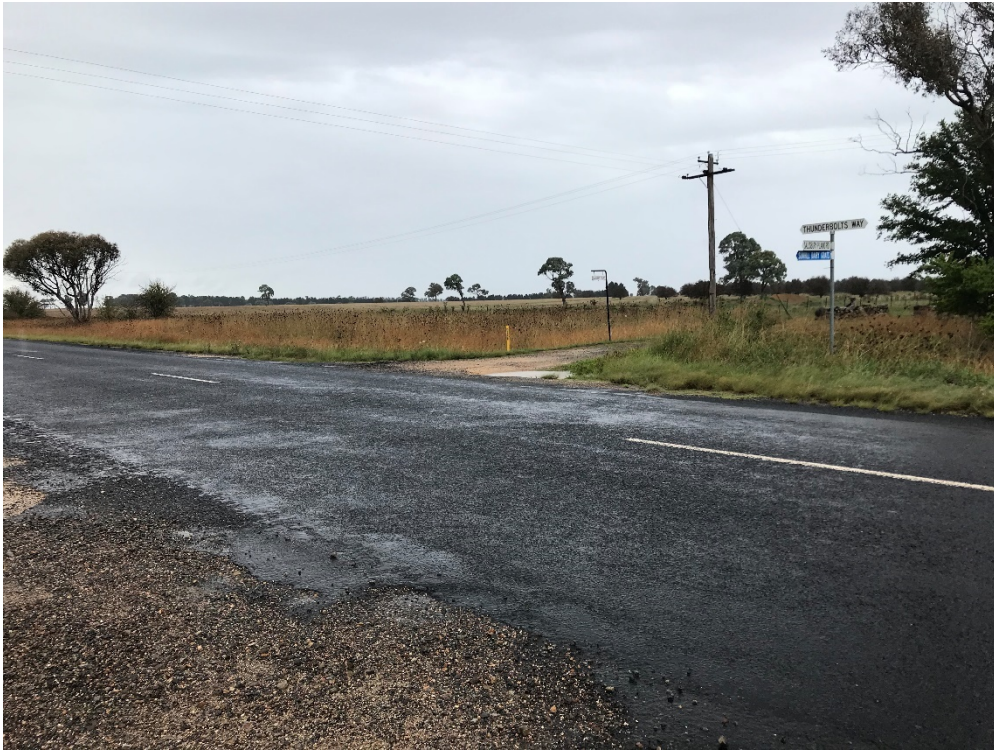
Photograph B.17 Thunderbolts Way / Salisbury Plains Road intersection (looking north)
