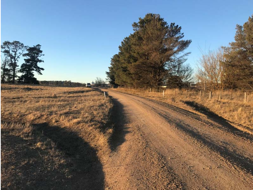
Photograph C.11 Hillview Road access point looking north – southern array
