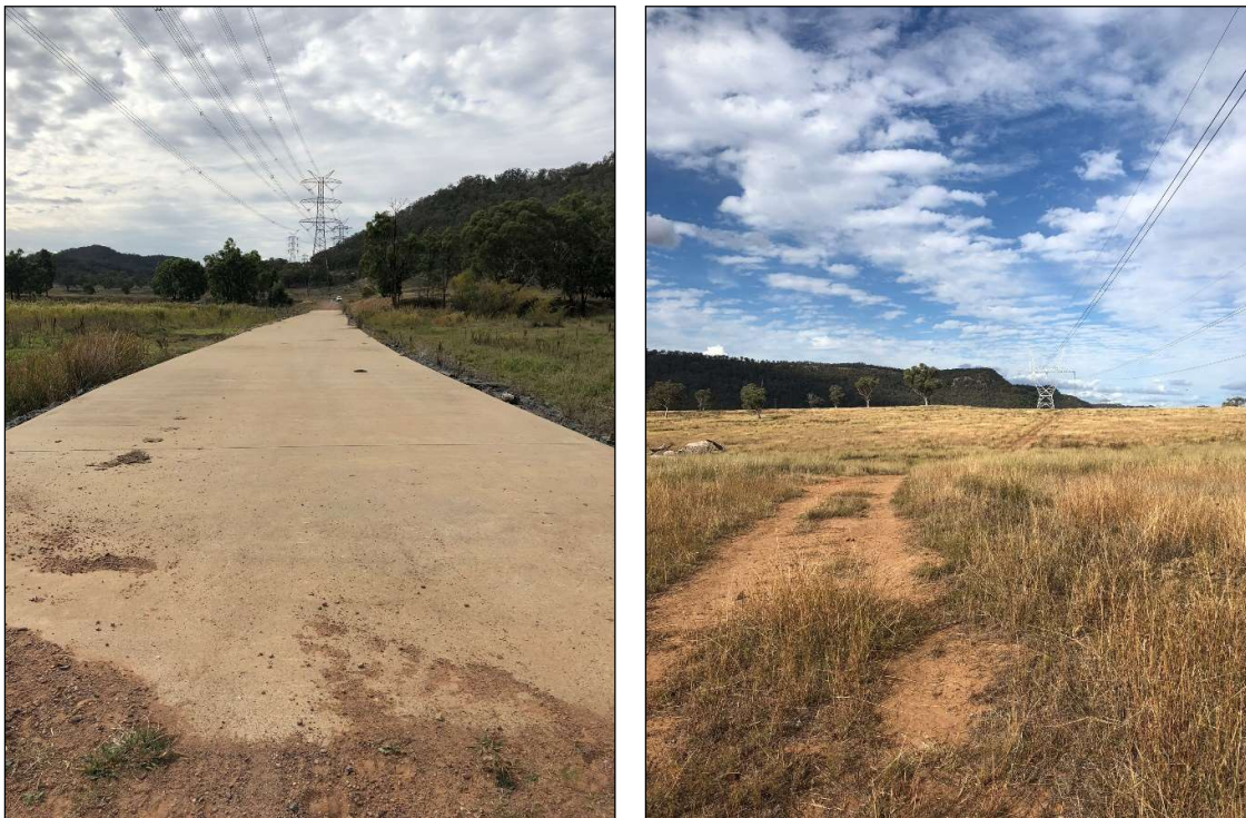
Figure A-10 Wollar Creek causeway along existing TransGrid access (left) and 330kV TransGrid transmission line between Wollar substation and proposed new substation location (right)
