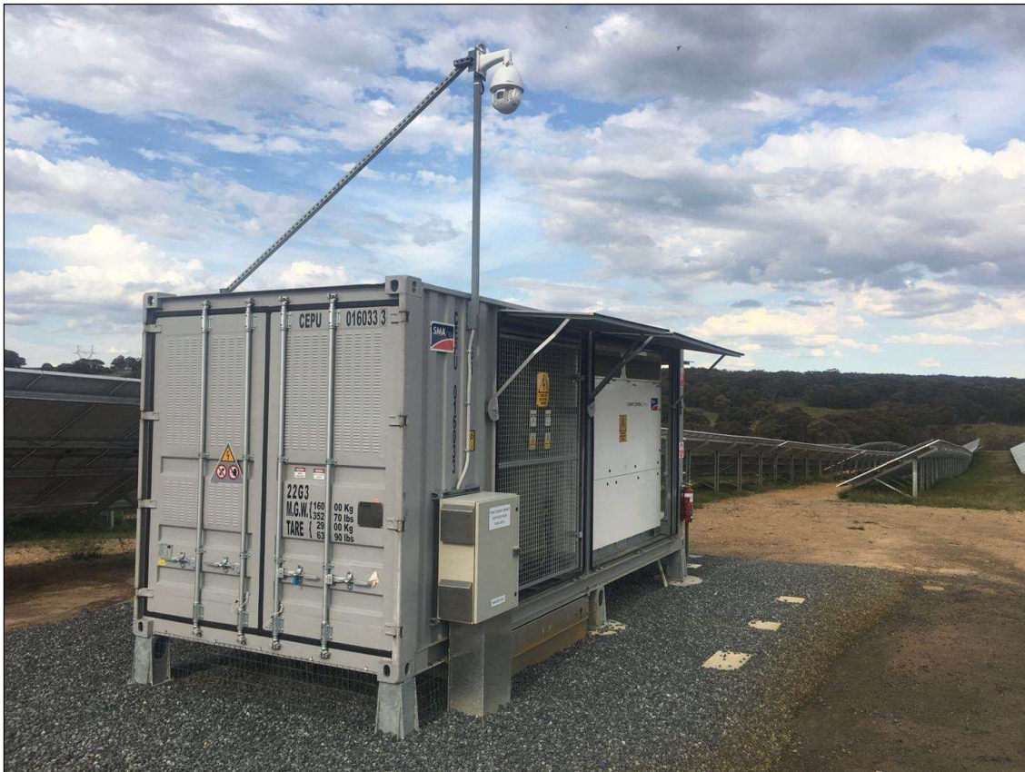
Figure A-6 Typical illustration of a PCU within the array.
