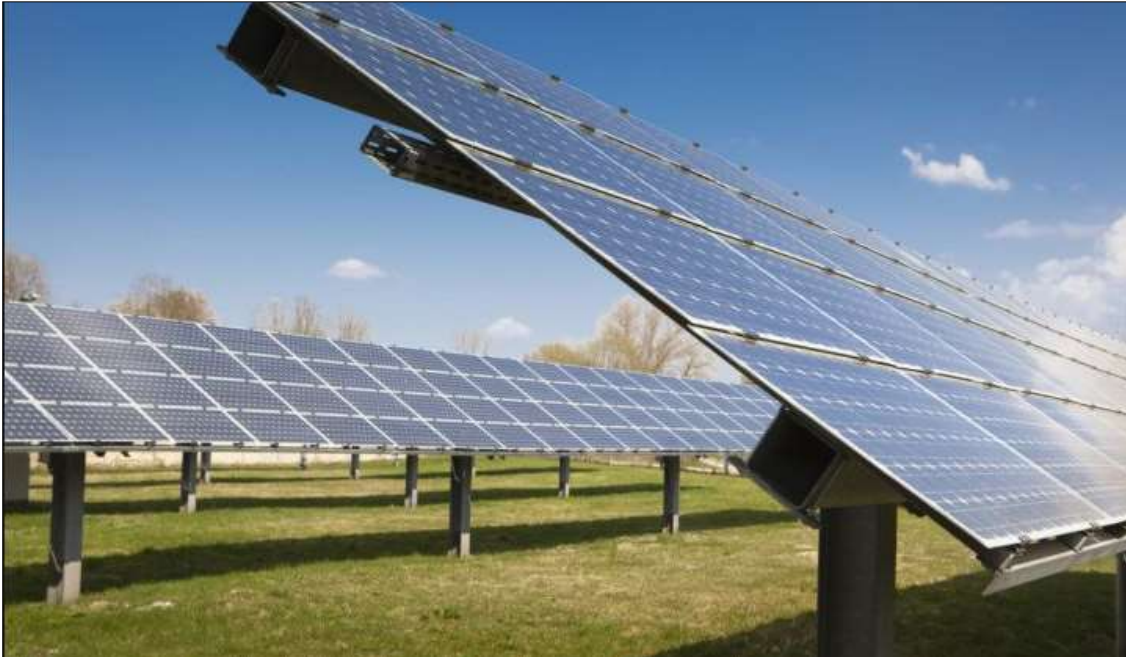
Figure A-3 Typical fixed tilted system.
