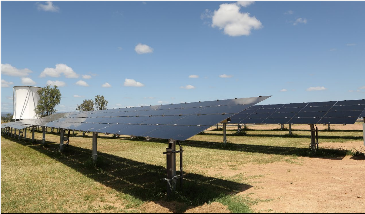
Figure A-3 Typical single-axis tracking system.
