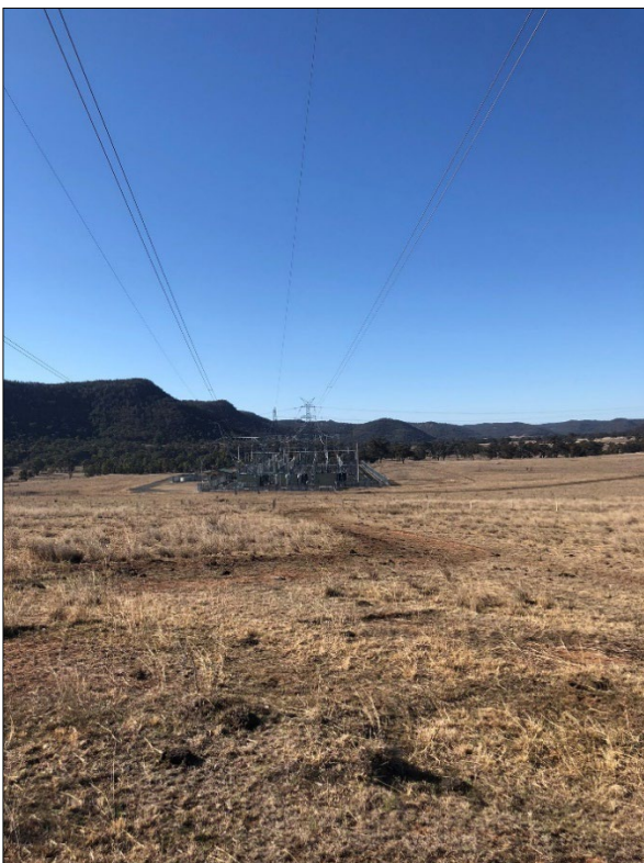
Figure A-7 330kV transmission line within 60m easement traversing the proposal site and connecting to the Wollar substation.
