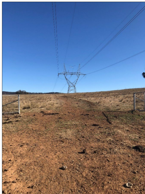
Figure A-7 330kV transmission line within 60m easement traversing the proposal site and connecting to the Wollar substation.
