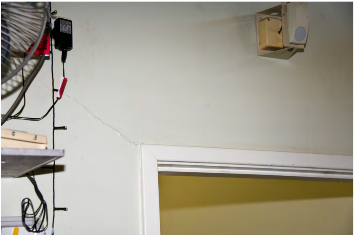
Block H. Interior. Eastern room. Room K6F. Western face. Cracked cladding.
