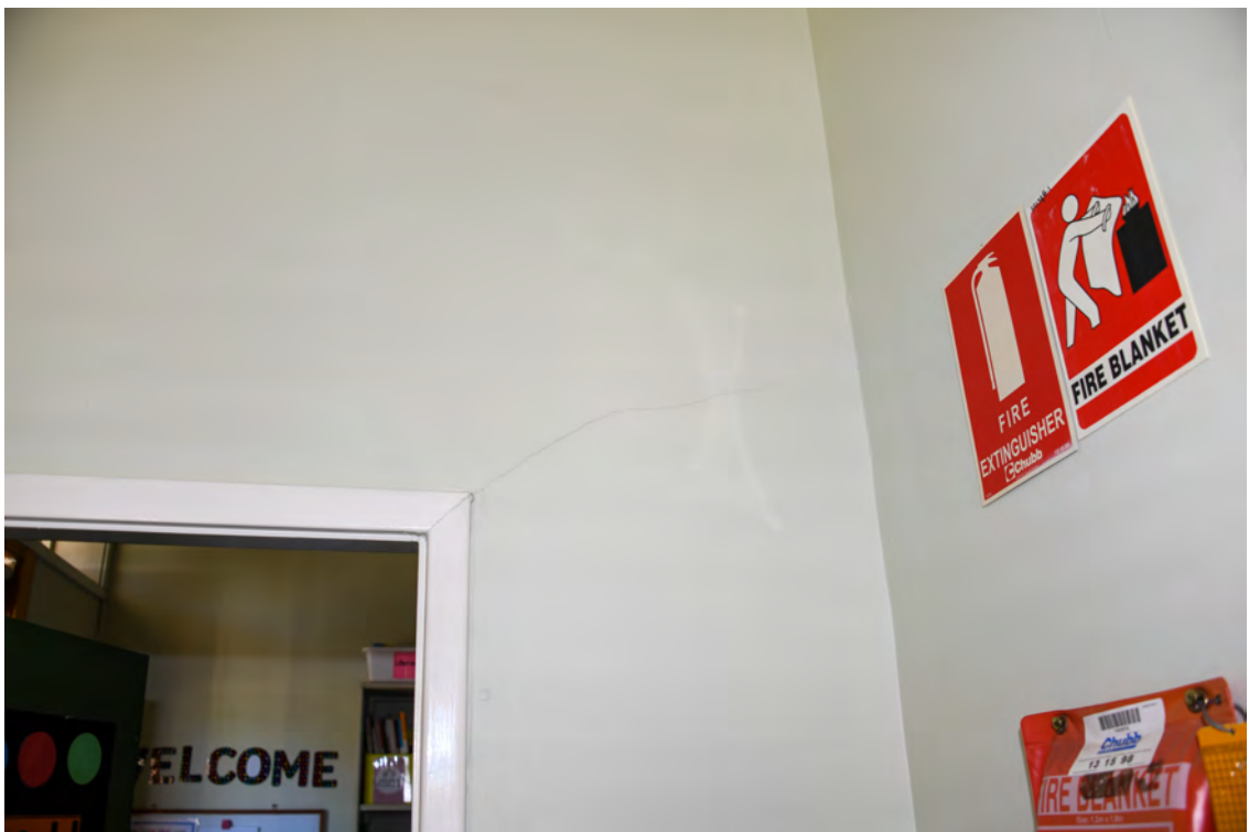
Block H. Interior. Eastern end. Foyer. Eastern face. Cracked wall cladding.
