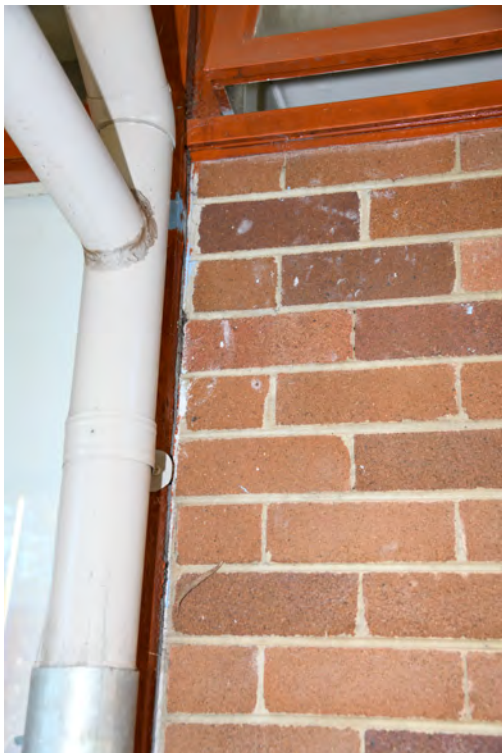
Block H. Northern elevation. Western end. Heading east. Control joint in the brickwork.
