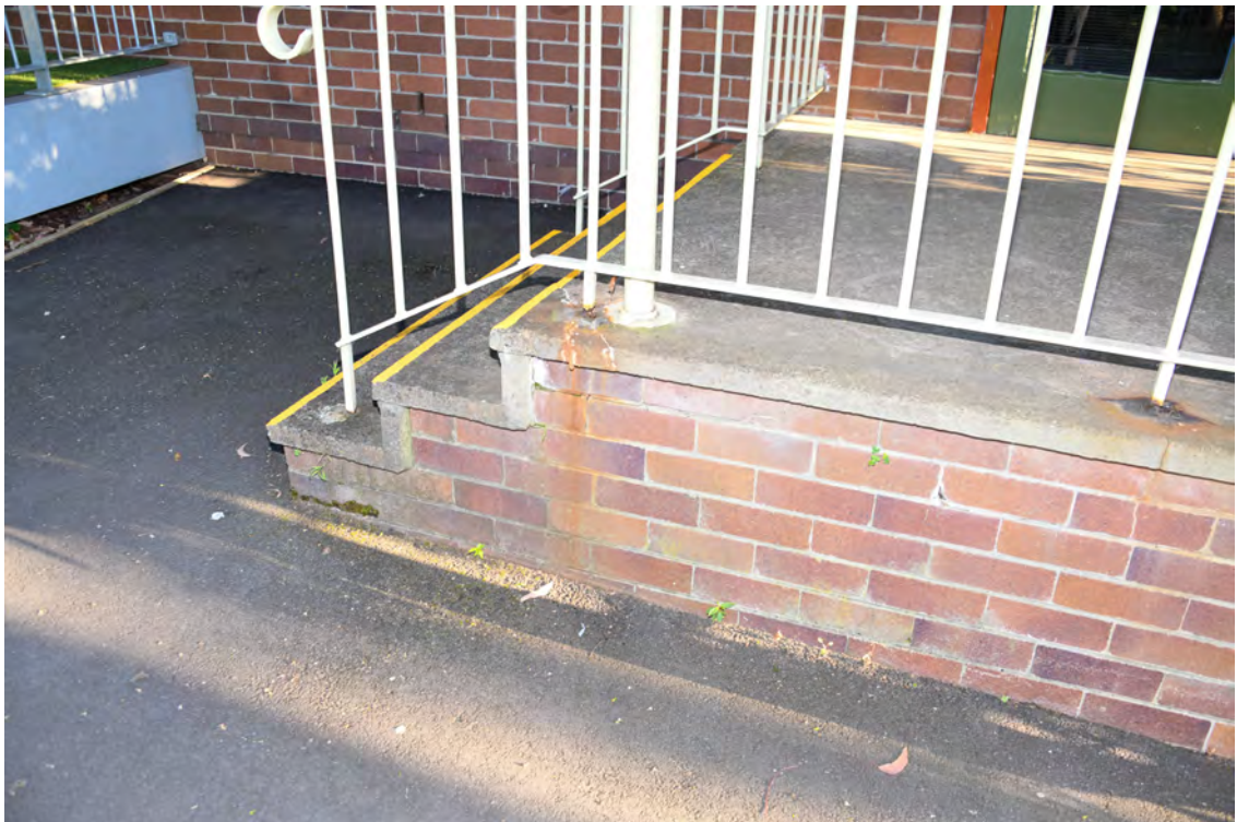
Block H. Southern elevation fronting Carlingford Road. Heading west. Eastern building entry. Cracked concrete landing.
