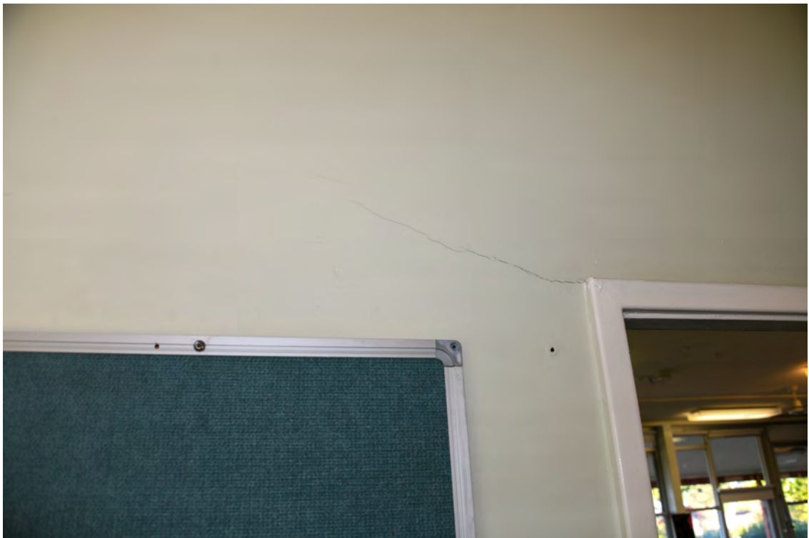
Block H. Interior. Eastern end. Foyer. Southern face. Western end. Cracked cladding stemming out from the doorway.
