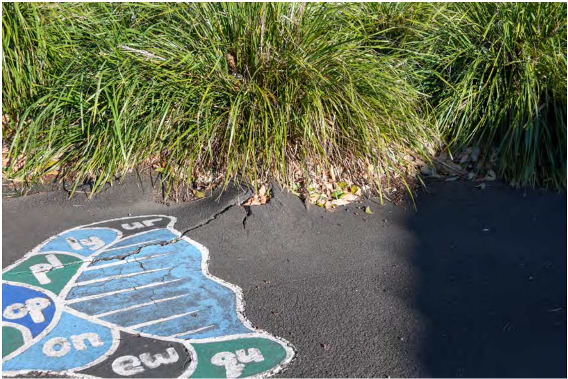
Block D. Eastern elevation. Southern end. Damaged adjacent asphalt paving.
