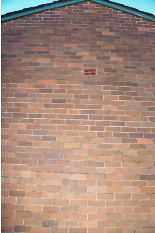
Block F. Western elevation. Movement to the brickwork.
