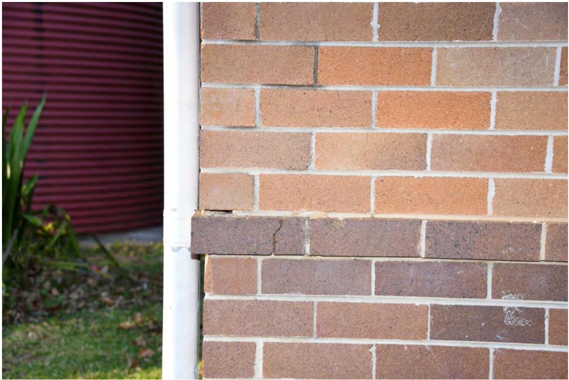
Block F. Northern elevation. Eastern end. Cracked brick.
