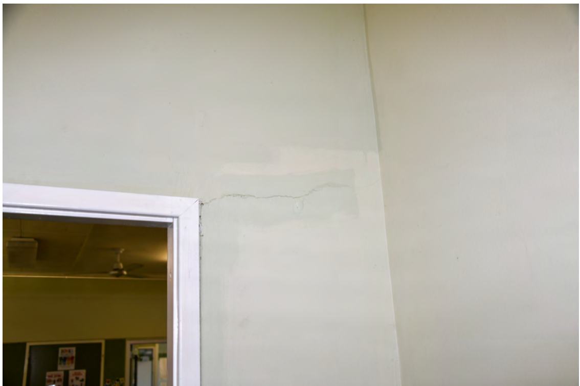
Block H. Interior. Foyer outside Room HR0027. Eastern face. Cracked wall cladding.
