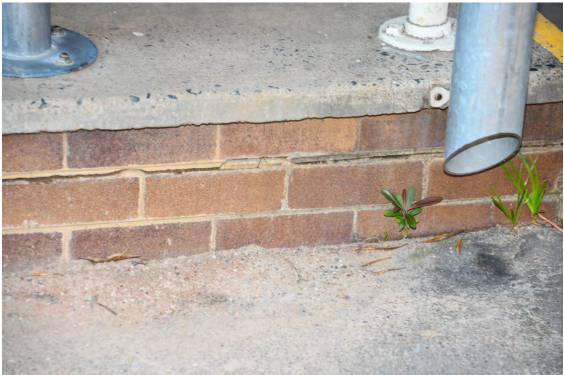
Block H. Northern elevation. Western stairs. Movement to the brickwork.
