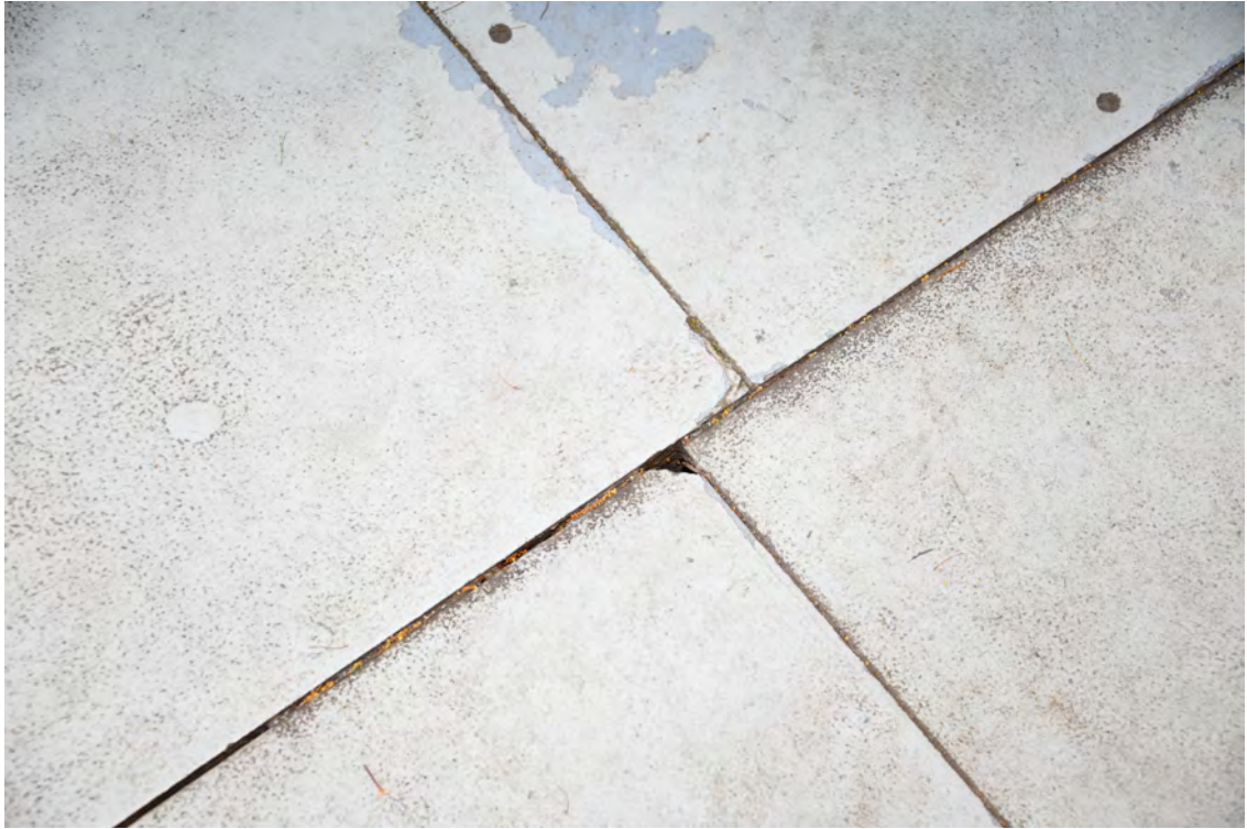
Block I. Southern side of the building. Access ramp. Chipped edges of the flooring.
