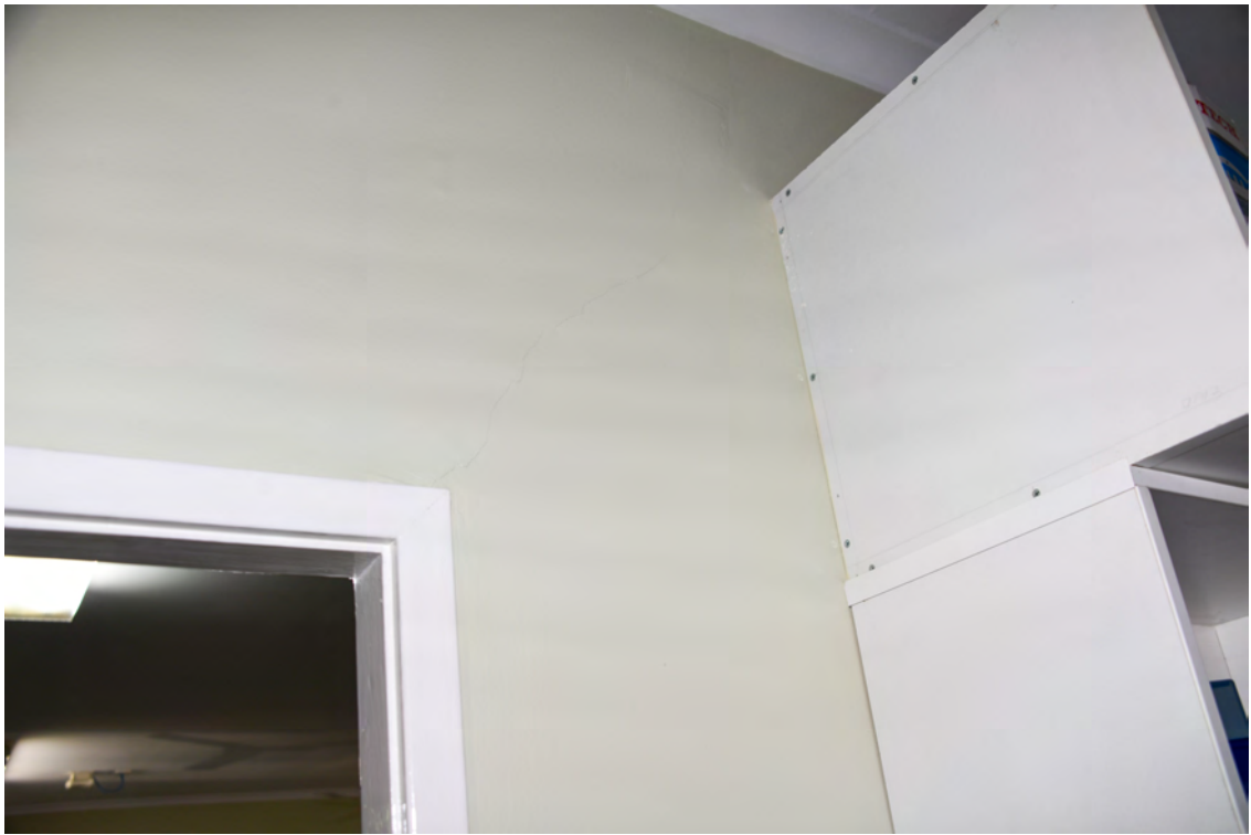
Block A. Building foyer. Northern face. Cracked wall cladding.
