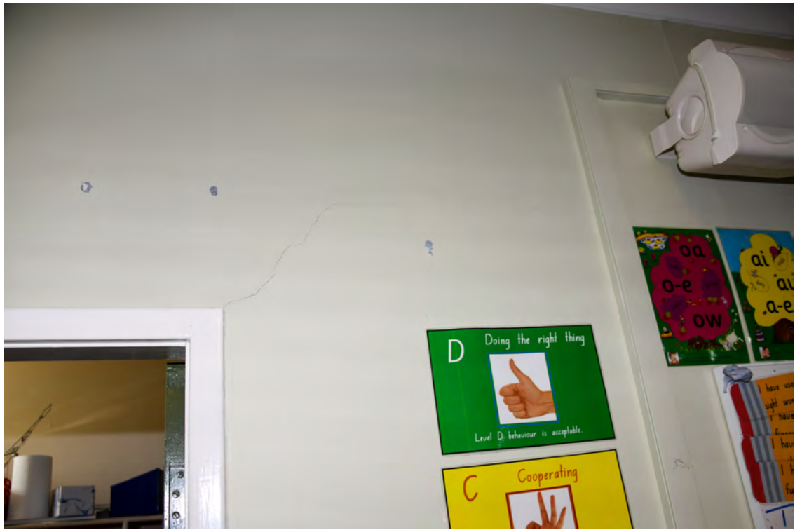
Block A. Room 1G. Southern face. Cracked wall cladding.
