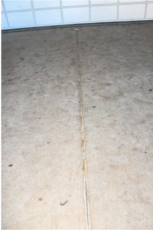
Block M / Hall / The Aurora Centre. COLA. Record of the concrete paving. Control joint in the paving.
