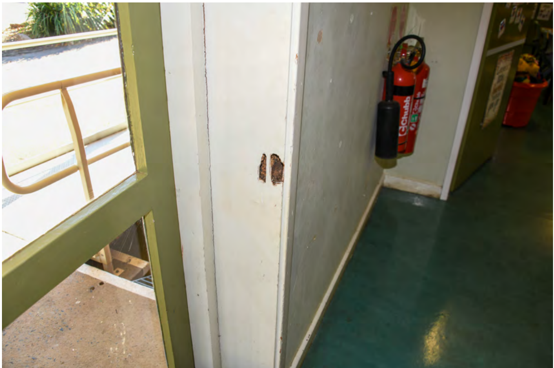
Block H. Interior. Foyer. Northern face. Eastern reveal to the doorway. Rot.
