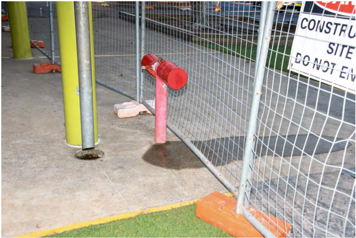
Block M / Hall / The Aurora Centre. Northern elevation. Western end. Leaking hydrant.
