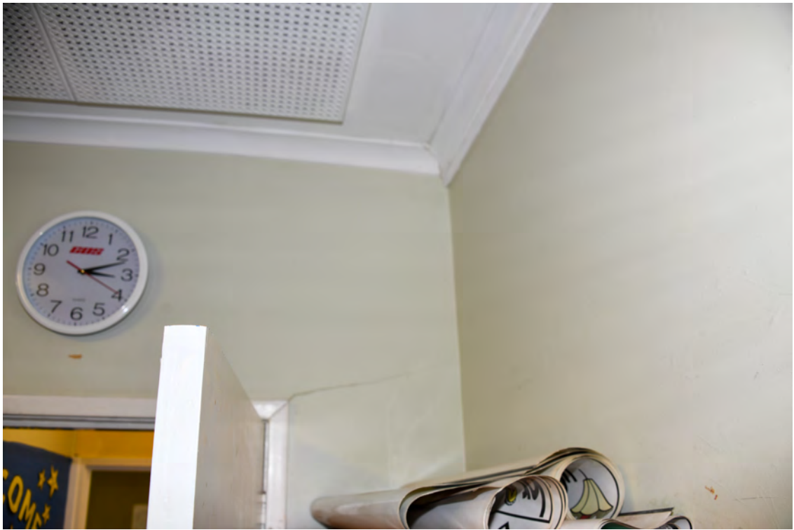
Block F. Interior. Second eastern room (Mrs Wiltshire). Eastern face. Cracked wall cladding.
