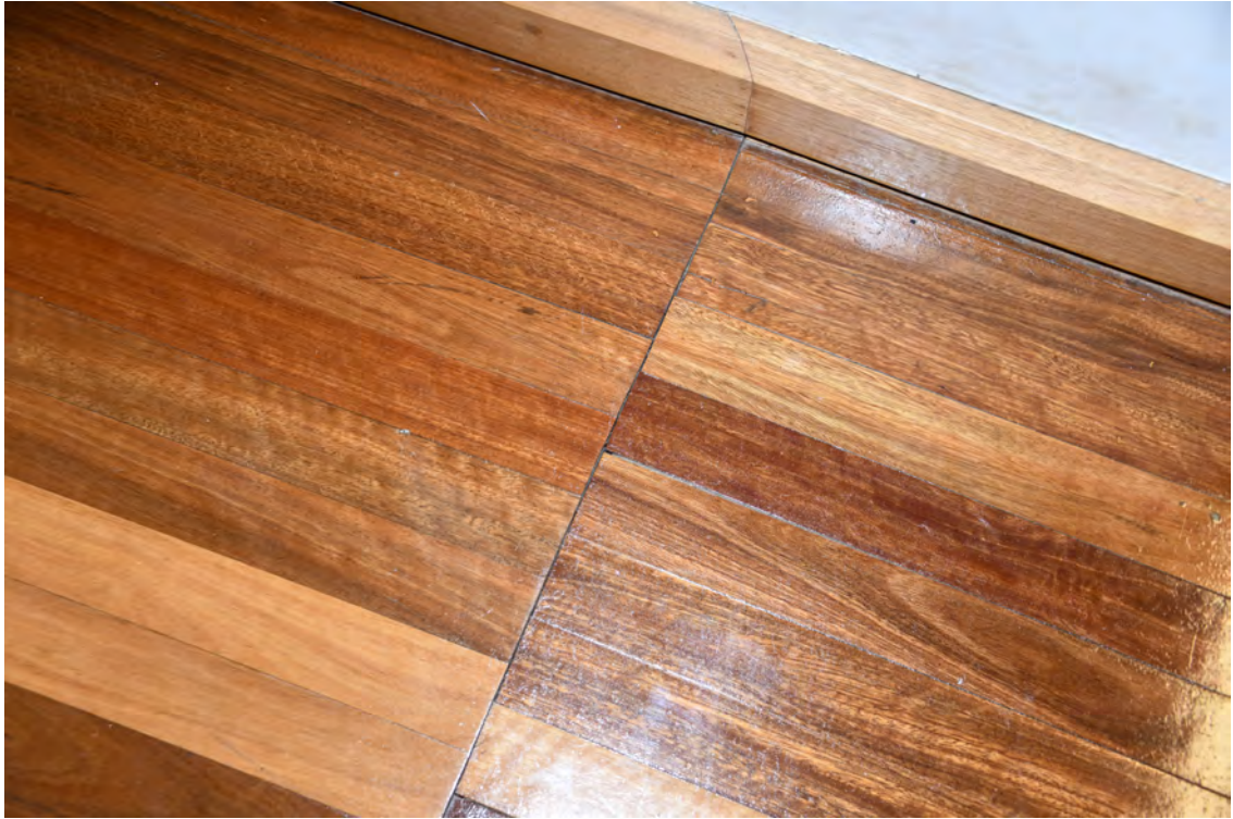
Block M / Hall / The Aurora Centre. Interior. Eastern face. Heading south. Movement at the join in the flooring.
