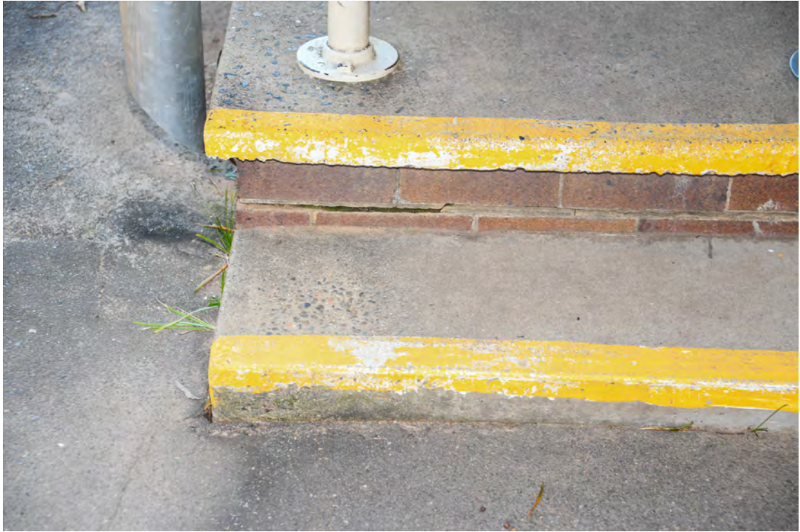
Block H. Northern elevation. Heading east. Eastern set of doors. Movement to the brick tread.
