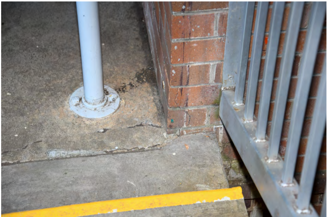
Block F. Southern elevation. Eastern end. Cracked brickwork and concrete paving.
