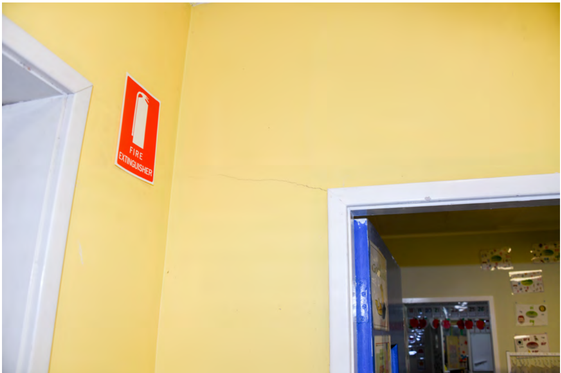
Block F. Interior. Entry Foyer (room 14). Western face. Cracked wall cladding.
