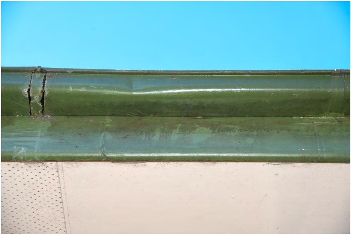
Block F. Northern elevation. Western end. Indentation in the roof gutter.
