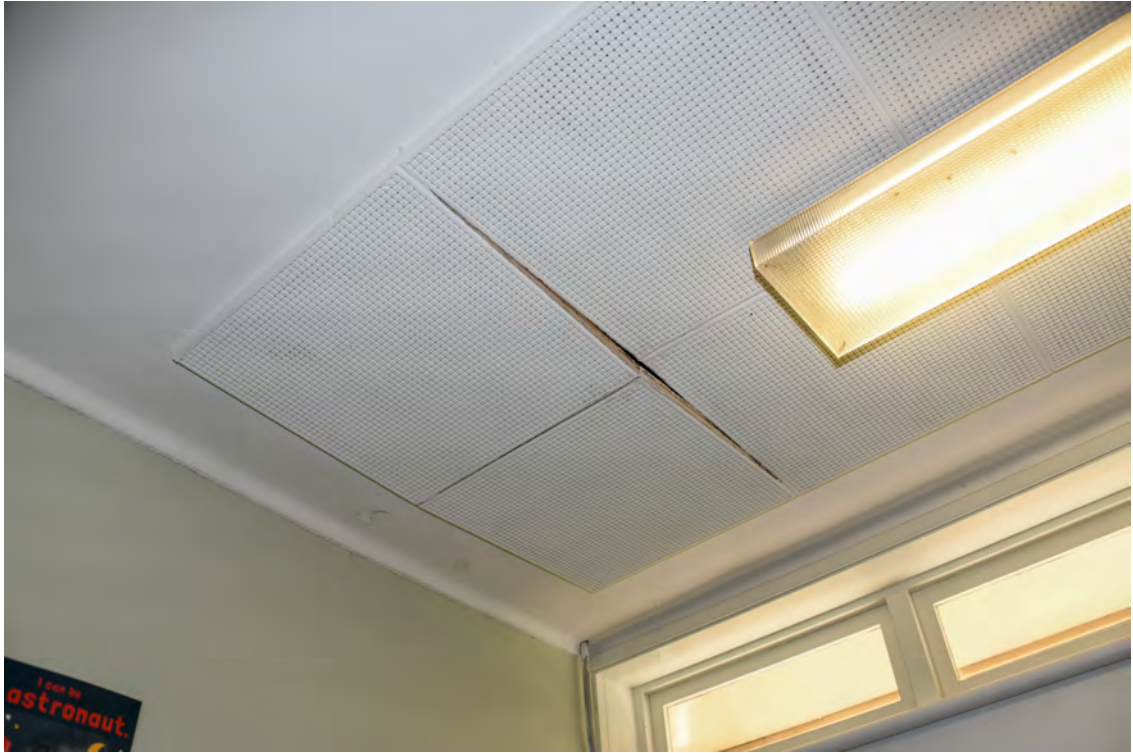
Block H. Interior. Room HR0027. Ceiling. Movement to the ceiling tiles in the north-western corner of the room.
