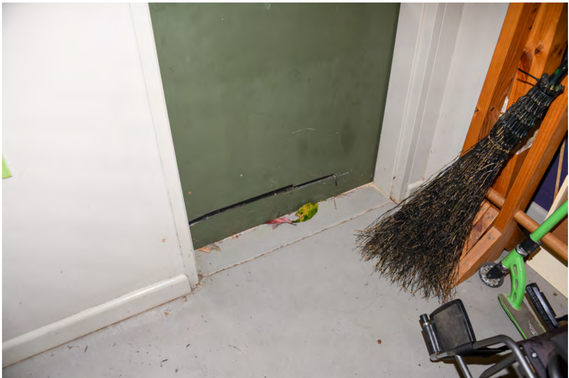
Block M / Hall / The Aurora Centre. Interior. Southern face. Boys Change Room. Southern face. Damage to the base of the door.
