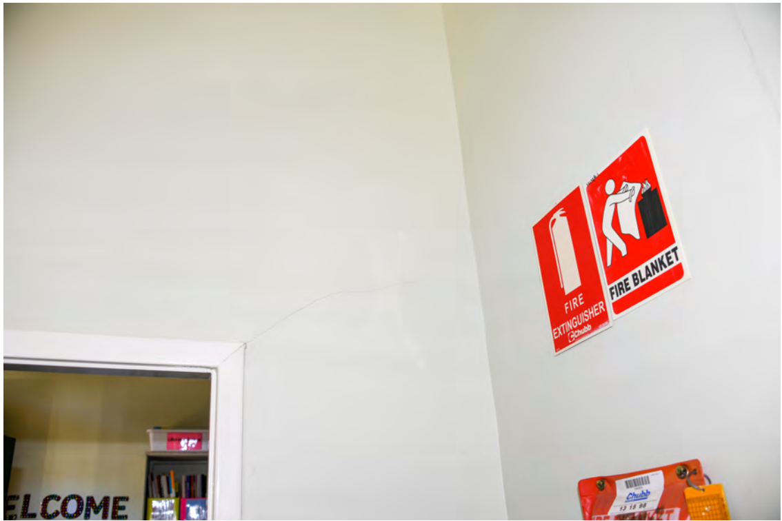
Block H. Interior. Eastern end. Foyer. Eastern face. Crack stemming out from the doorway.
