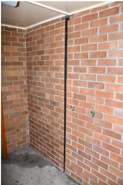
Block F. Southern elevation. Eastern end. Control joint in the brickwork.
