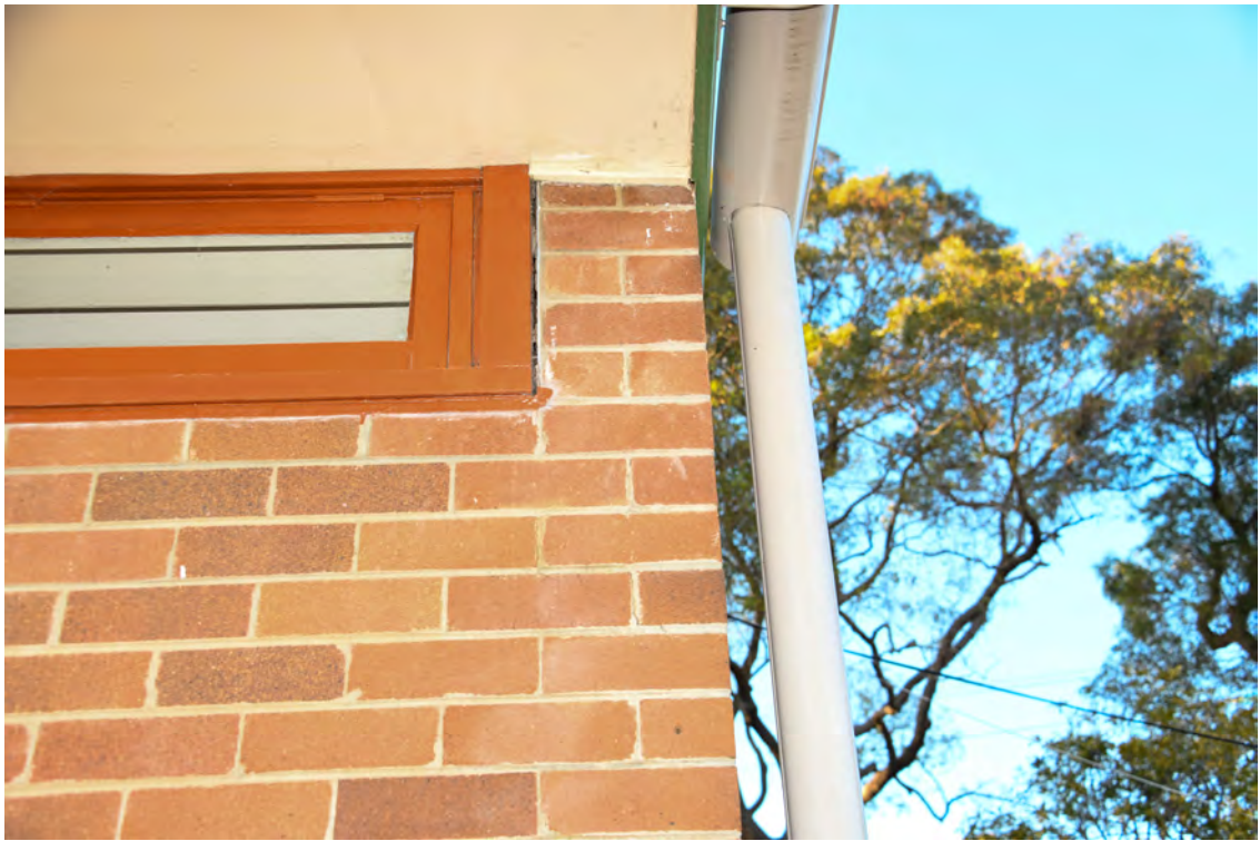
Block H. Northern elevation. Heading east. Gap between the brickwork and the window framing.
