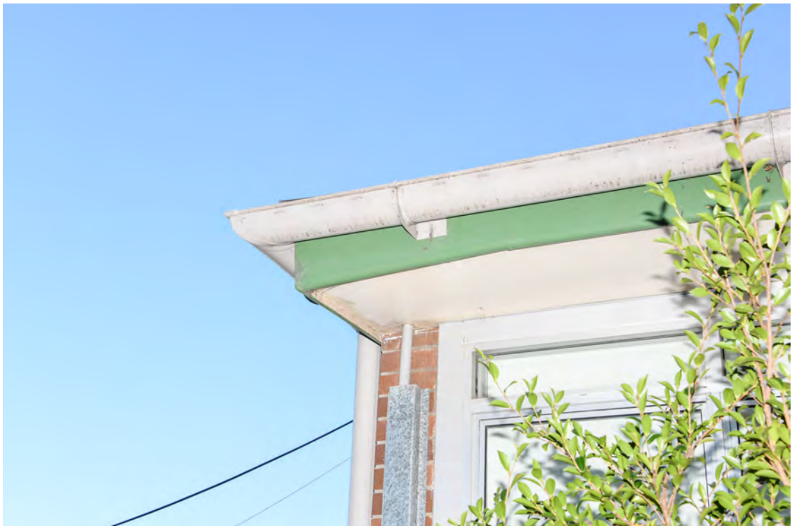
Block H. Southern elevation fronting Carlingford Road. Western end. Sagging of the fascia board and eaves.
