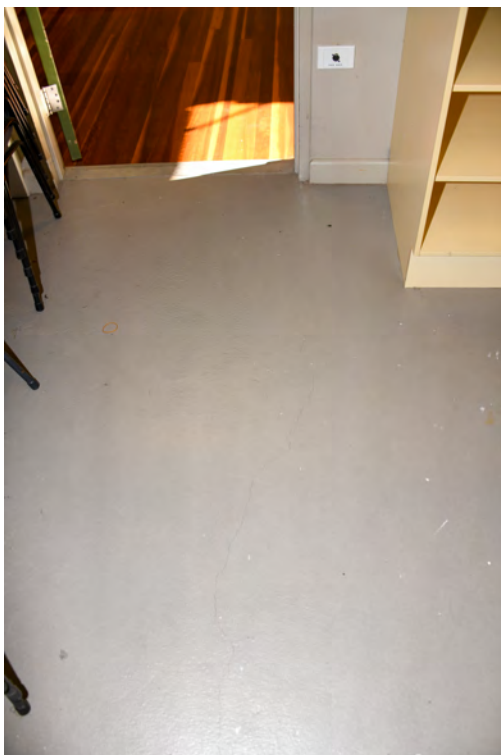
Block M / Hall / The Aurora Centre. Interior. Southern face. Boys Change Room. Flooring. Cracked flooring.
