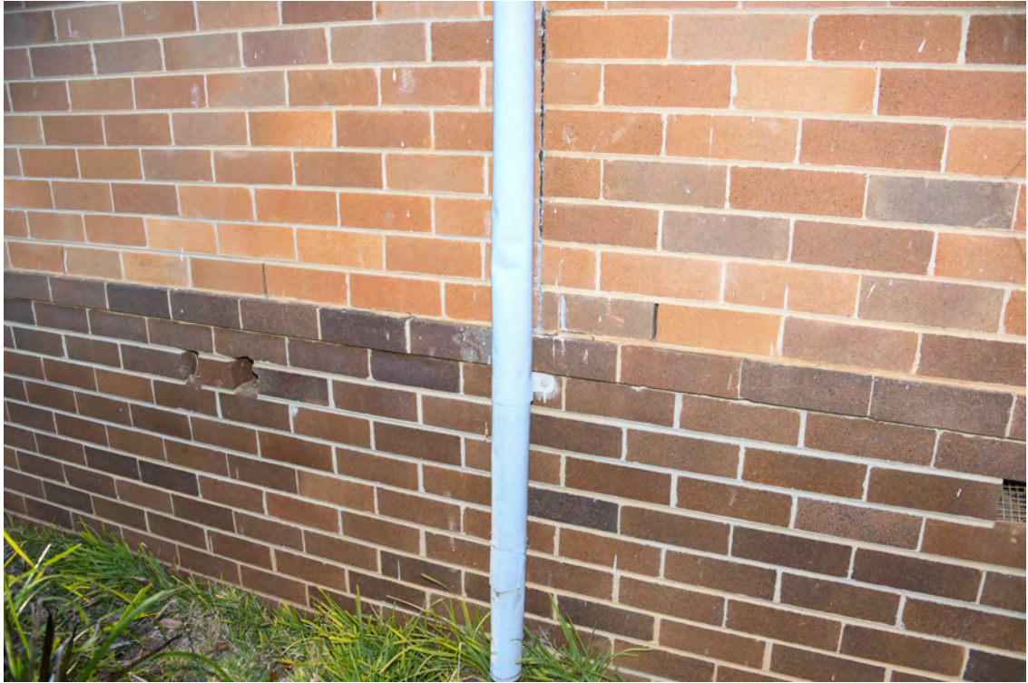
Block F. Northern elevation. Heading west. Chipped brick edges at the wall vent.
