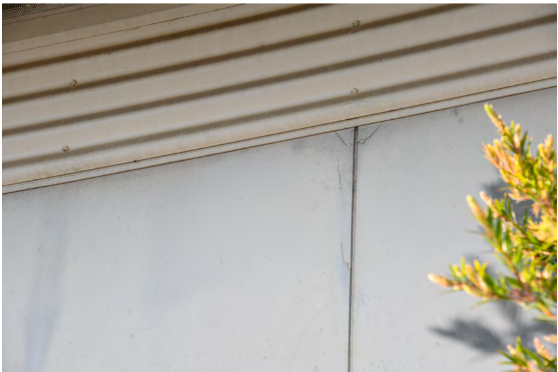
Block I. Northern elevation. Cracked wall cladding.
