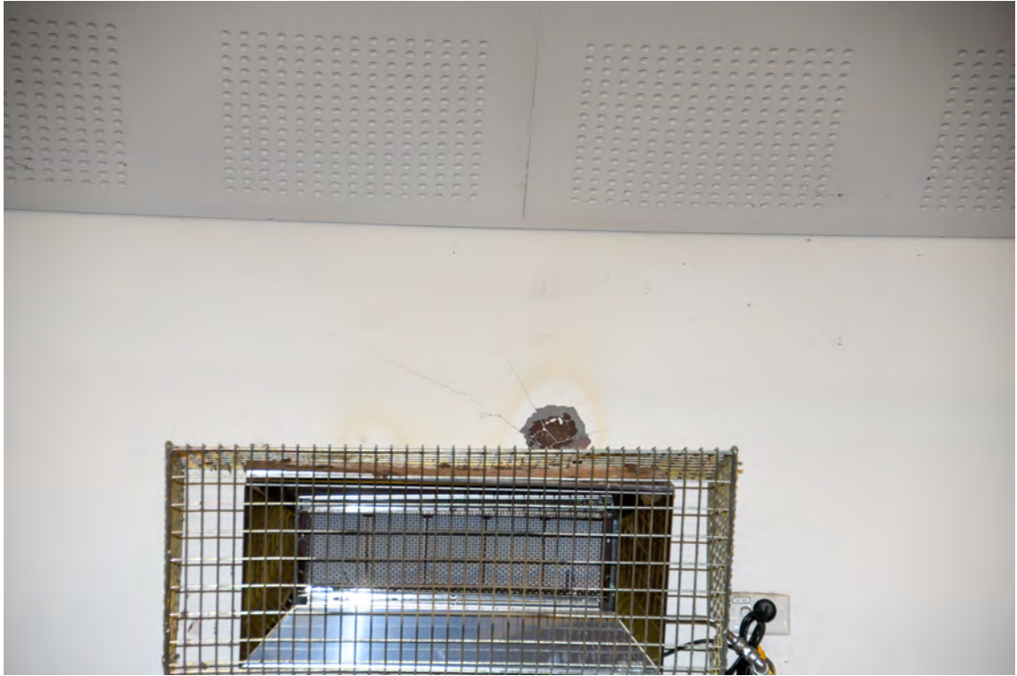
Block M / Hall / The Aurora Centre. Interior. Northern face. Damaged wall above the heater.
