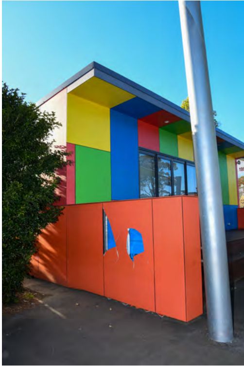
Block R. Northern elevation. Western end. Damaged cladding.
