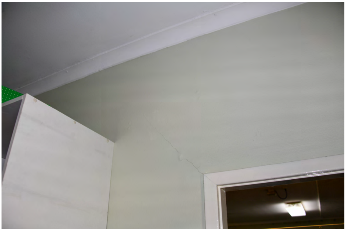
Block F. Interior. Foyer. Western face. Cracked cladding stemming out from the doorway.
