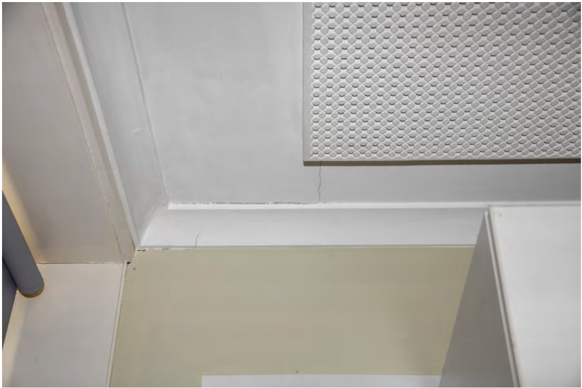
Block F. Interior. Room KA. North-eastern corner of the ceiling. Cracked ceiling.
