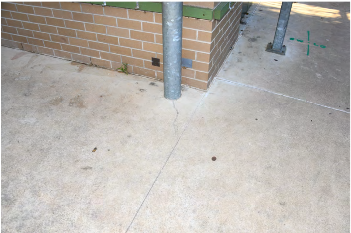
Block M / Hall / The Aurora Centre. Southern elevation. Eastern end. Cracked paving.
