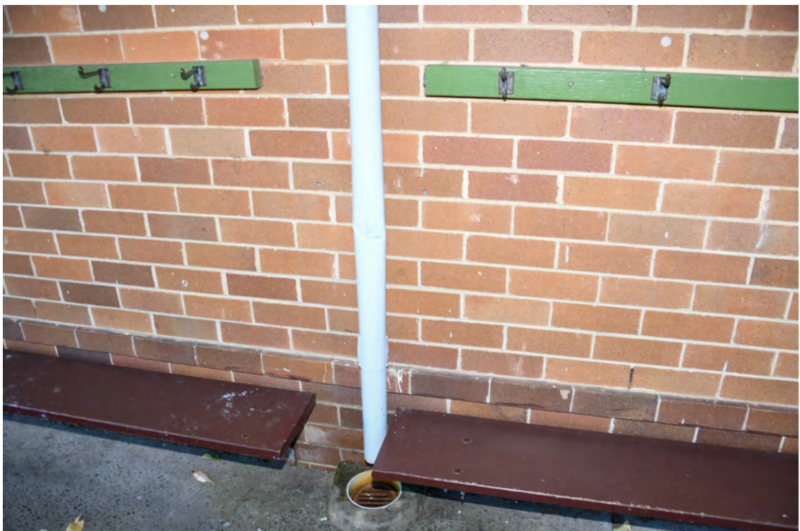
Block F. Southern elevation. Heading west. Indentation in the down pipe.
