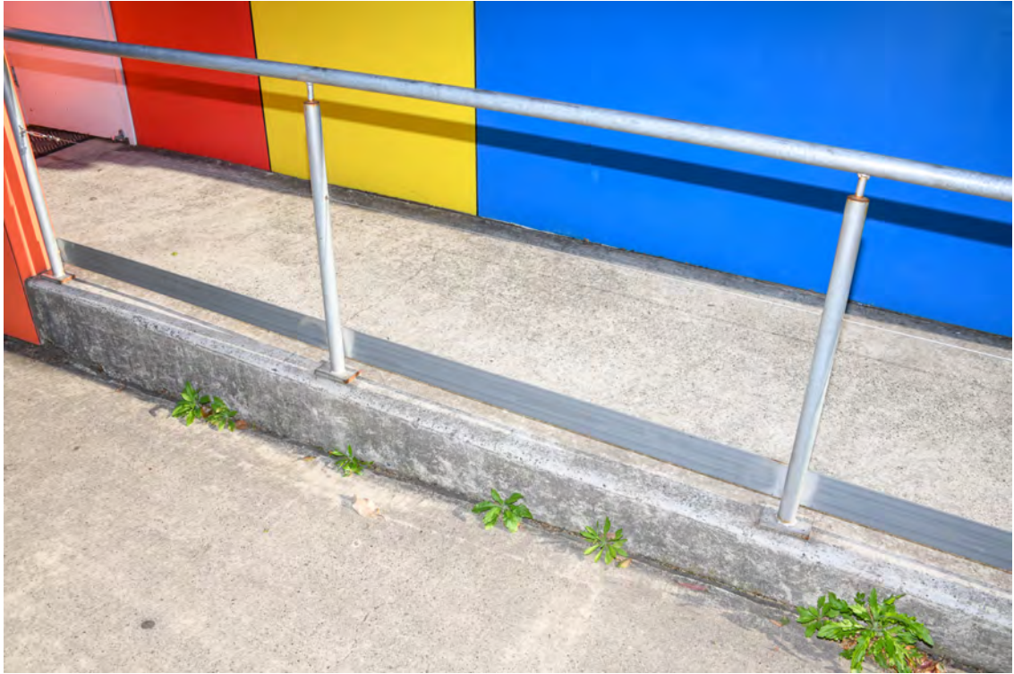
Block R. Southern side. Cracked adjacent paving.
