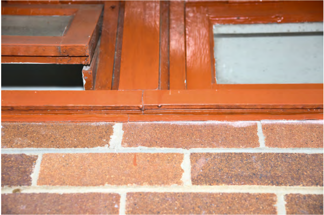
Block H. Northern elevation. Heading east. Movement in window framing.
