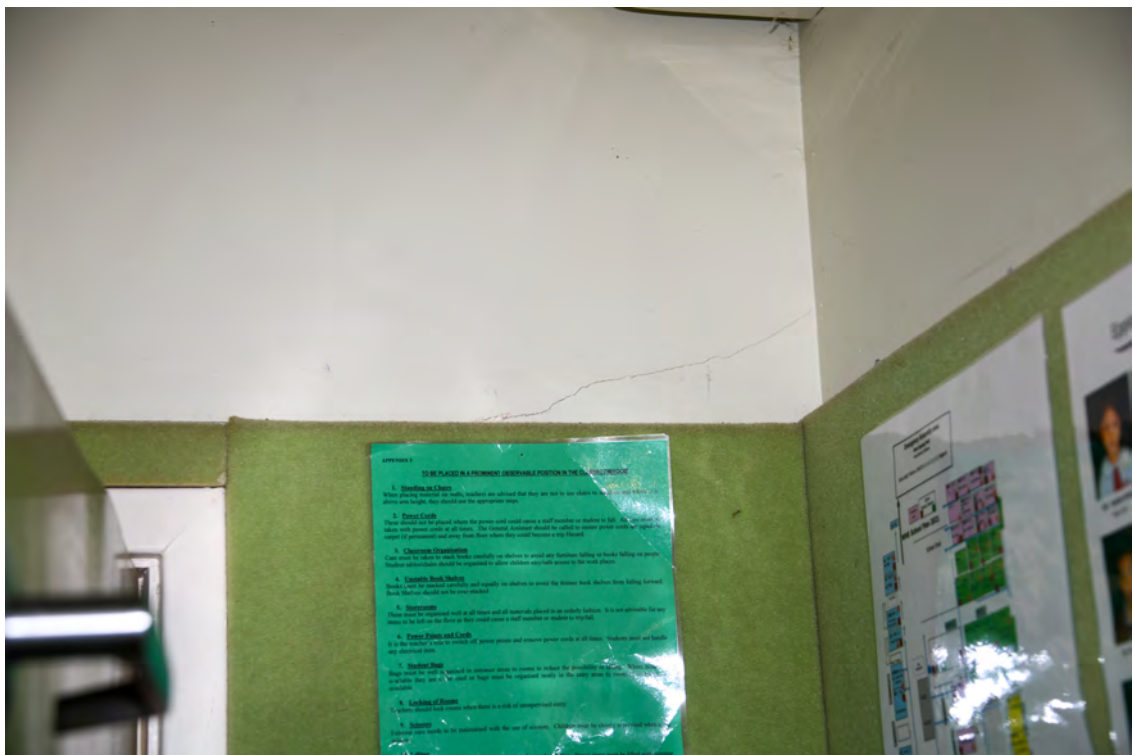
Block H. Interior. Room HR0031. North-eastern corner. Cracked wall.
