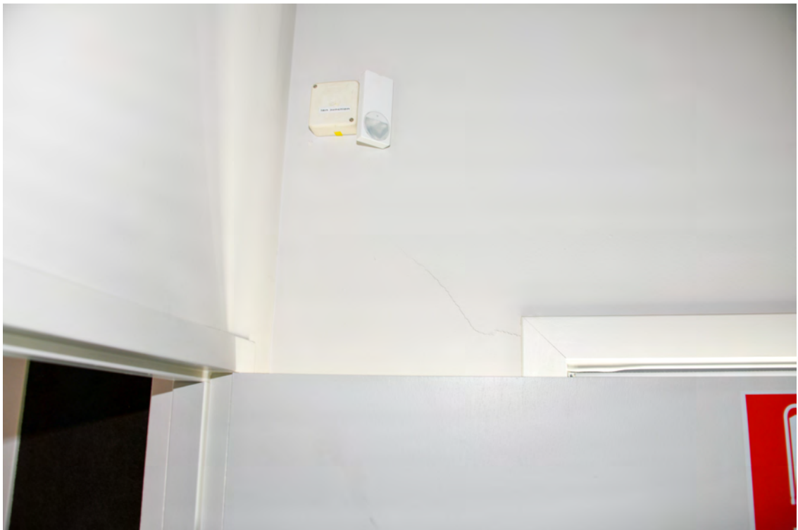
Block R. Interior. Western half. Western face. Crack in the wall lining.
