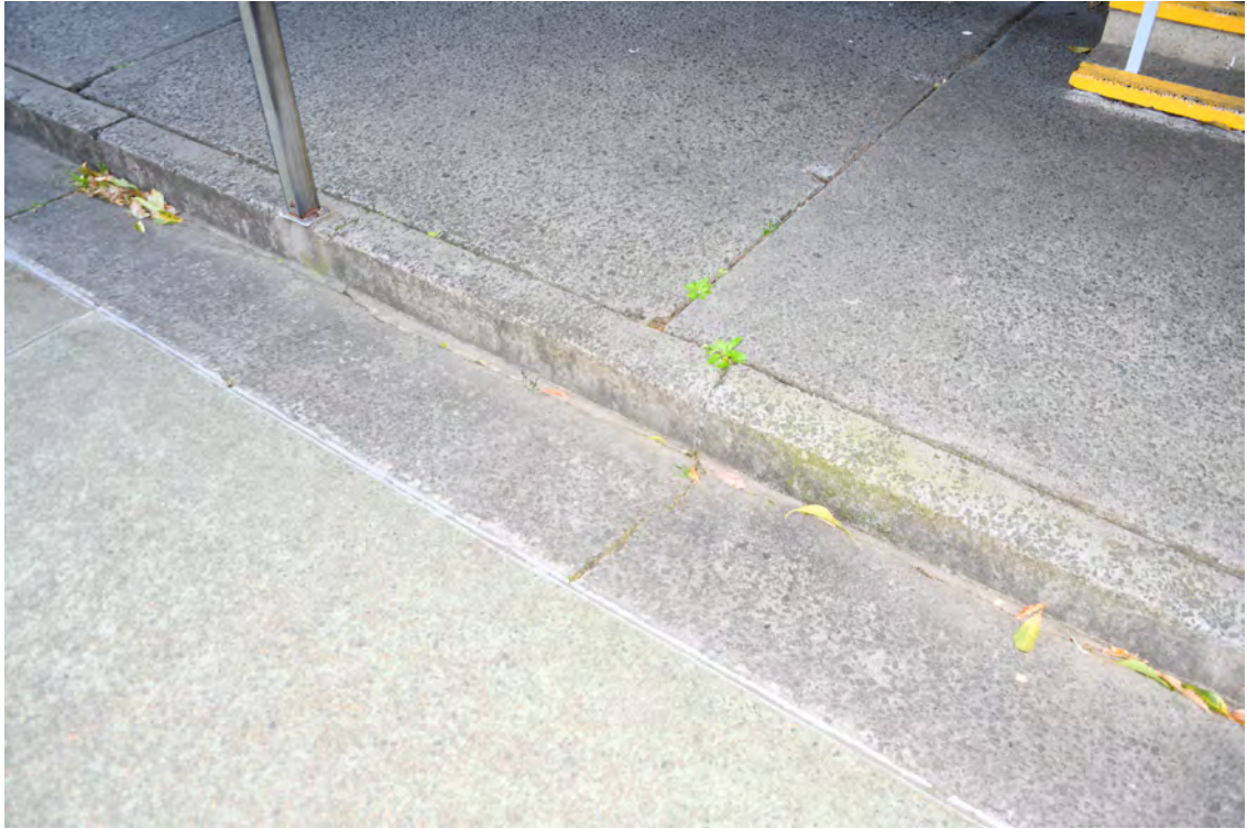
Block F. Southern elevation. Western end. Cracked kerb and gutter.
