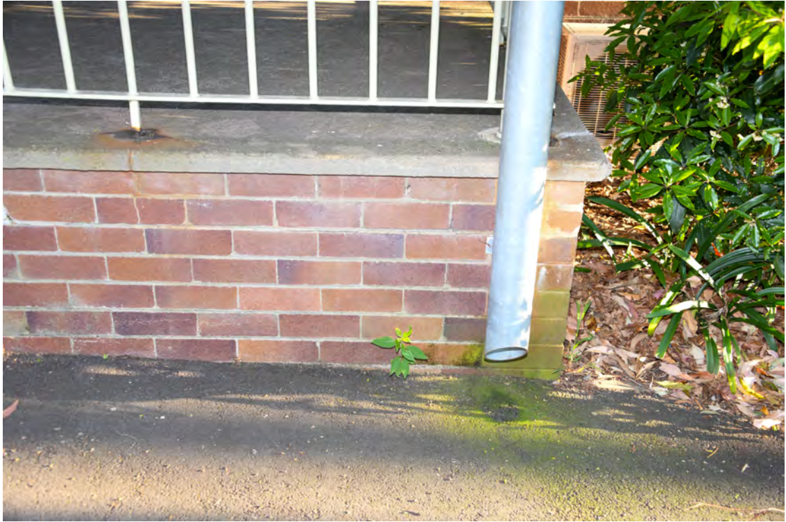
Block H. Southern elevation fronting Carlingford Road. Heading west. Eastern building entry. Cracked mortar beds.
