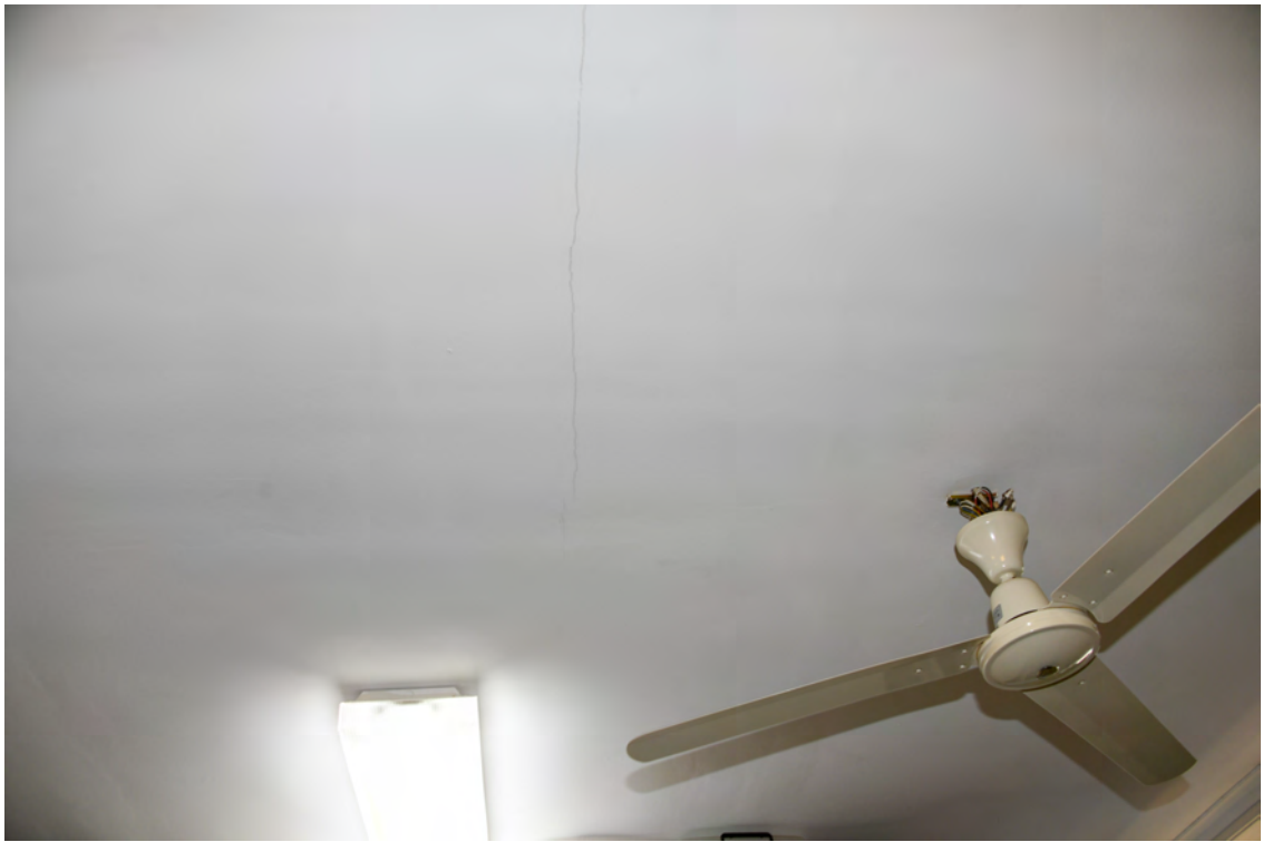
Block F. Interior. Eastern room. Cracked ceiling.
