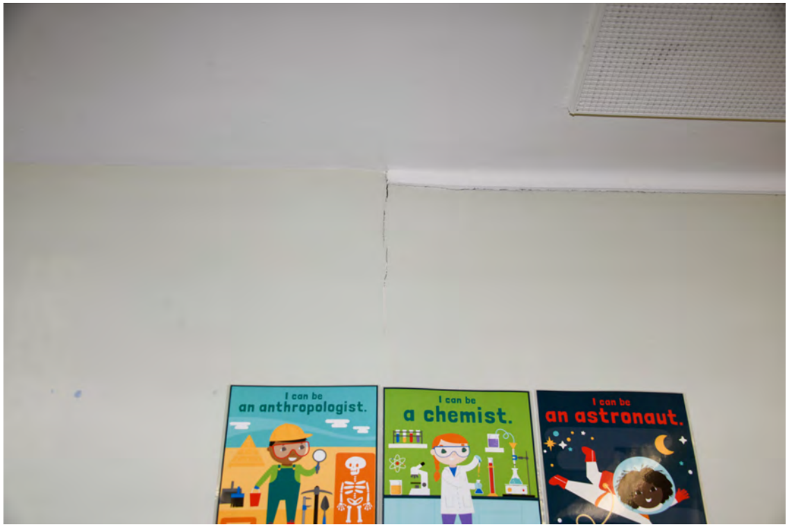
Block H. Interior. Room HR0027. Western face. Crack.
