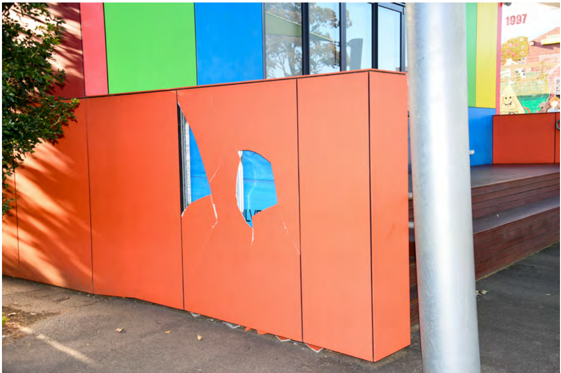
Block R. Northern elevation. Western end. Damaged cladding.
