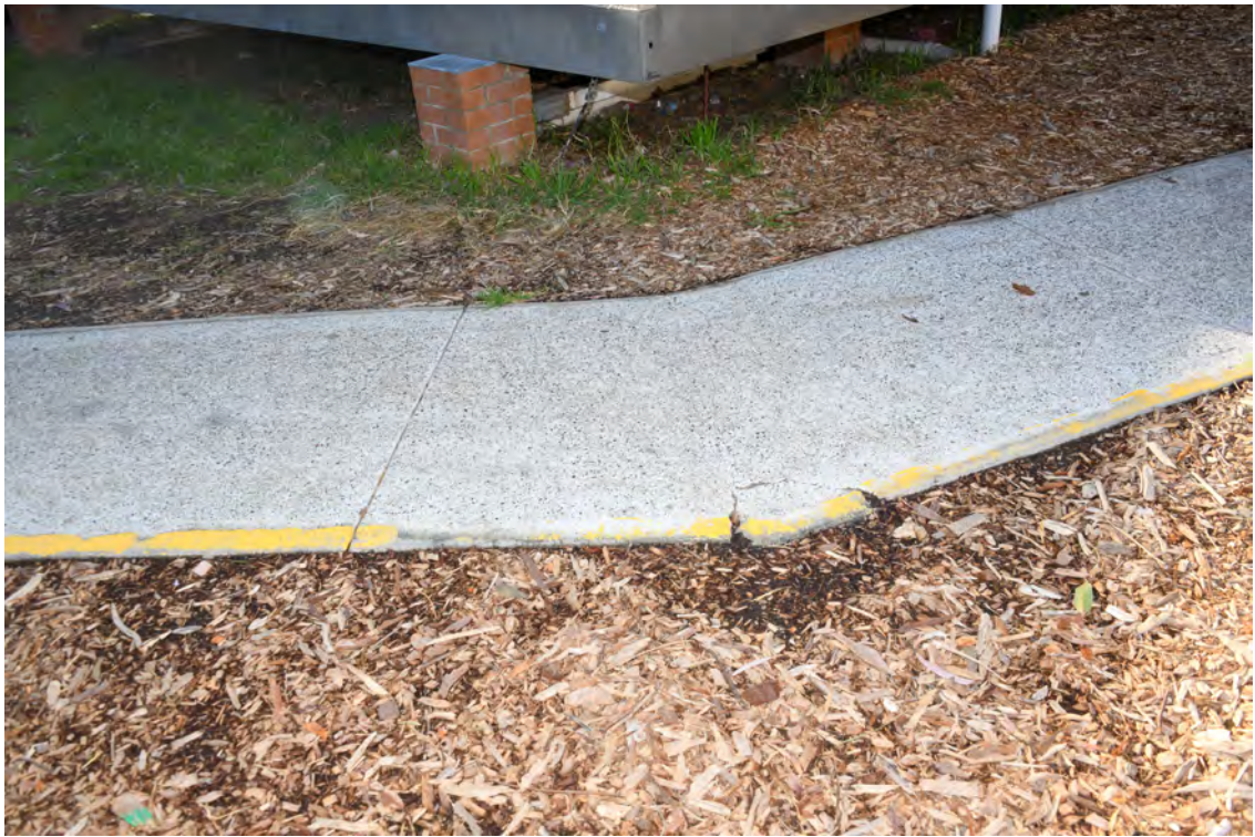
Amenities on the northern side of Block M / Hall / The Aurora Centre. Area on the eastern side of the block. Damaged paving.
