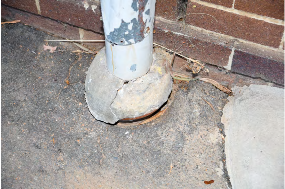
Block H. Northern elevation. Eastern end. Cracked surround to the base of the downpipe.
