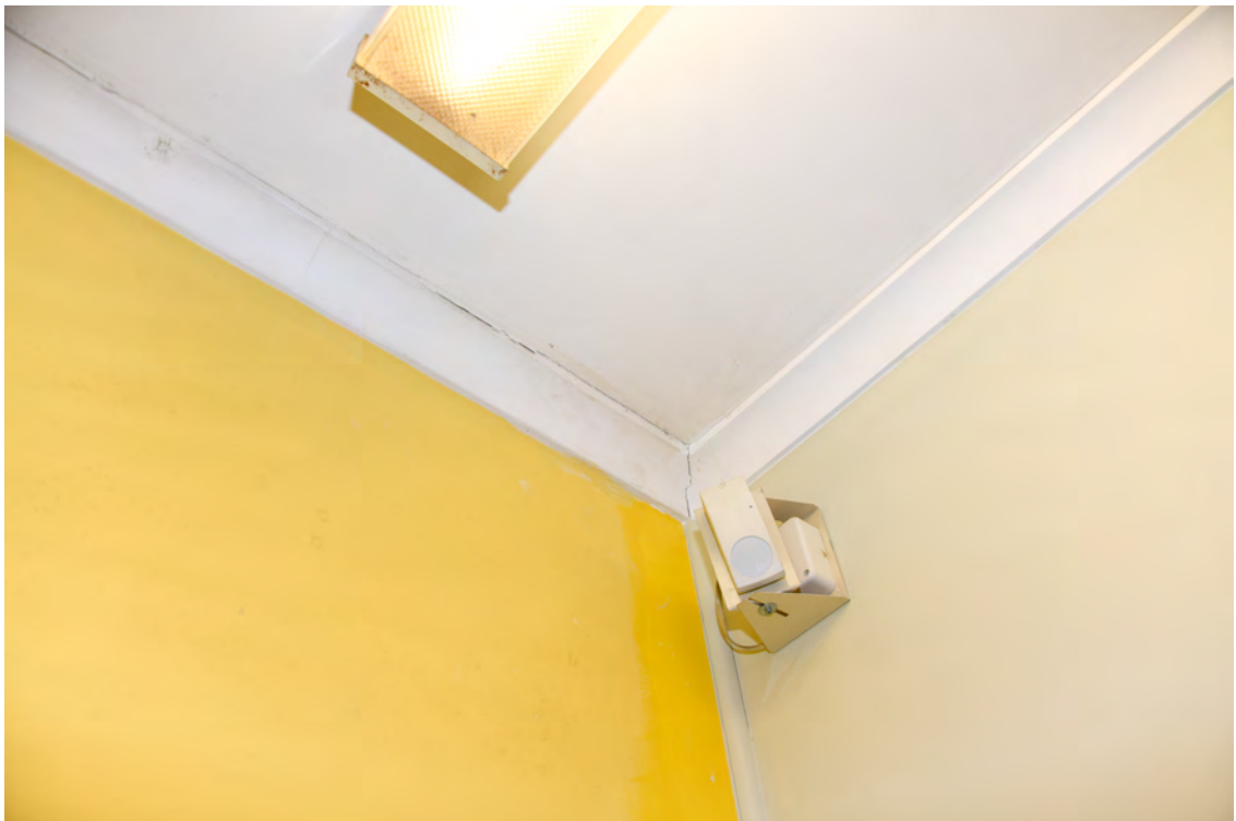
Block F. Interior. Entry Foyer (room 14). Northern face. Movement to the cornice.
