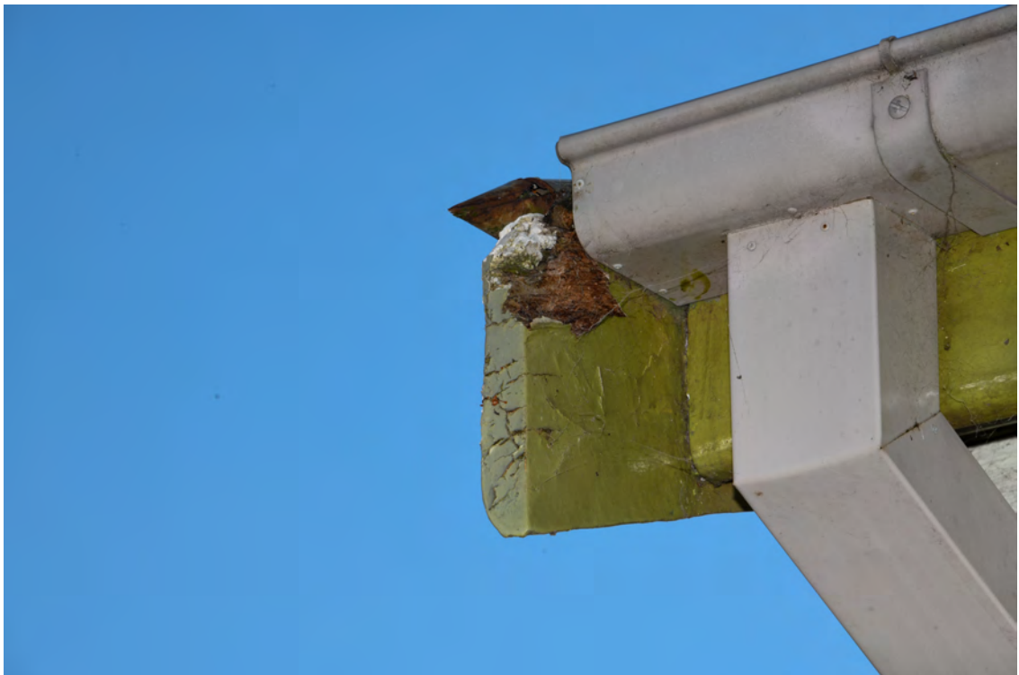
Block D. Western elevation. Northern end. Rotten fascia.
