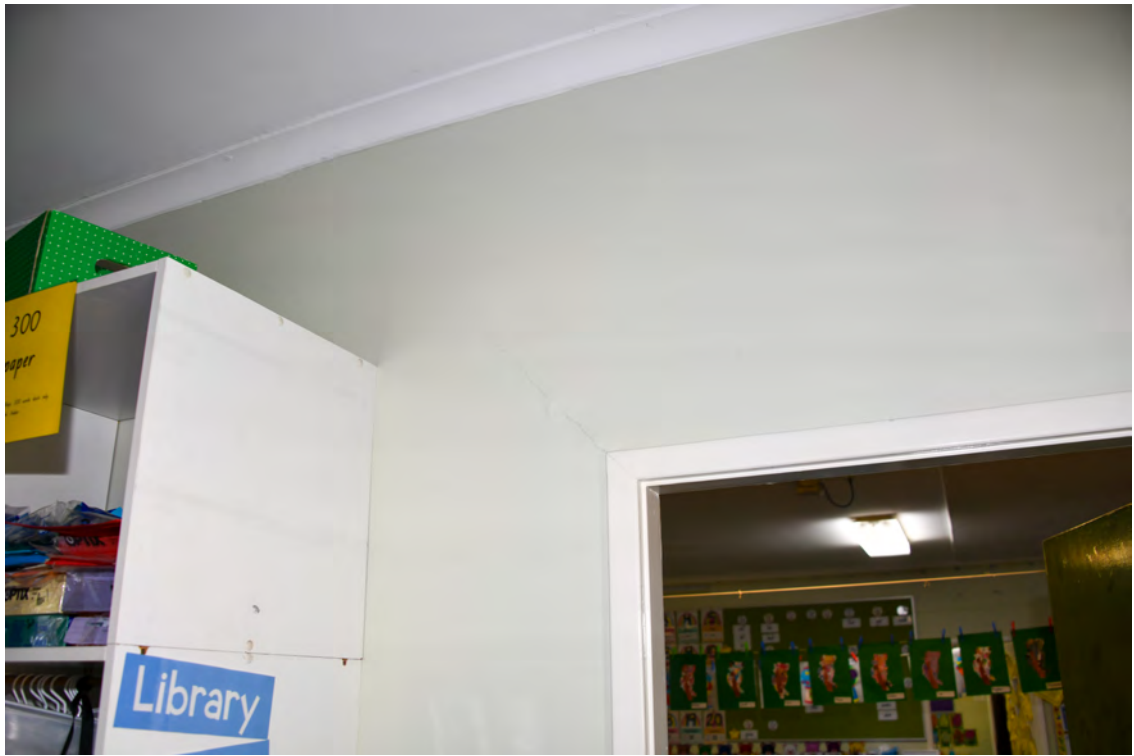
Block F. Interior. Foyer. Eastern face. Cracked wall cladding stemming out from the doorway.
