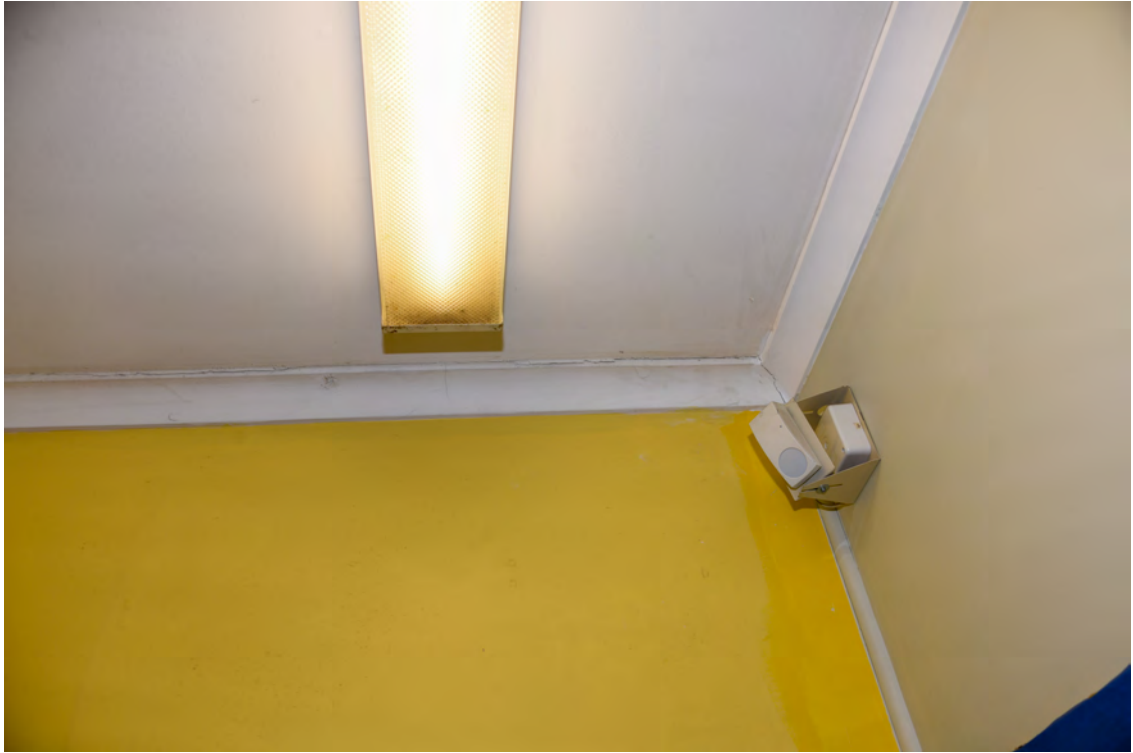
Block F. Interior. Entry Foyer (room 14). Western face. Movement to the cornice.
