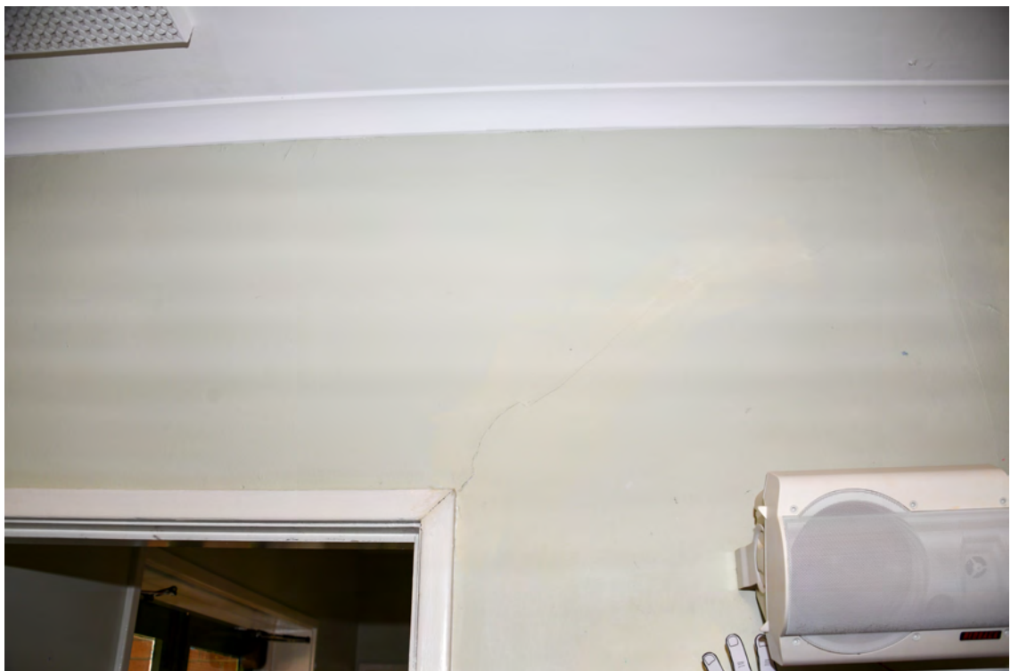
Block F. Interior. Room KG. Western face. Cracked cladding stemming out from the doorway.
