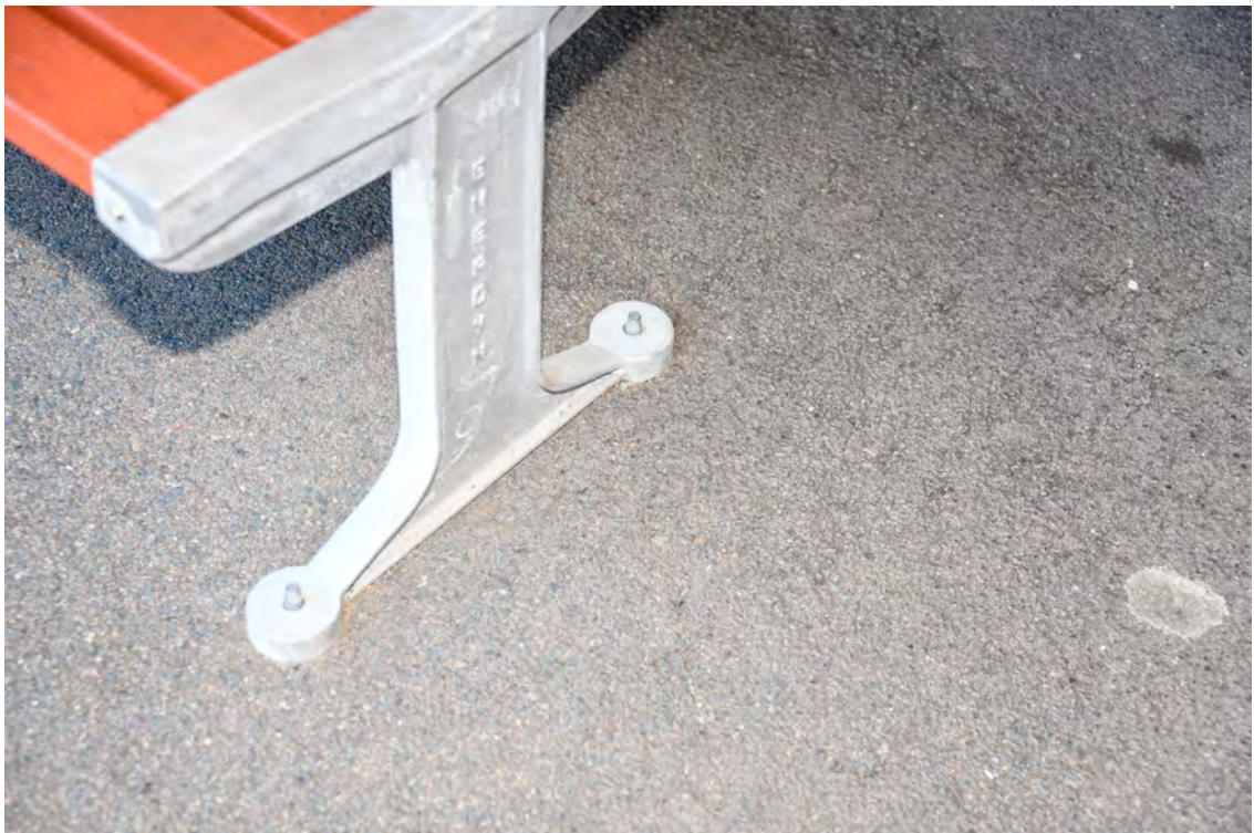
Block A. Western elevation. Heading south. Seats missing fixing nuts.
