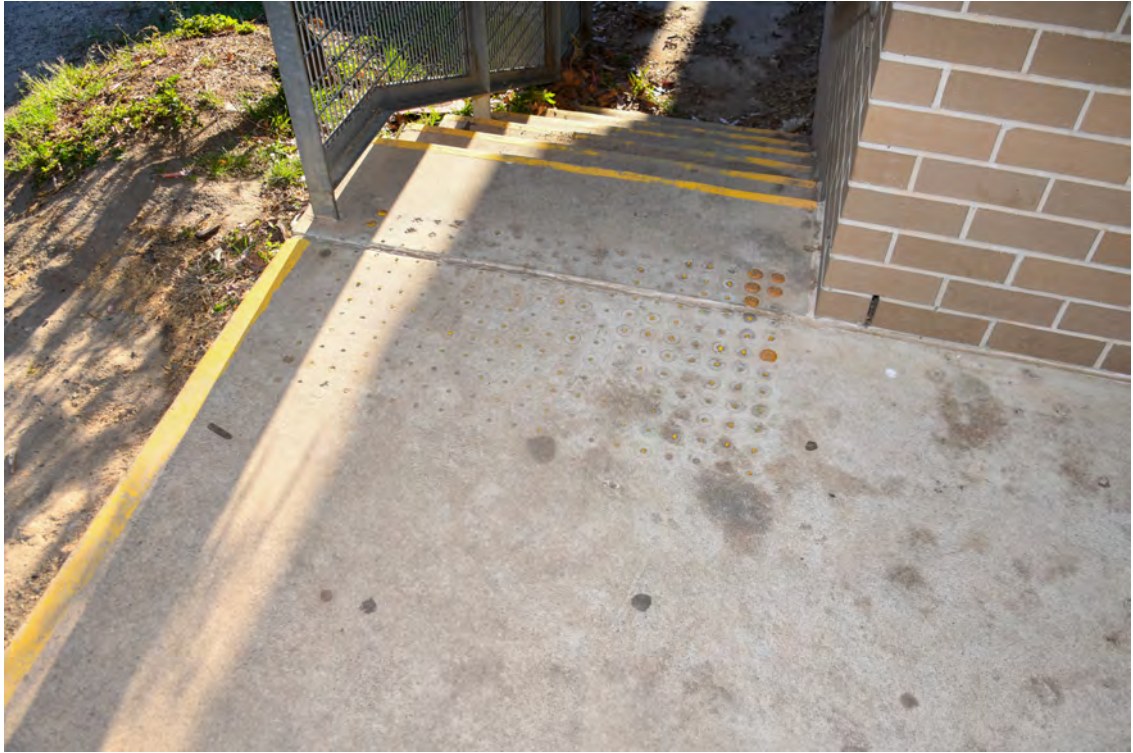
Block M / Hall / The Aurora Centre. Western elevation. COLA. Northern end. Dislodged 'tactiles'.
