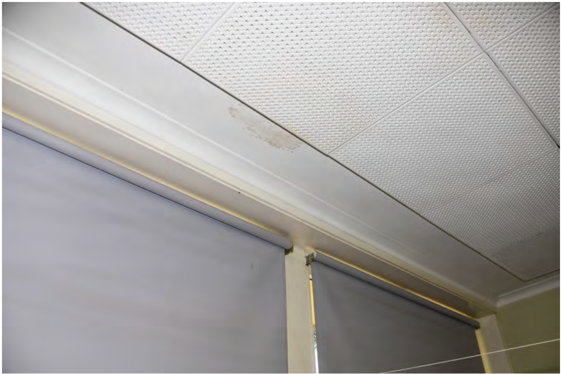
Block F. Interior. Room KH. Northern face. Stain on the ceiling.
