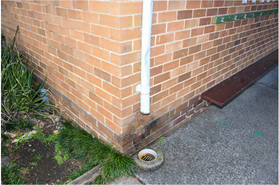
Block F. South-western corner. Indentation in the down pipe.
