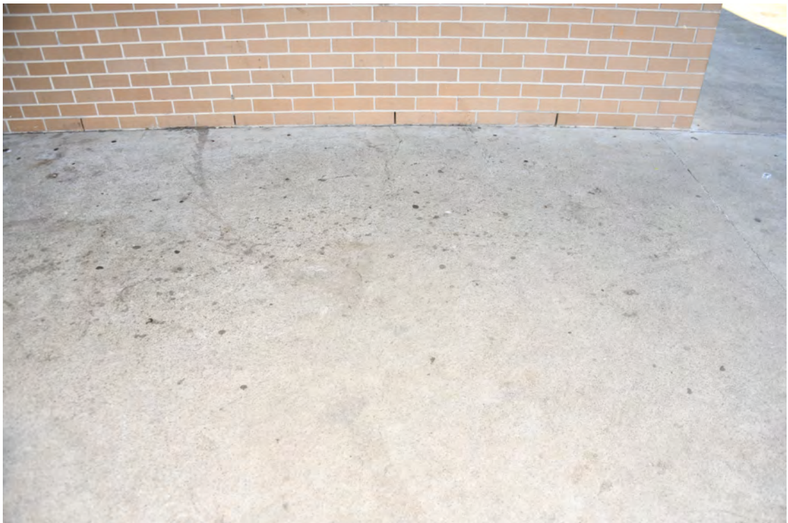
Block M / Hall / The Aurora Centre. Western elevation. COLA. Cracked paving.
