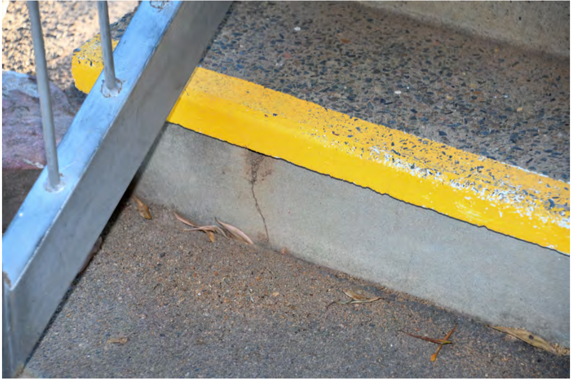
Block H. Northern elevation. Eastern entry. Cracked rendered finish to the stair tread.
