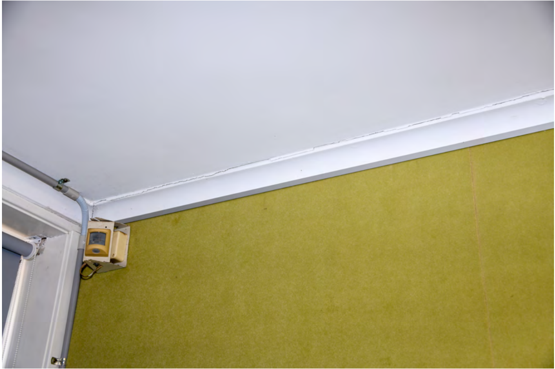
Block F. Interior. Eastern room. Eastern face. Movement to the cornice.
