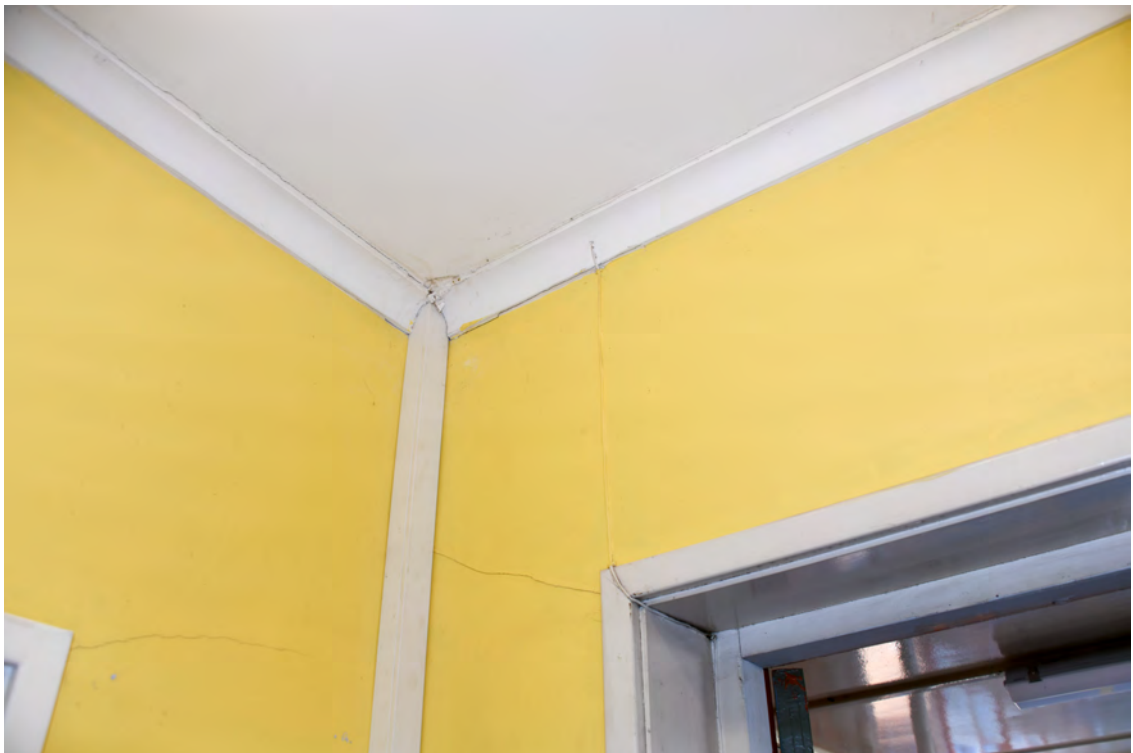
Block F. Interior. Entry Foyer (room 14). Southern face. Cracked wall cladding and movement to the cornice.
