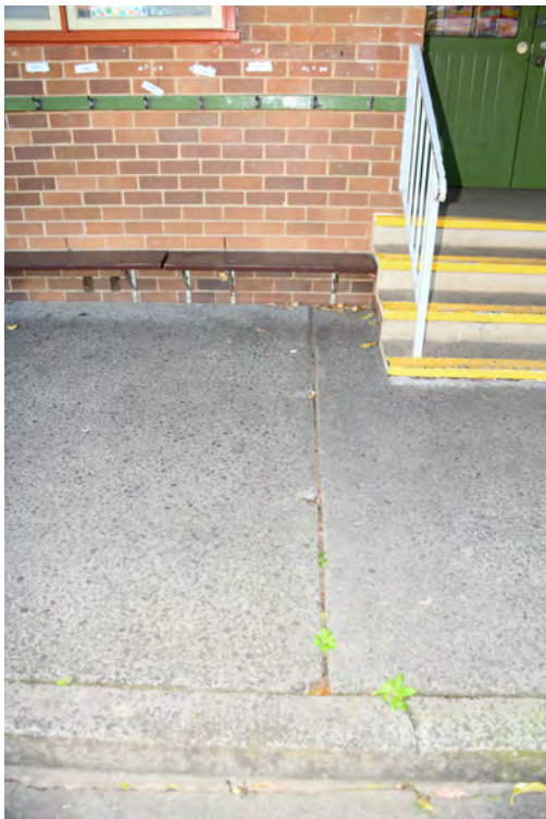
Block F. Southern elevation. Western end. Chipped concrete paving.
