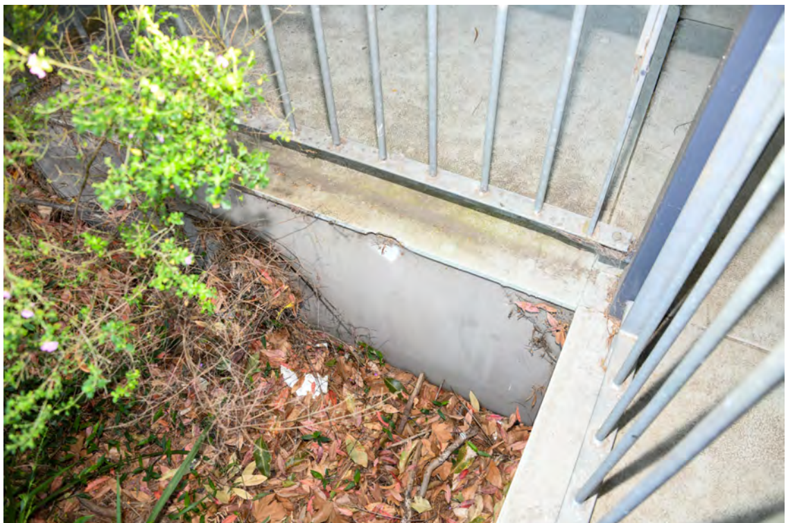
Block I. Southern elevation. Eastern end. Chipped edge of the flooring.
