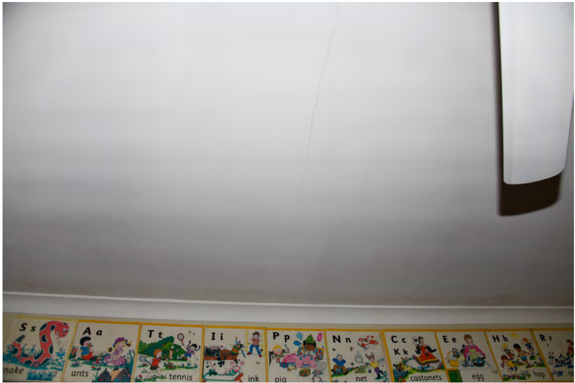
Block F. Interior. Room KA. Eastern side of the ceiling. Cracked ceiling.
