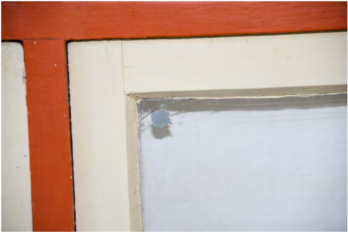
Block H. Northern elevation. Western end. Cracked glazing.
