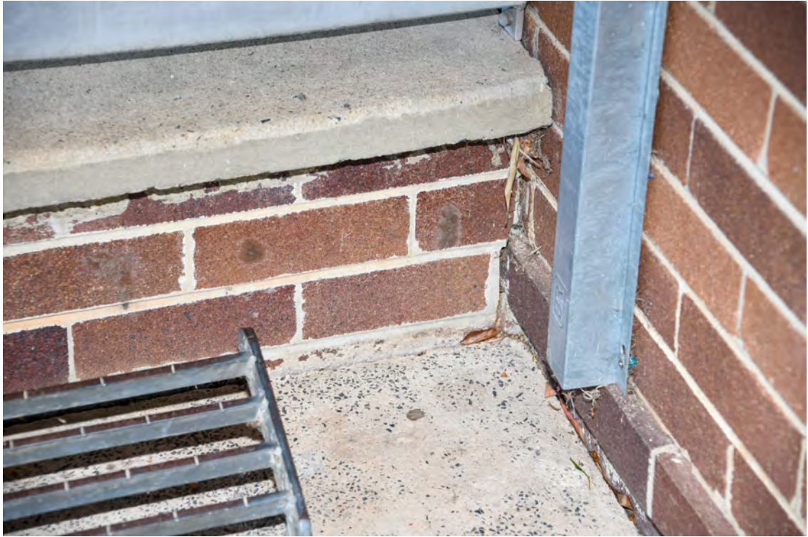
Block H. Northern elevation. Eastern entry. Movement to the brickwork.
