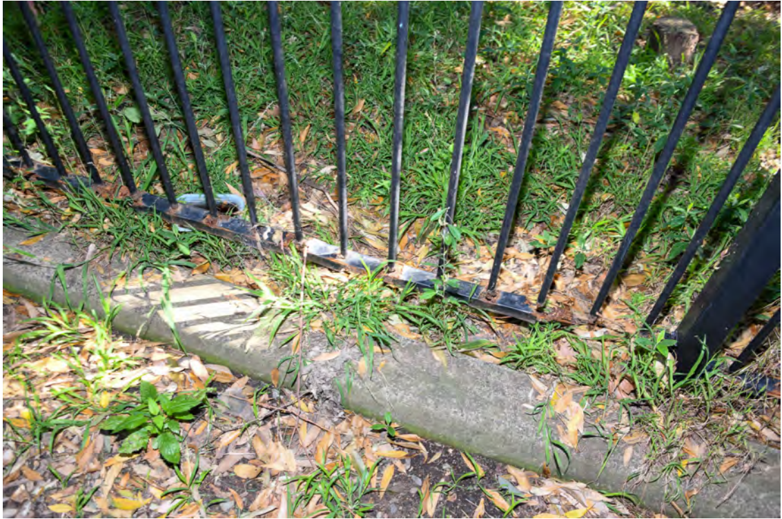
School boundaries. Northern boundary common with the YMCA. Heading west. Rusted and damaged boundary fence.
