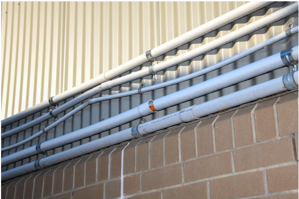
Block M / Hall / The Aurora Centre. Eastern elevation. Heading south. Gap in the electrical conduit.
