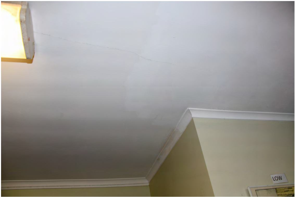
Block F. Interior. Eastern room. Cracked ceiling.
