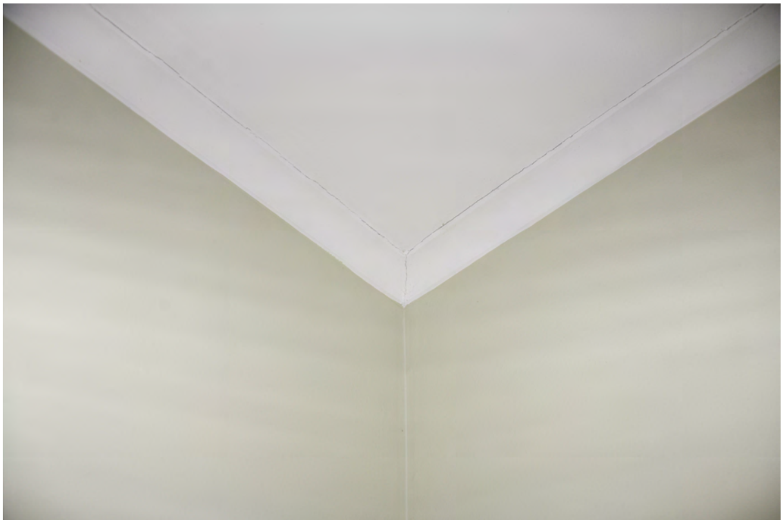
Block F. Interior. Foyer. Western face. Movement to the cornice.
