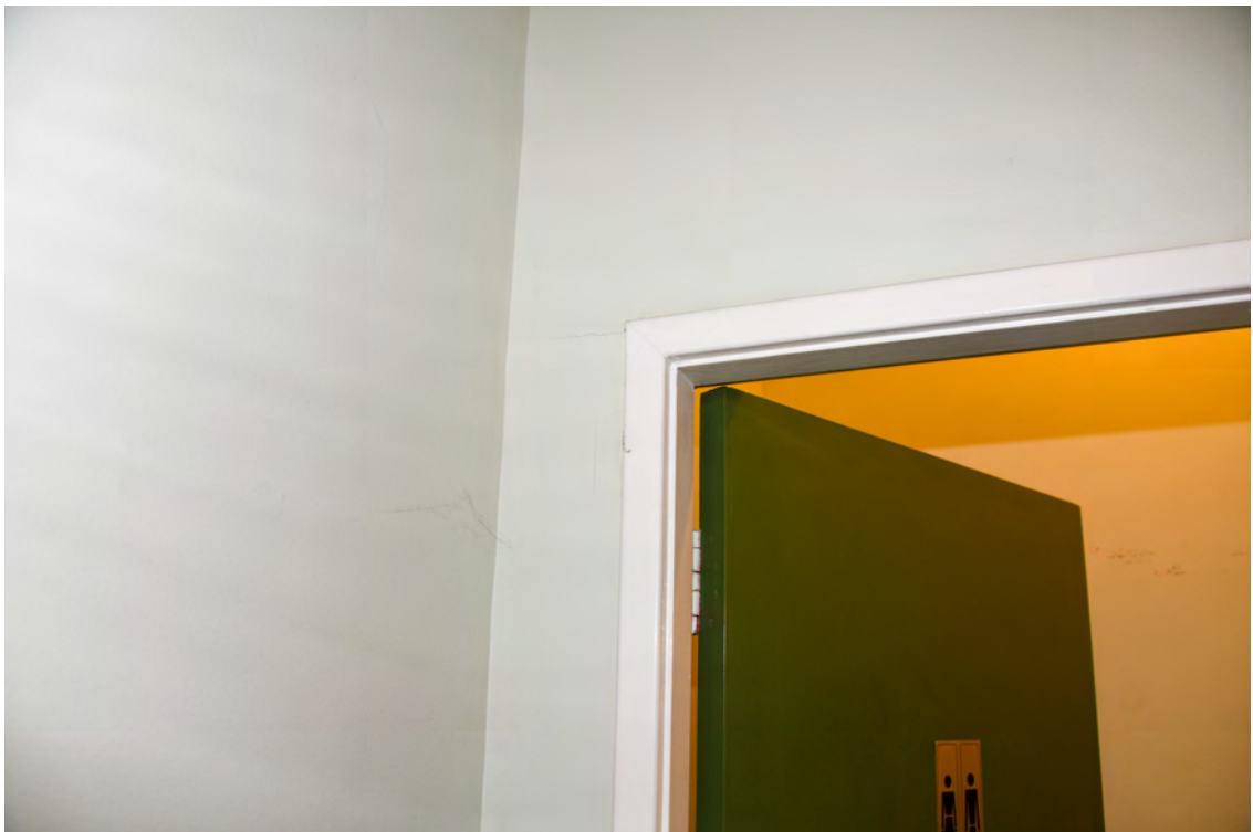
Block H. Interior. Eastern end. Foyer. Western face. Cracked cladding stemming out from the doorway.
