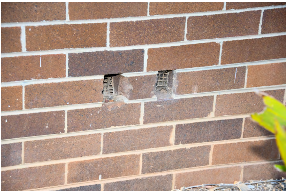
Block F. Northern elevation. Eastern end. Chipped brick edges at the wall vent.
