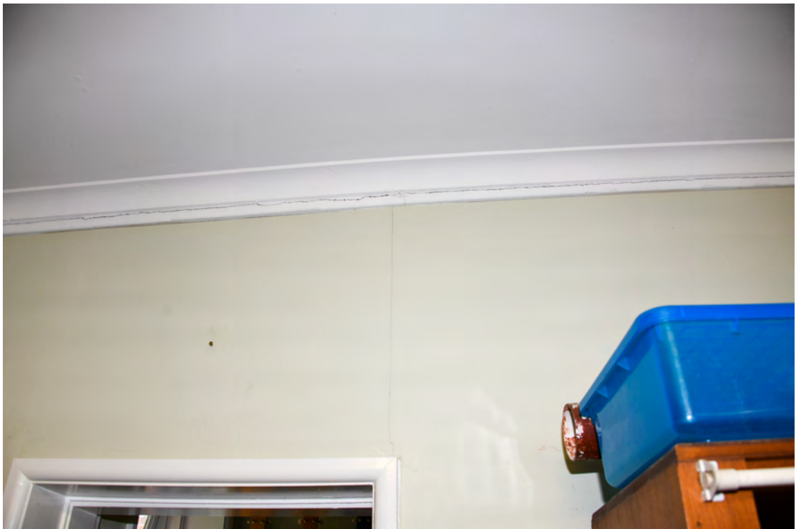
Block F. Interior. Eastern room. Southern face. Movement to the cornice.
