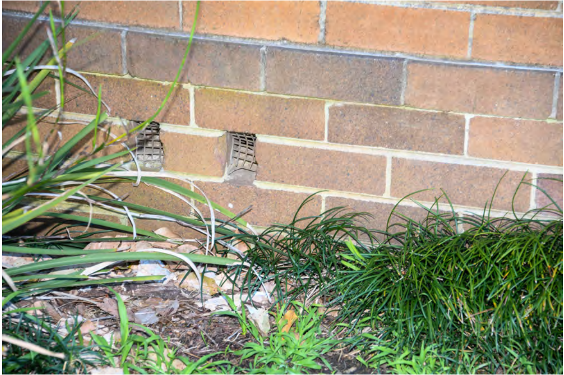
Block F. Western elevation. Southern end. Damaged wall vents.
