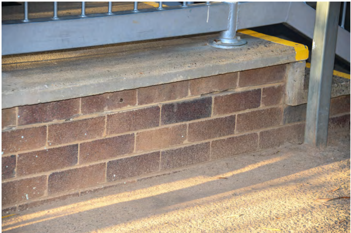
Block H. Northern elevation. Eastern entry. Eroded mortar beds.
