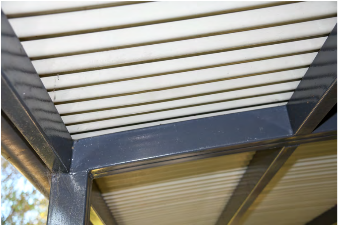
Block I. Southern side of the building. Access ramp. Indentation in the roof sheeting.
