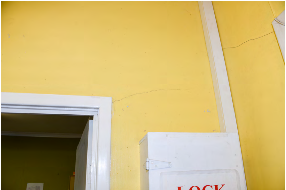
Block F. Interior. Entry Foyer (room 14). Eastern face. Cracked wall cladding.
