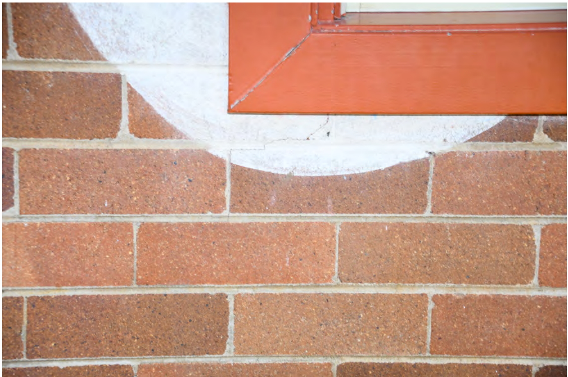
Block H. Northern elevation. Heading east. Cracked mortar bed.
