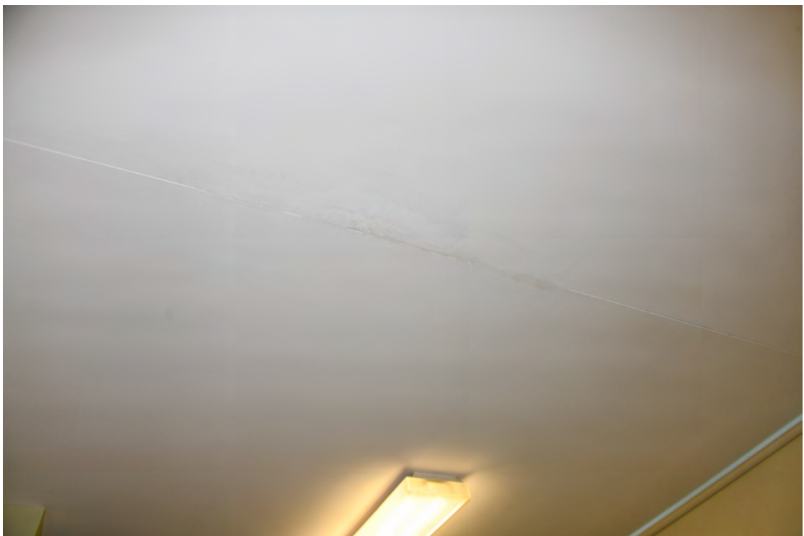
Block I. Eastern room. Ceiling. Water damage.
