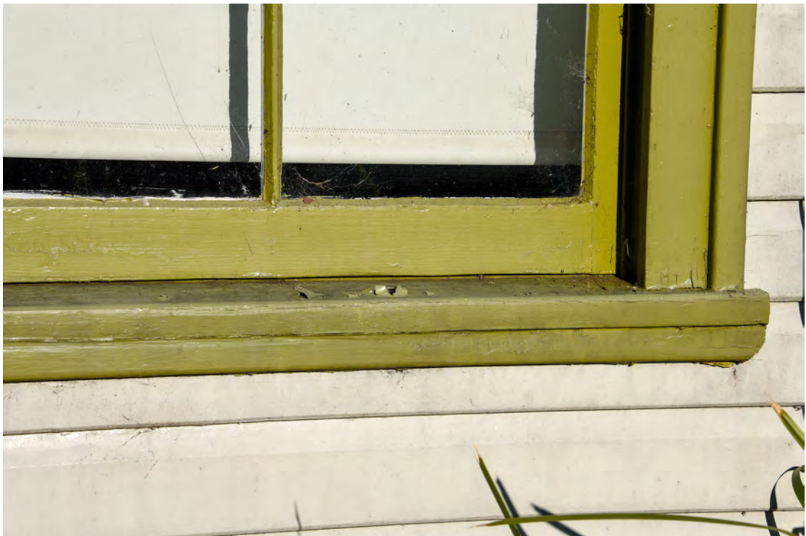
Block D. Eastern elevation. Northern end. Flaking paint finish.
