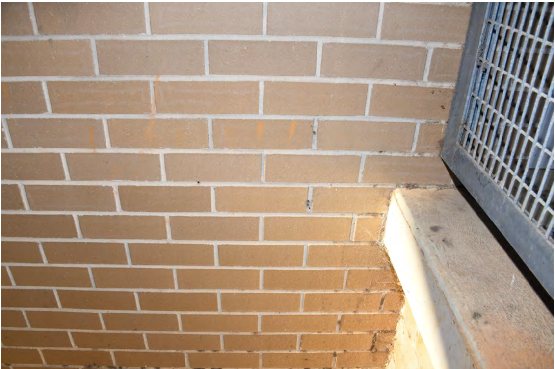
Block M / Hall / The Aurora Centre. Northern elevation. Heading east. Cracked mortar beds.
