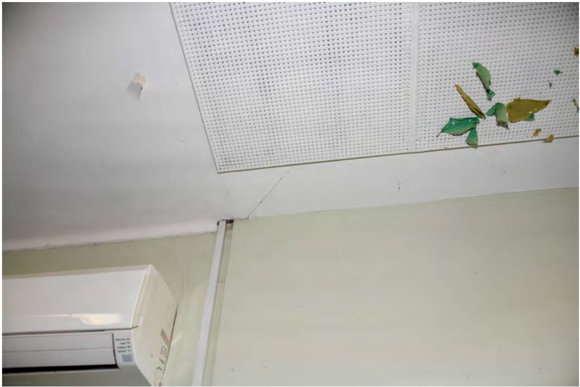
Block H. Interior. Room HR0031. Eastern face. Ceiling. Crack.
