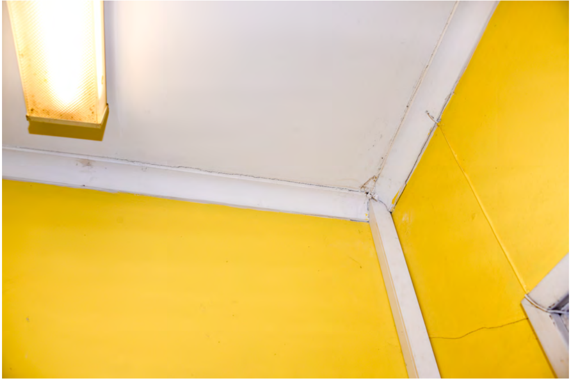
Block F. Interior. Entry Foyer (room 14). Eastern face. Cracked wall cladding and movement to the cornice.
