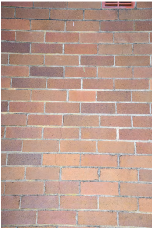
Block F. Western elevation. Cracked brickwork.
