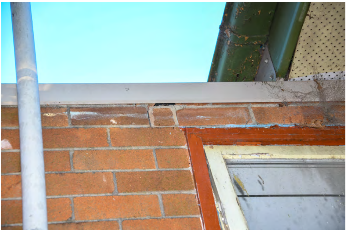
Block F. Eastern elevation. Southern end. Loose brick.
