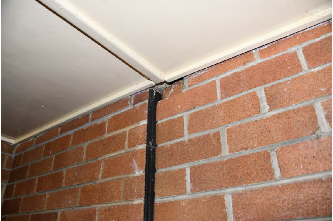
Block F. Southern elevation. Eastern end. Control joint in the brickwork. Loose brick.
