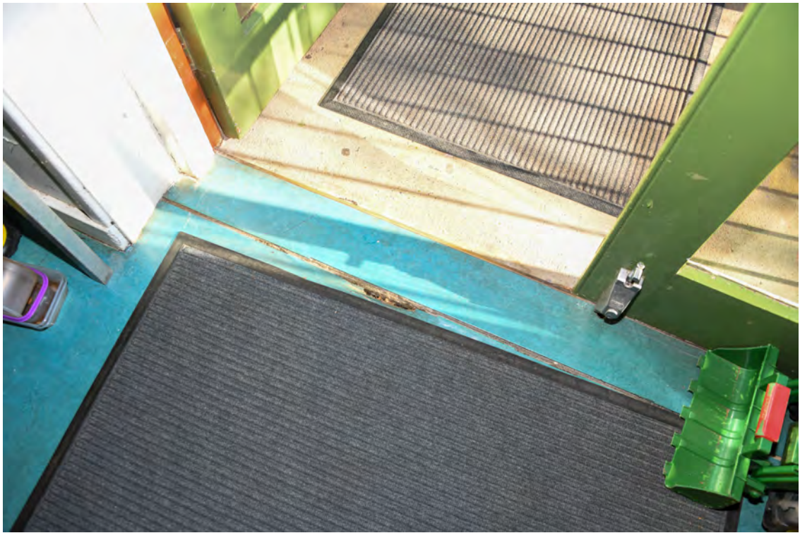
Block H. Interior. Eastern end. Foyer. Northern side of the flooring. Damaged sub flooring.
