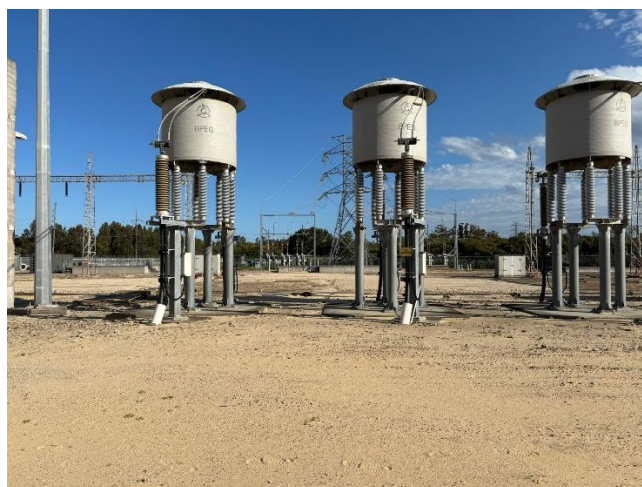
Figure 9 Existing reactors
