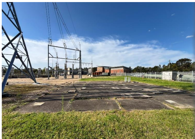
Figure 6 Vacant area within the site
