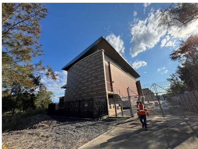
Figure 10 Substation building and northern driveway to Captain Cook Drive
