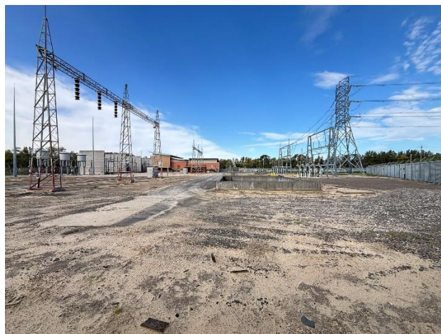
Figure 7 Vacant area within the site
