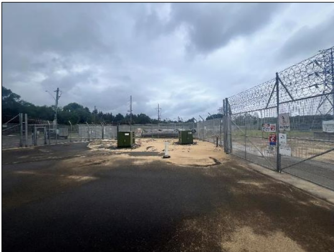
Plate 5: Looking south through the zone substation site.
