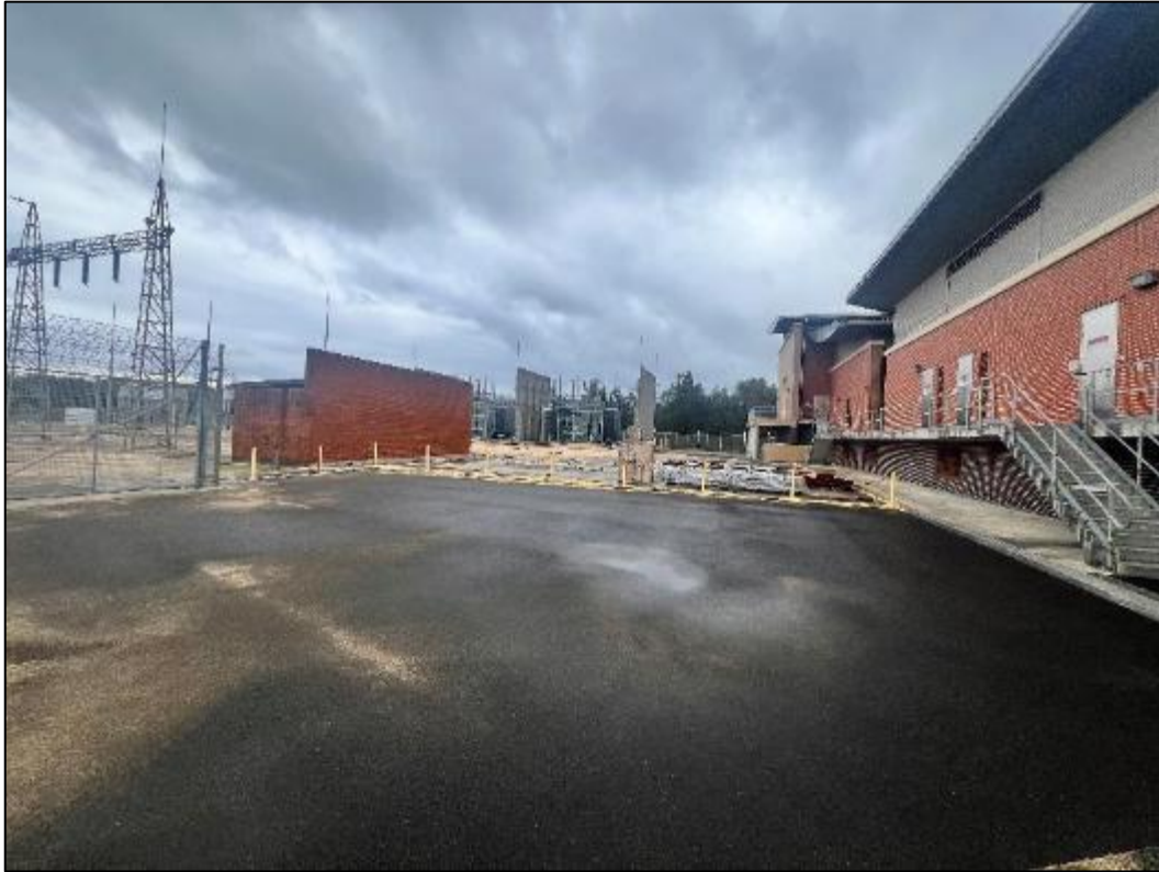
Plate 4: Looking north at area directly west of main Zone Substation building.
