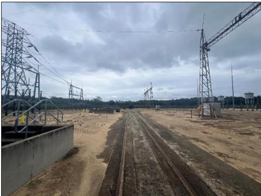
Plate 7: Looking west through the central portion of the site showing significant ground surface disturbance.
