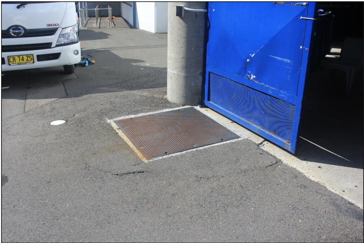
Figure 3.2: Cast iron access plate currently covering shaft 10, looking east.
