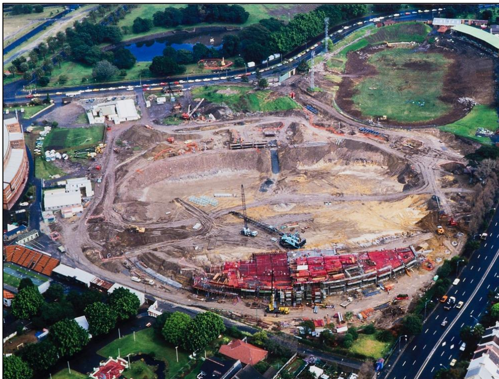
Figure 5.2: Excavation for SFS Construction, 1987, view West (Source: SCG Museum Collection 12/123)
