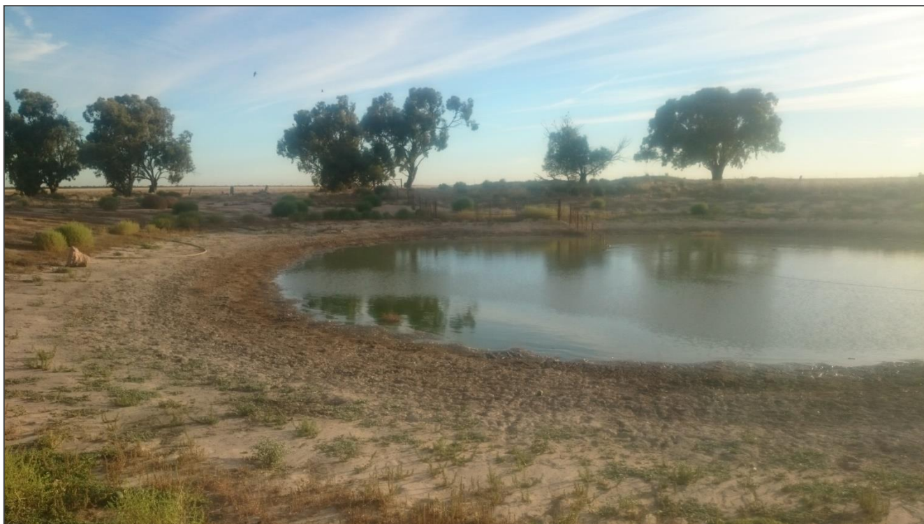
Photo 3 Constructed Dam within the Project Site
