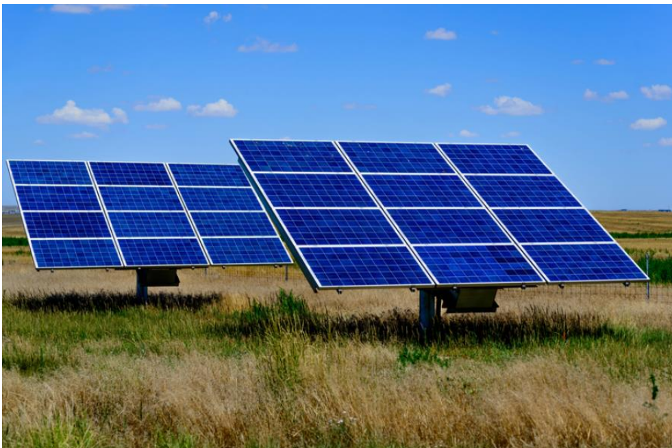
Figure A.10 Long grass, solar panels above flood level, sparse support posts n=0.05
