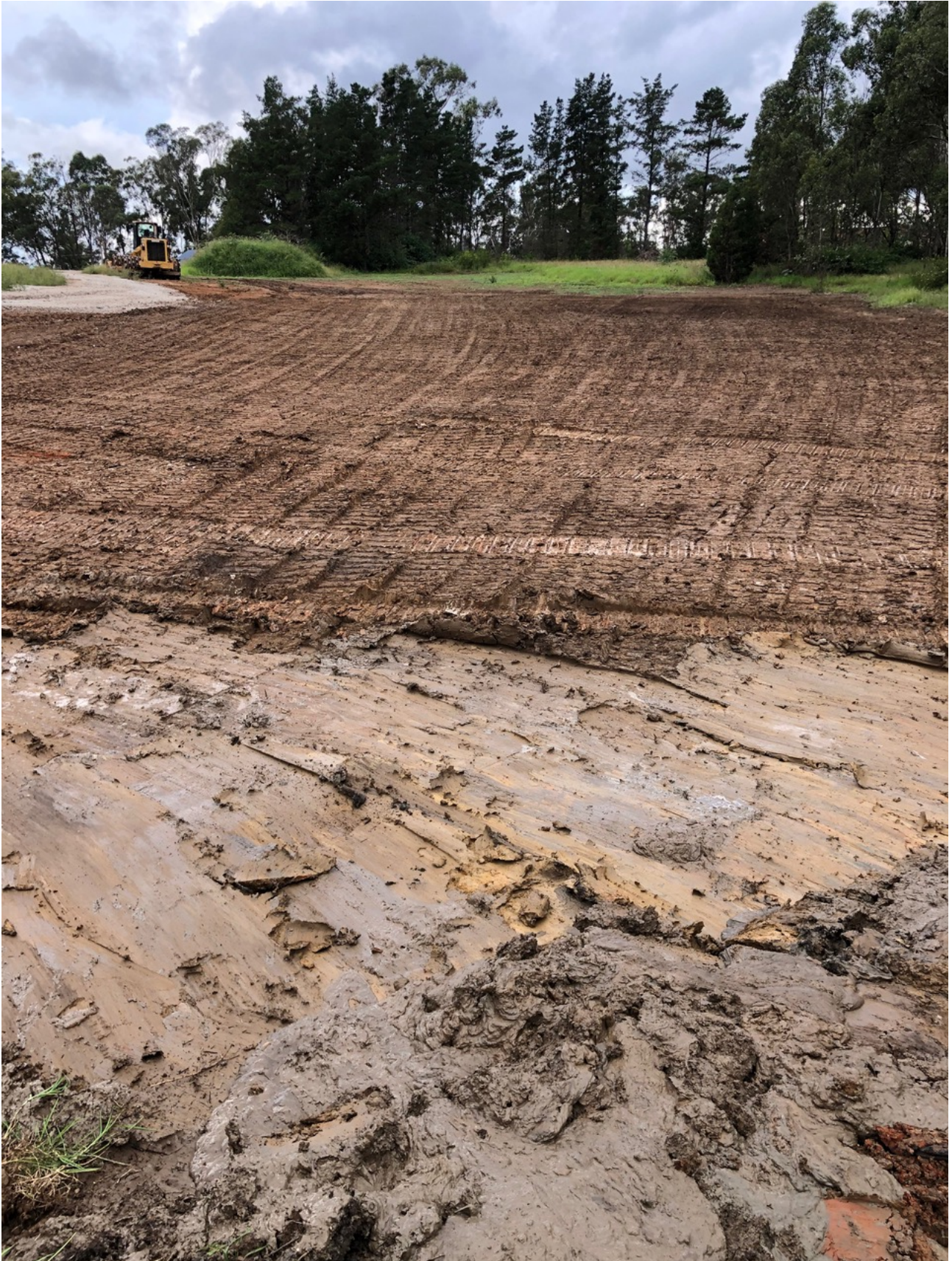
Photograph above: April 2021. View of contaminated areas, 3 (left), 4 (foreground) and 5 (background) following removal of contaminated material to landfill, and following filling and levelling with clean fill.
