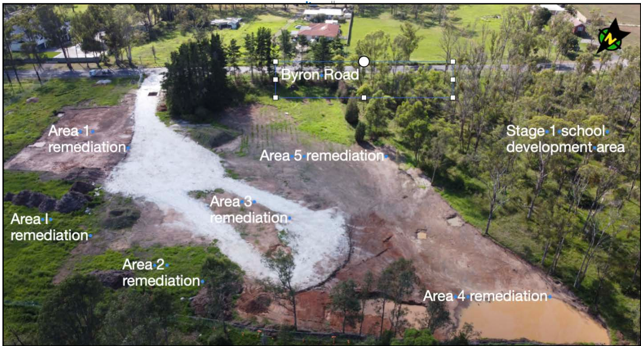
Photograph above: The extent of cleared areas subject to the approved site remediation works is clearly visible from this January 2021 drone photograph of the site, viewed from the west. Byron Road is in the background. (approx. North point shown)
