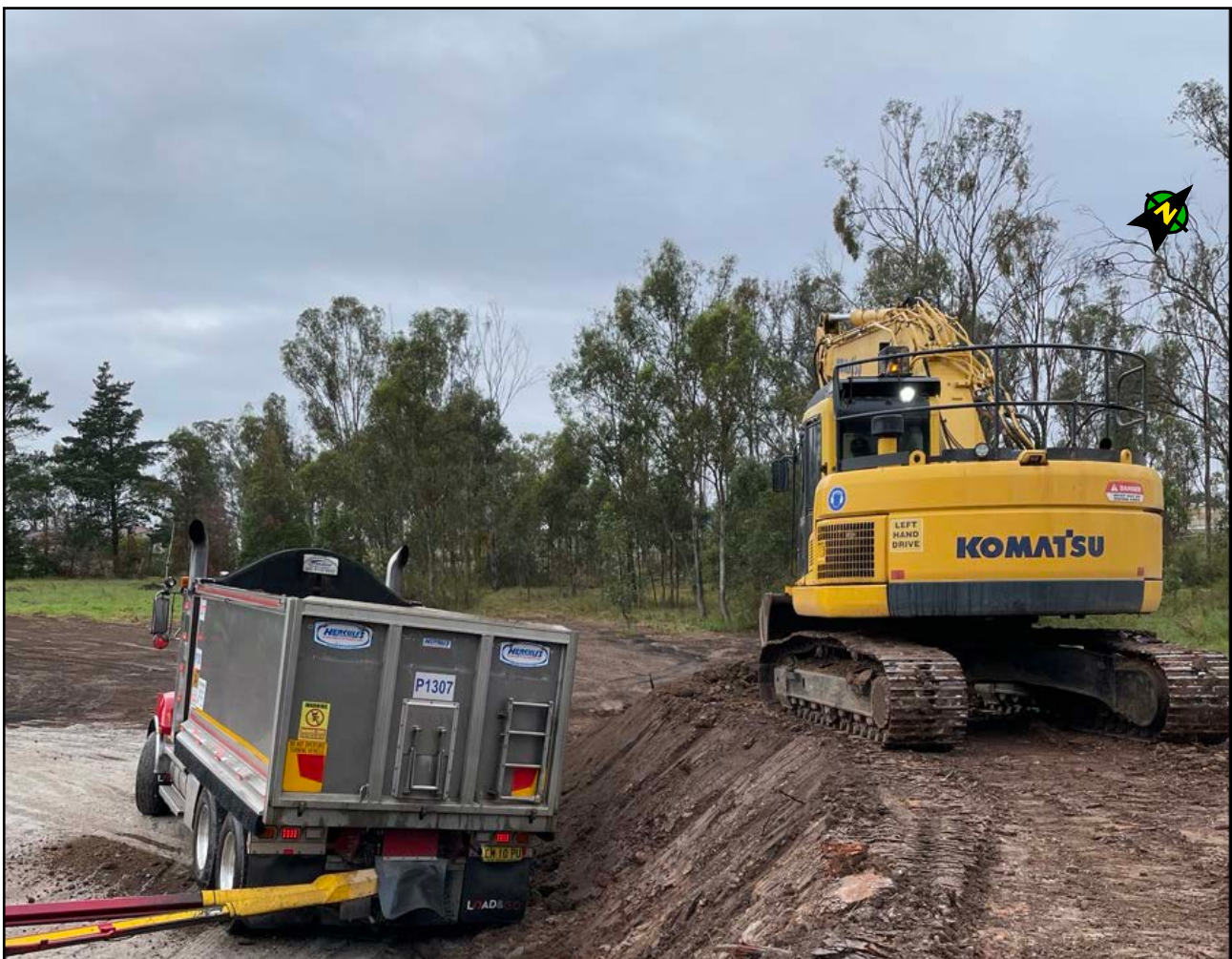
Photograph: Site remediation works underway December 2020
