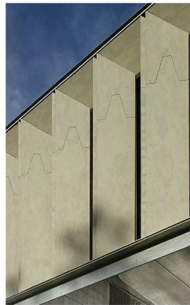
C. CFC CLADDING
