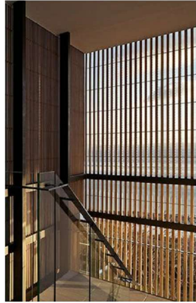
A: ALUMINIUM CLADDING TO GLAZED WINDOWS
