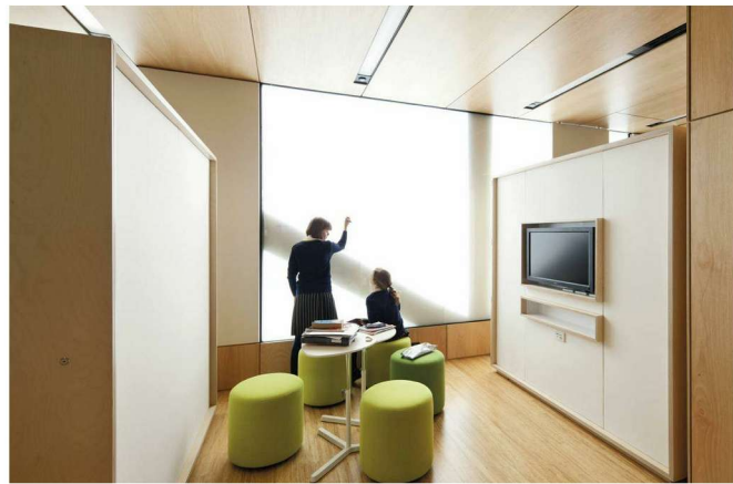
B: MULTI CELL POLYCARBONATE PANELS
