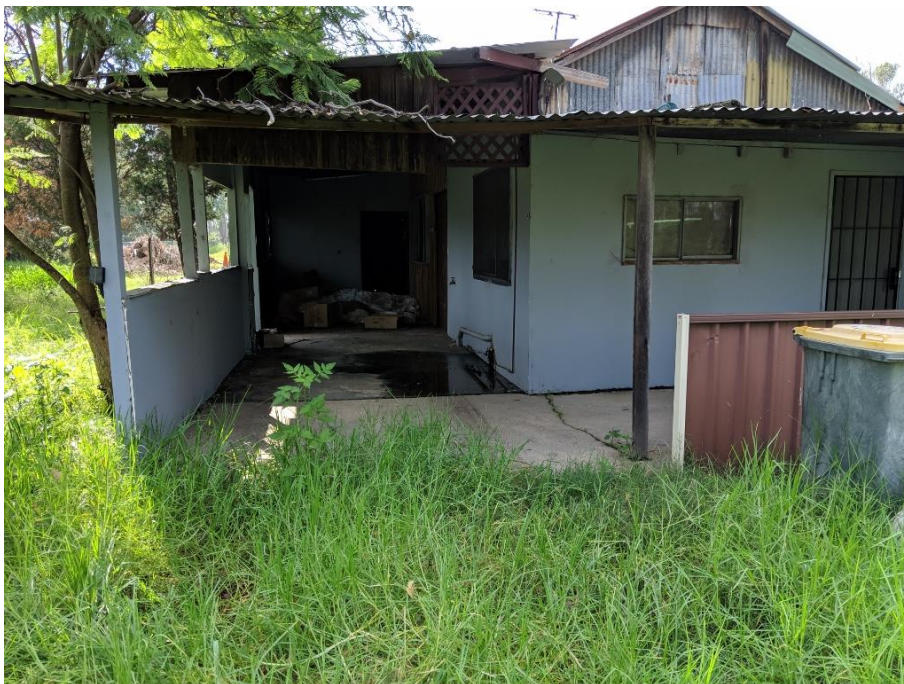
Photo No 8 – Metal, timber and fibro shed (Site Feature E)
