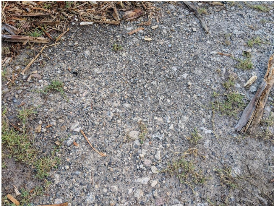
Photo No 3 – Gravel driveway (Site Feature D) with traces of building debris (eg concrete, bricks and asphalt)
