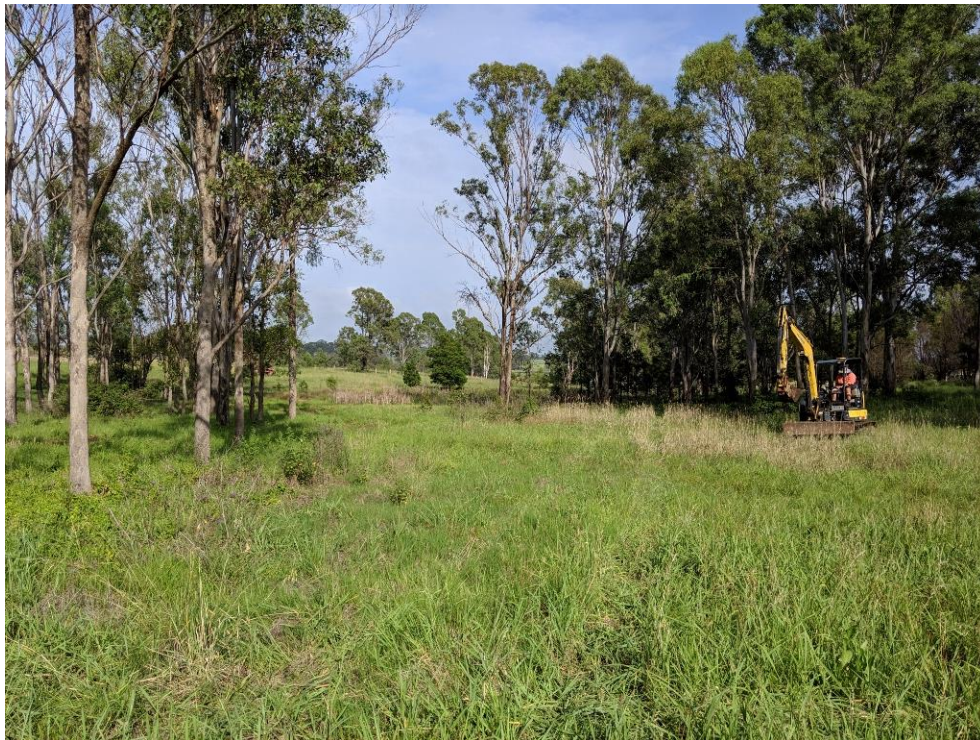
Photo No 6 – Central western portion of the site facing north-west to the backfilled depression area (Site Feature G).
