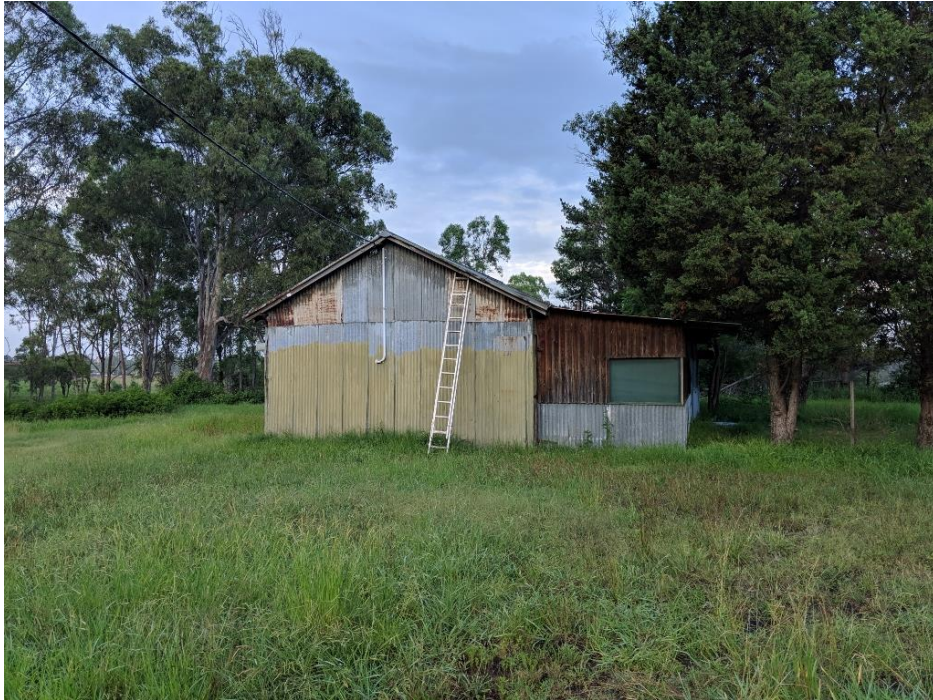
Photo No 7 – Metal, timber and fibro shed (Site Feature E) facing east
