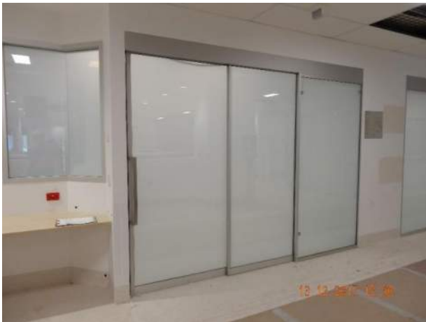
Figure 36 – Examples of compliant sliding door assemblies
