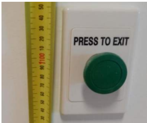
Figure 43 – Installation height setout
