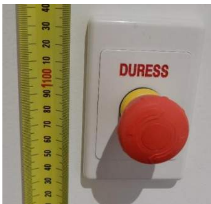
Figure 45 – Installation height setout
