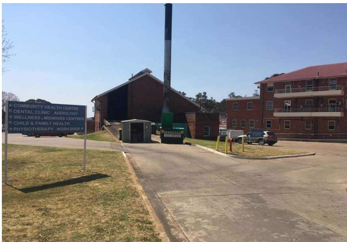
Photo 6 - View of Boiler House looking north
