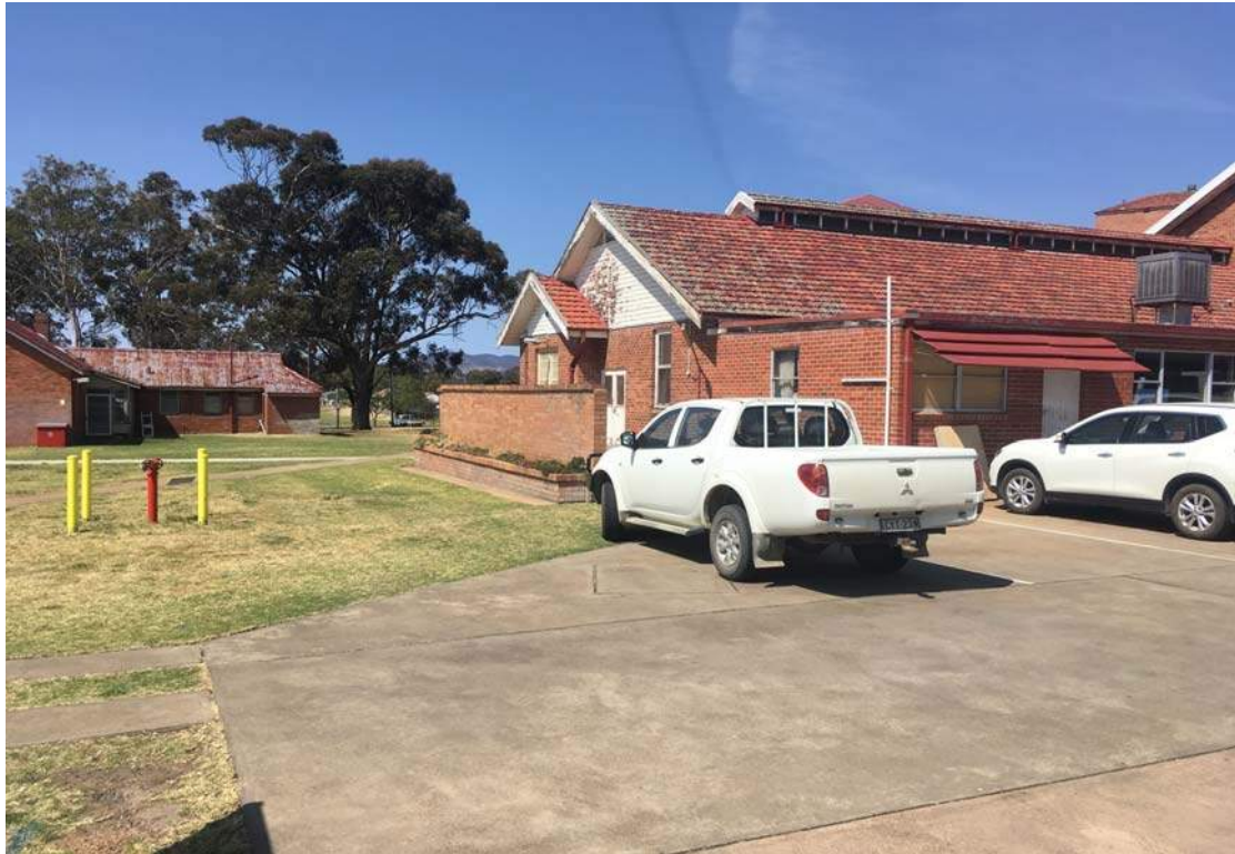
Photo 9 - Northern part of Boiler House looking east
