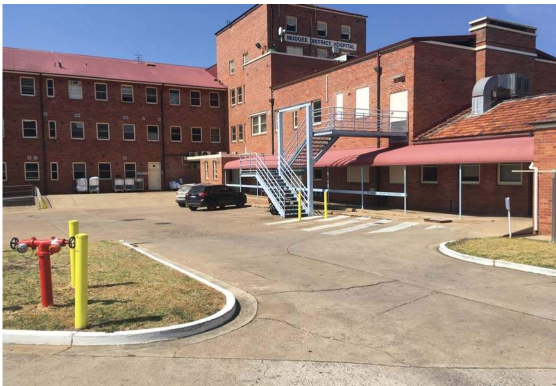
Photo 10 - North-western area of Main Building looking east
