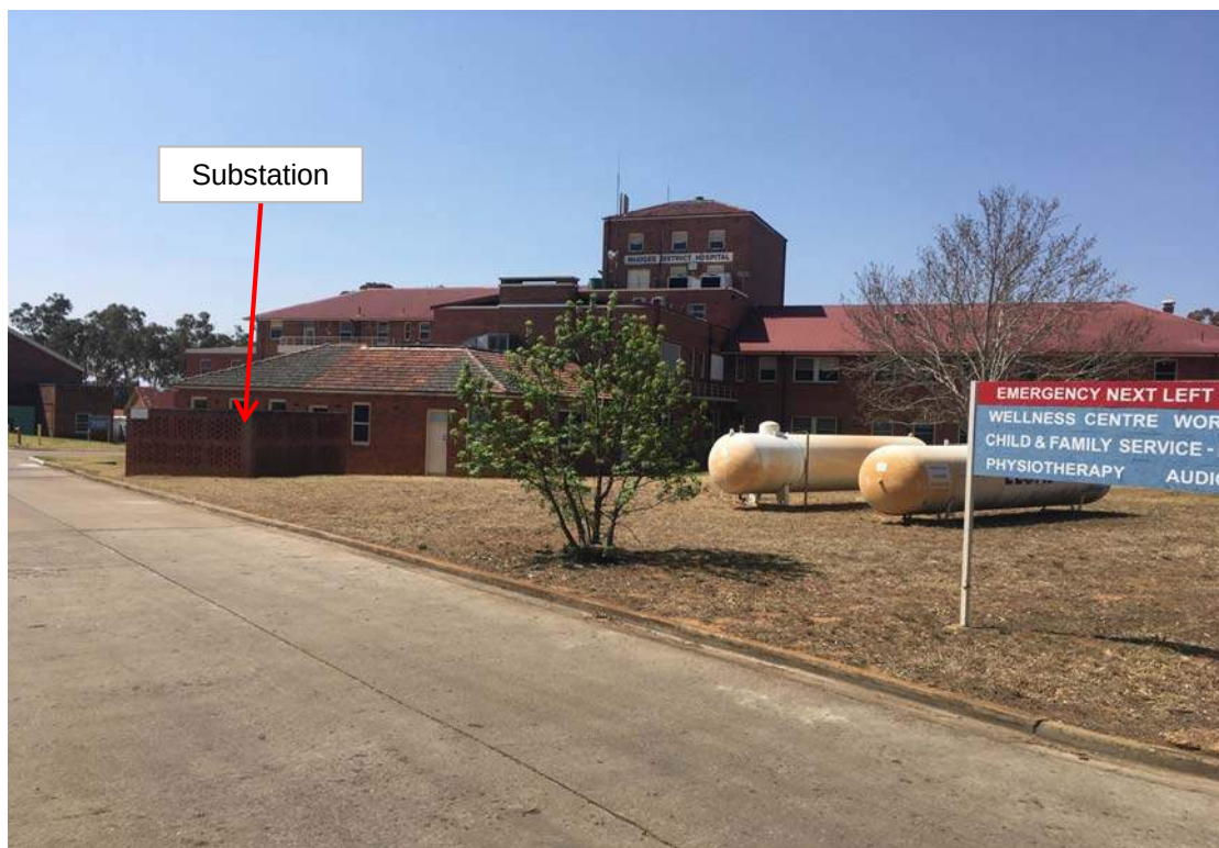
Photo 11 - Gas tanks and electricity substation to south-west of Main Building
