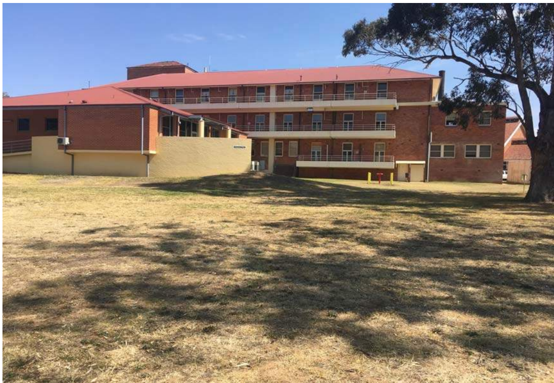
Photo 14 - Main Building from central eastern boundary looking west
