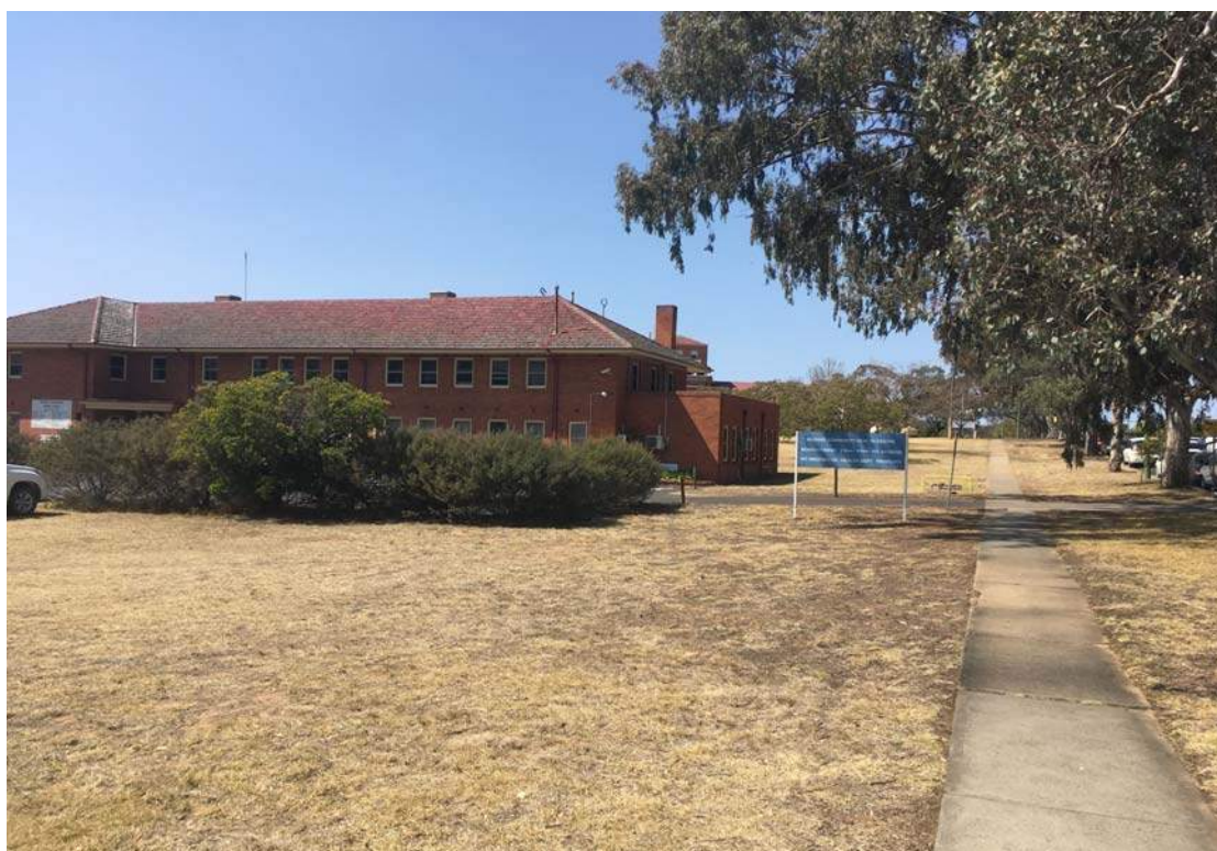
Photo 2 - South-western corner looking east
