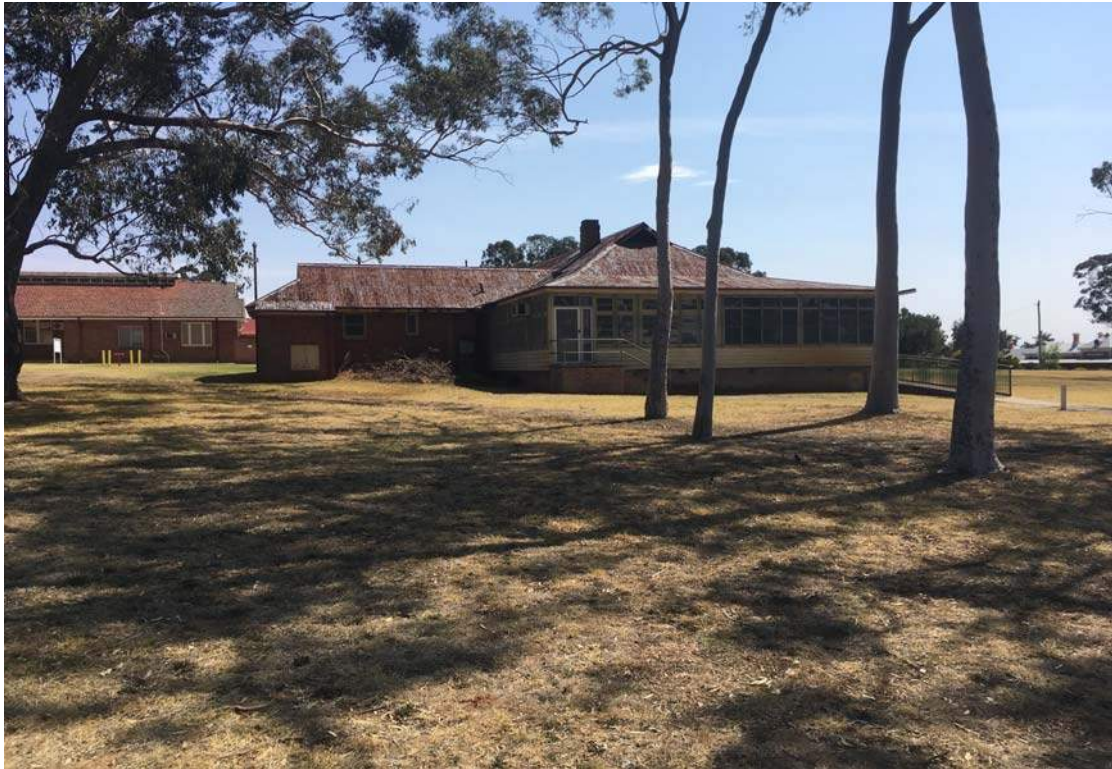
Photo 15 - Vacant building north of Main Building looking west
