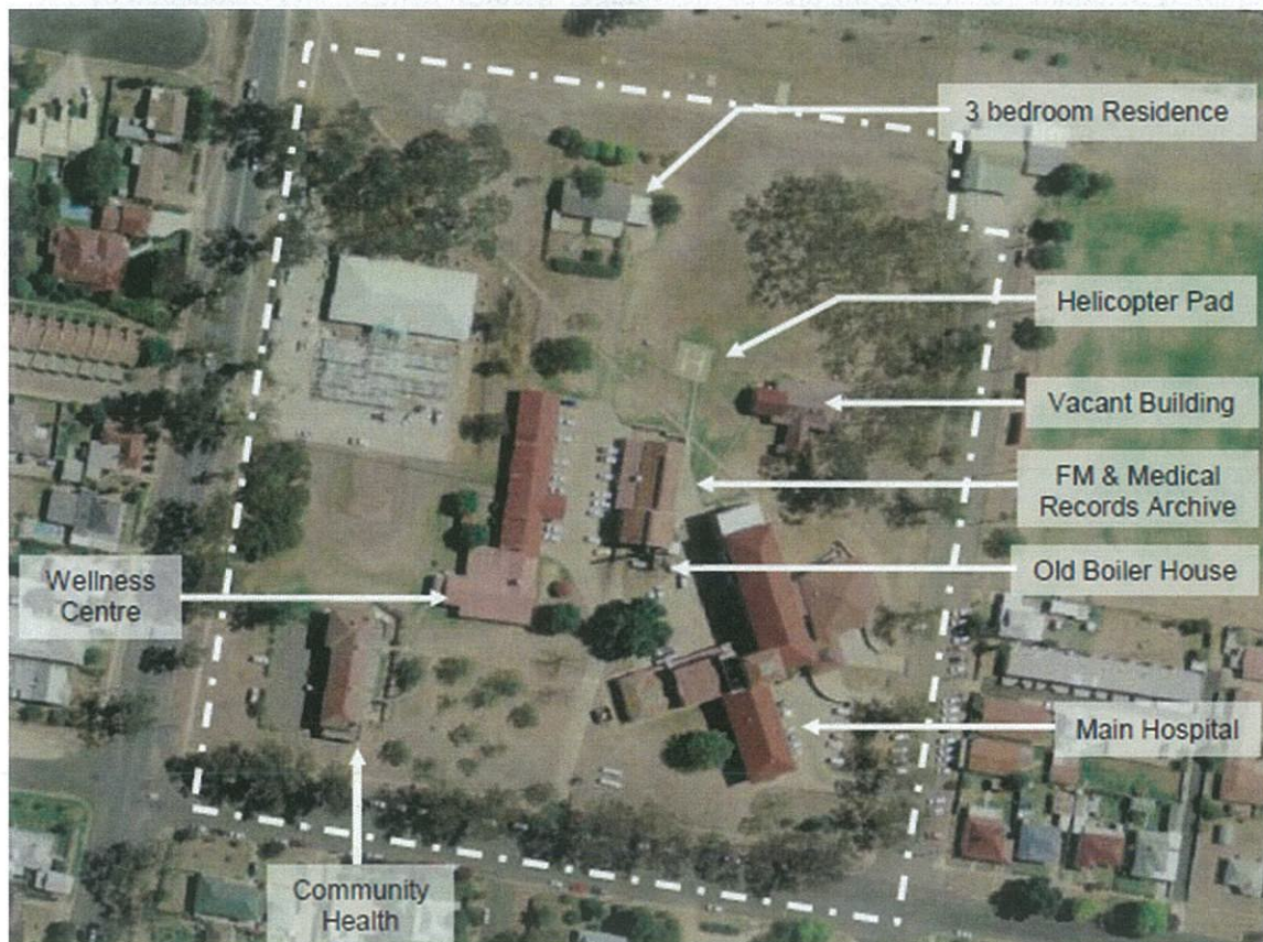
Figure 5: Mudgee Hospital and Health Service existing built form.
