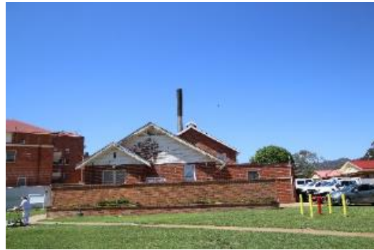
Plate 14 Old Boiler Room Building north face
