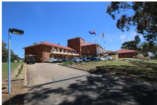
Plate 31 Main Building entrance on Lewis St) (western side)
