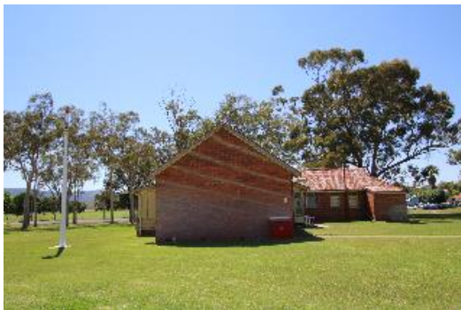
Plate 11 Vacant building southern wall
