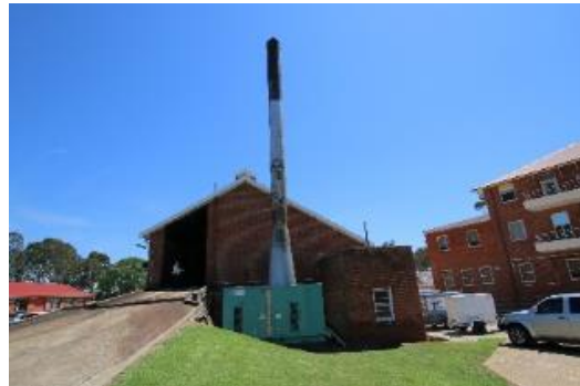
Plate 16 Old Boiler Room Building south face
