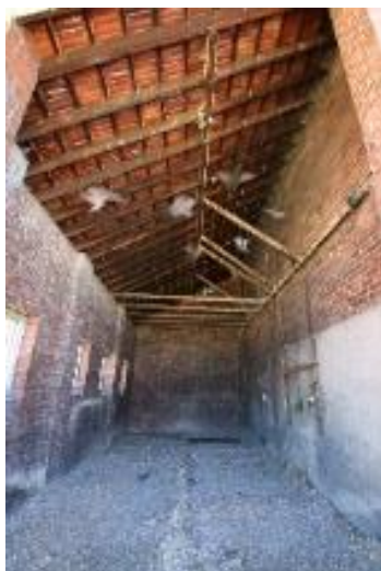
Plate 19 Coal store on southern end of Old Boiler Room
