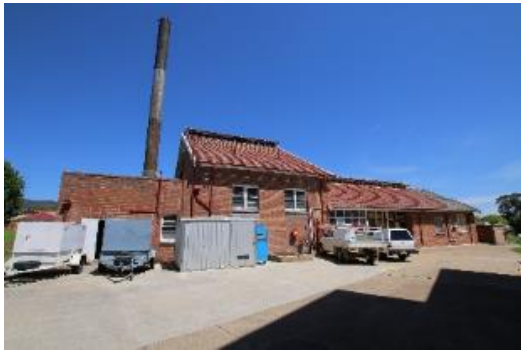
Plate 13 Old Boiler Room Building east face
