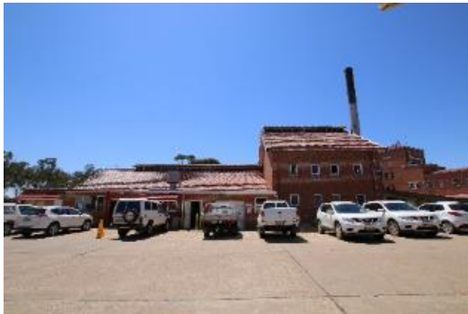
Plate 15 Old Boiler Room Building west face
