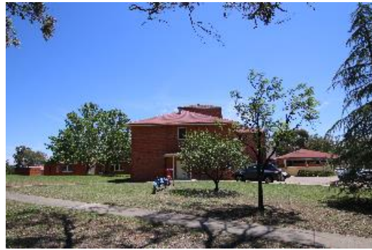
Plate 30 Main Building southern wall
