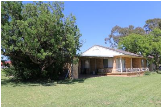
Plate 5 Residence eastern side
