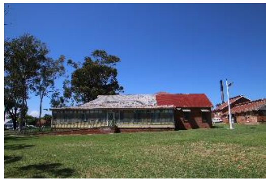
Plate 10 Vacant building northern wall
