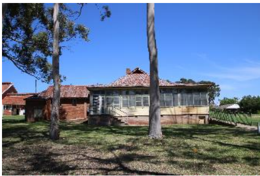
Plate 9 Vacant building eastern wall
