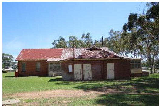
Plate 12 Vacant building western wall
