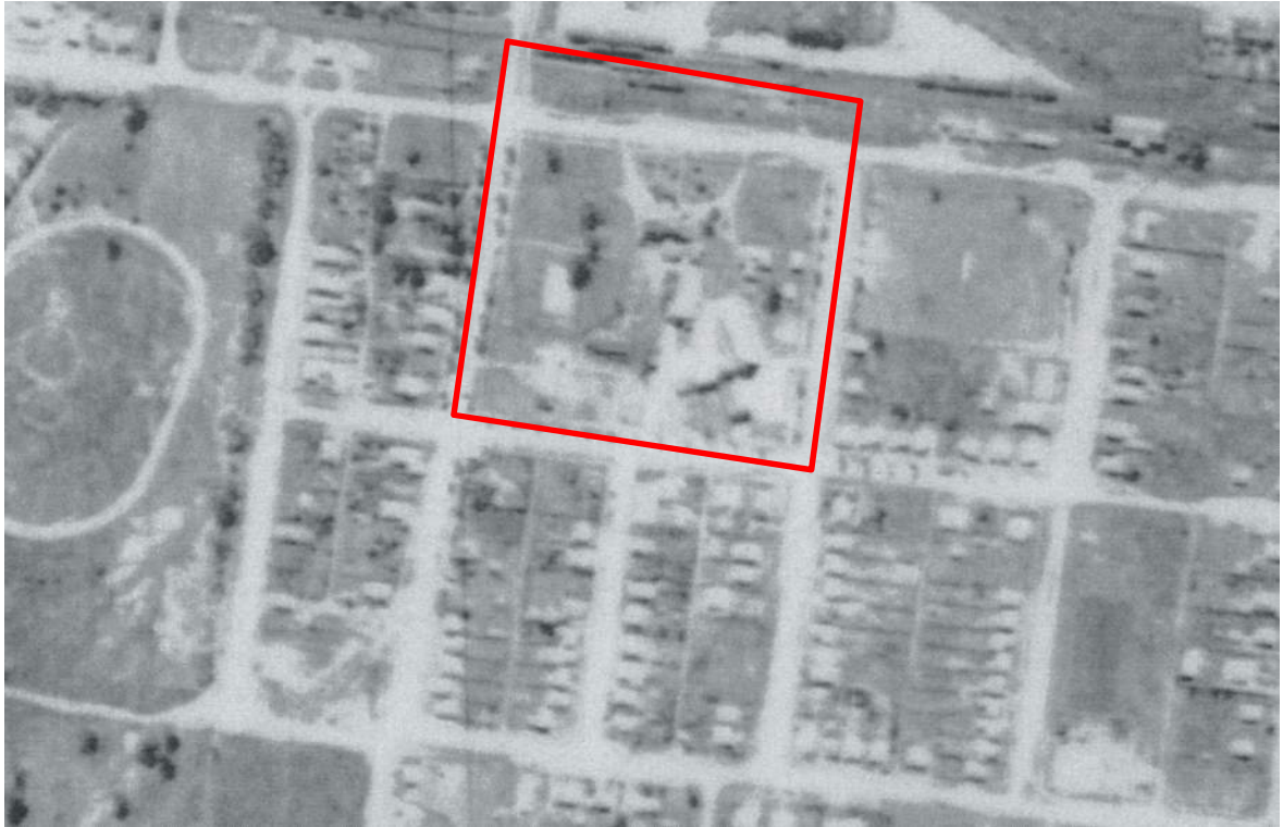
Aerial photograph from 1956
